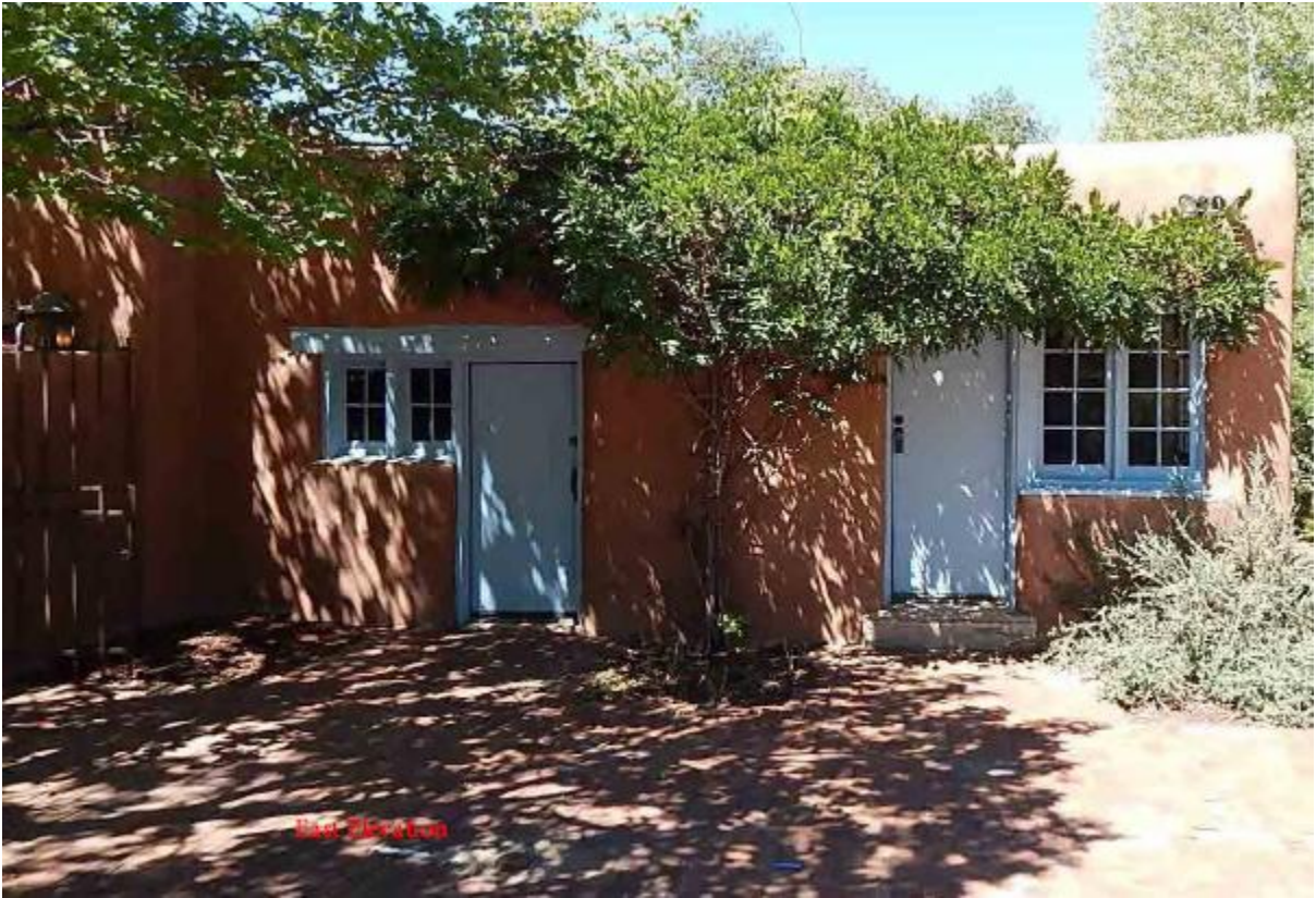
Figure 3. East Facade I.
