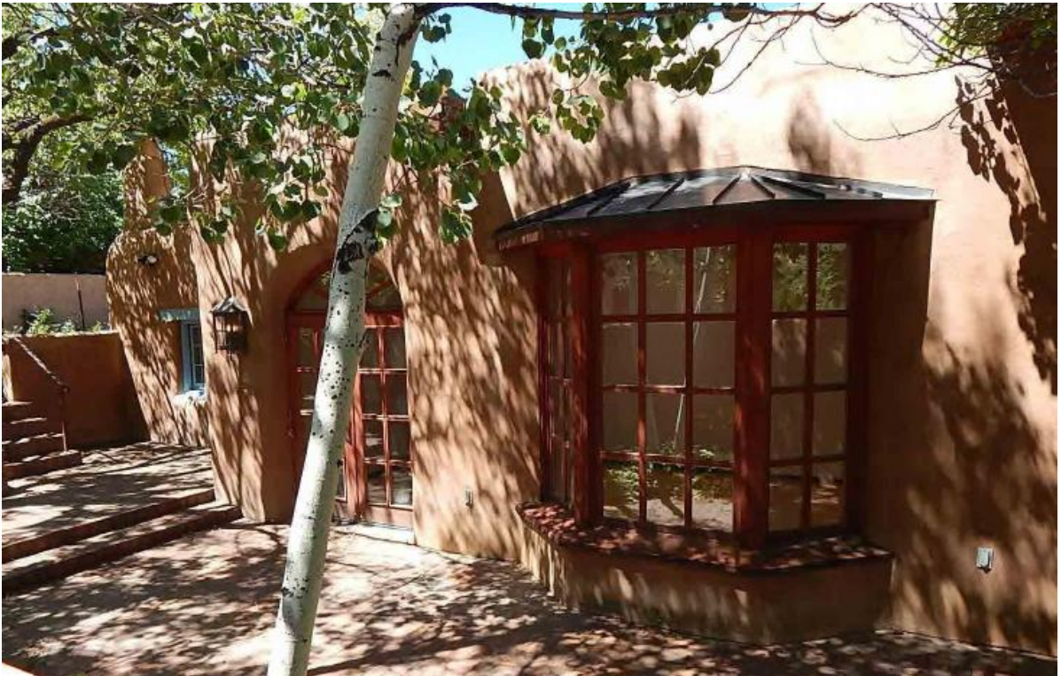
Figure 5. East Facade III.
