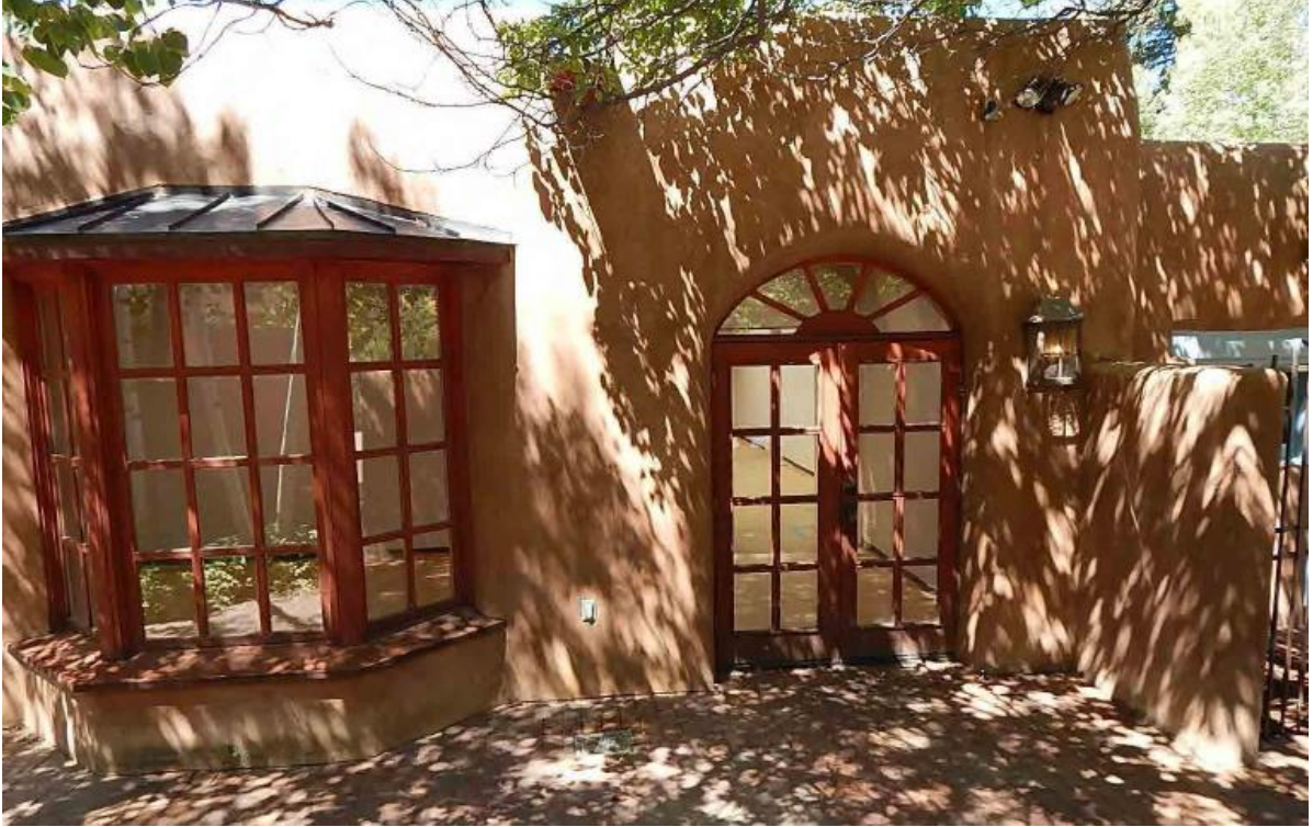
Figure 4. East Facade II.
