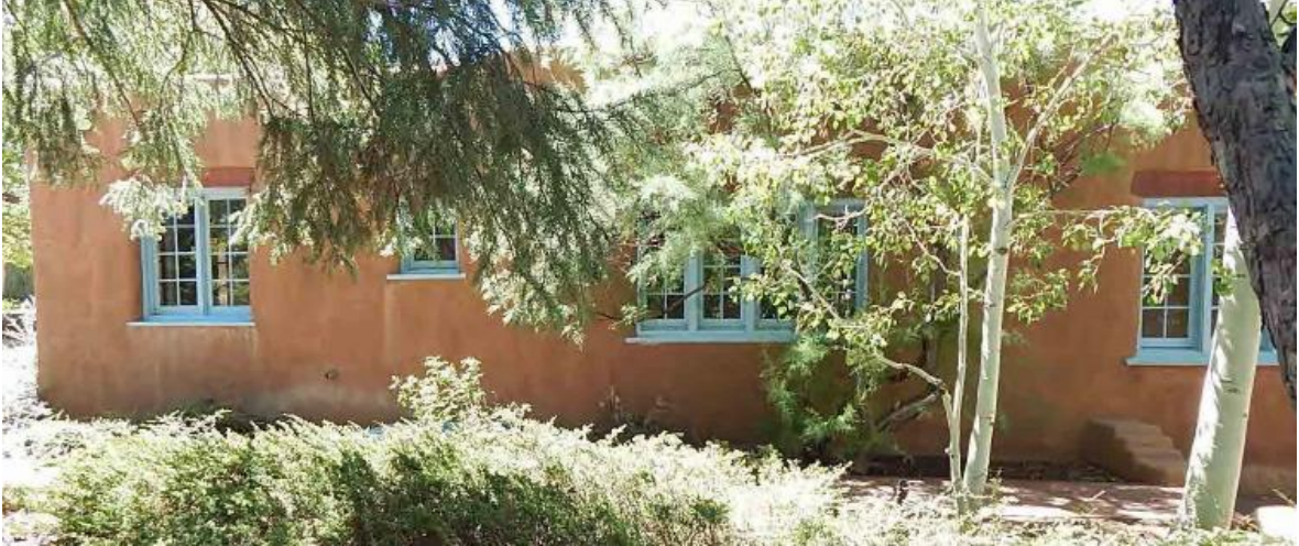
Figure 2. North Facade II.
