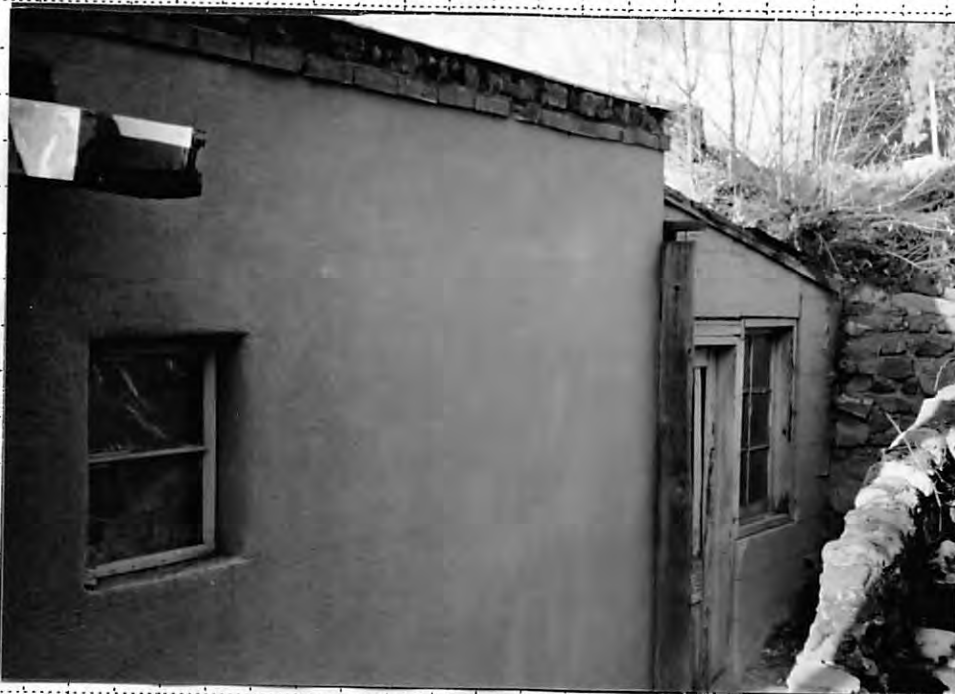
Above: Detail of rear east elevation
