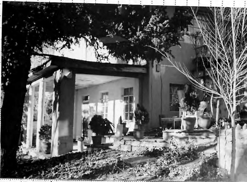
Southeast elevation - porch detail
