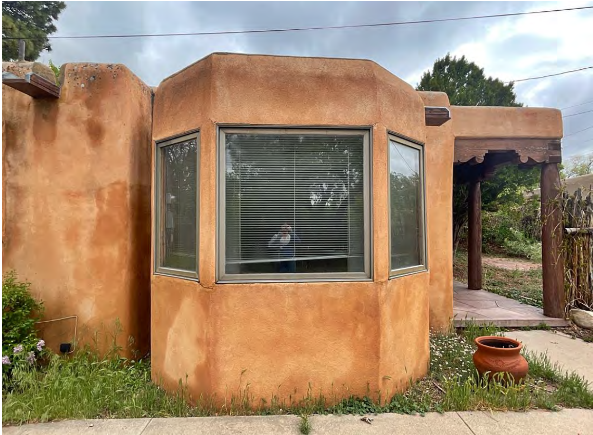
Photo 10: Bay projection. Camera facing east.
