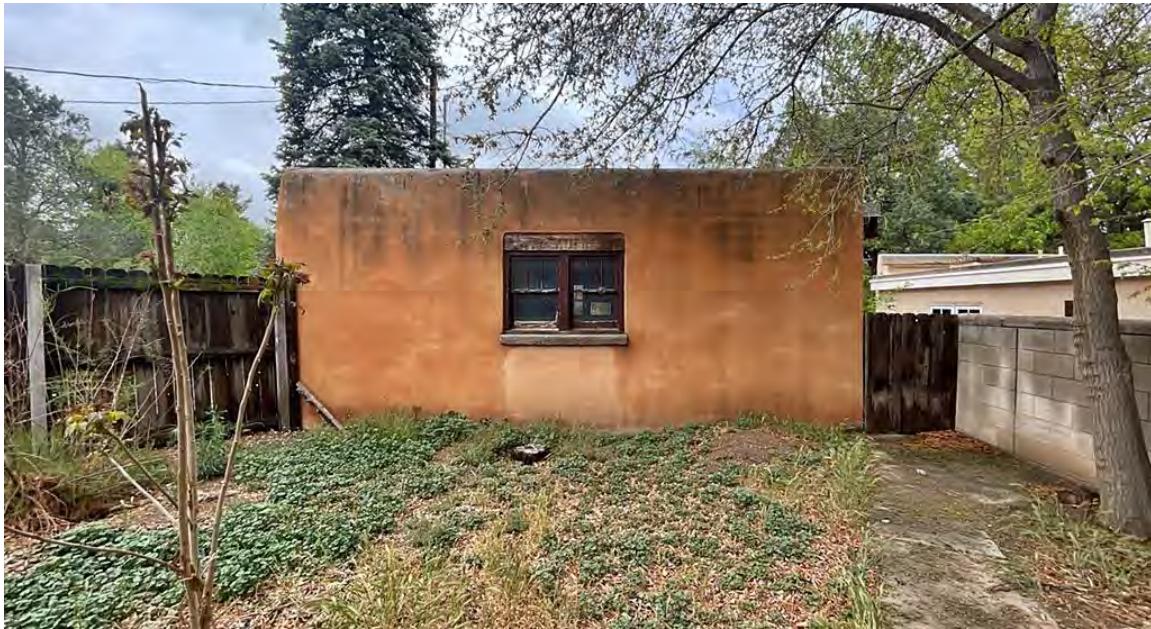
Photo 22: Garage. East elevation. Camera facing west.
