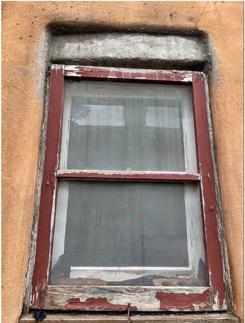
Photo 16: East elevation. Window at bedroom. Camera facing up.
