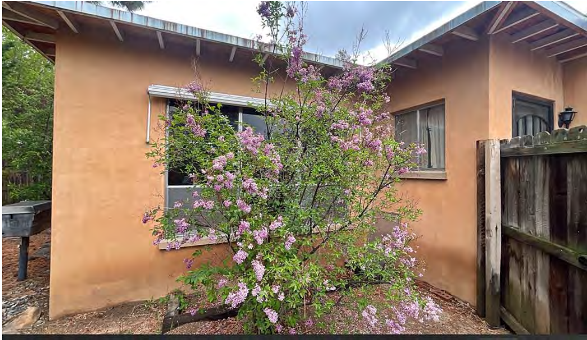
Photo 12: West elevation. Addition. Camera facing southeast.
