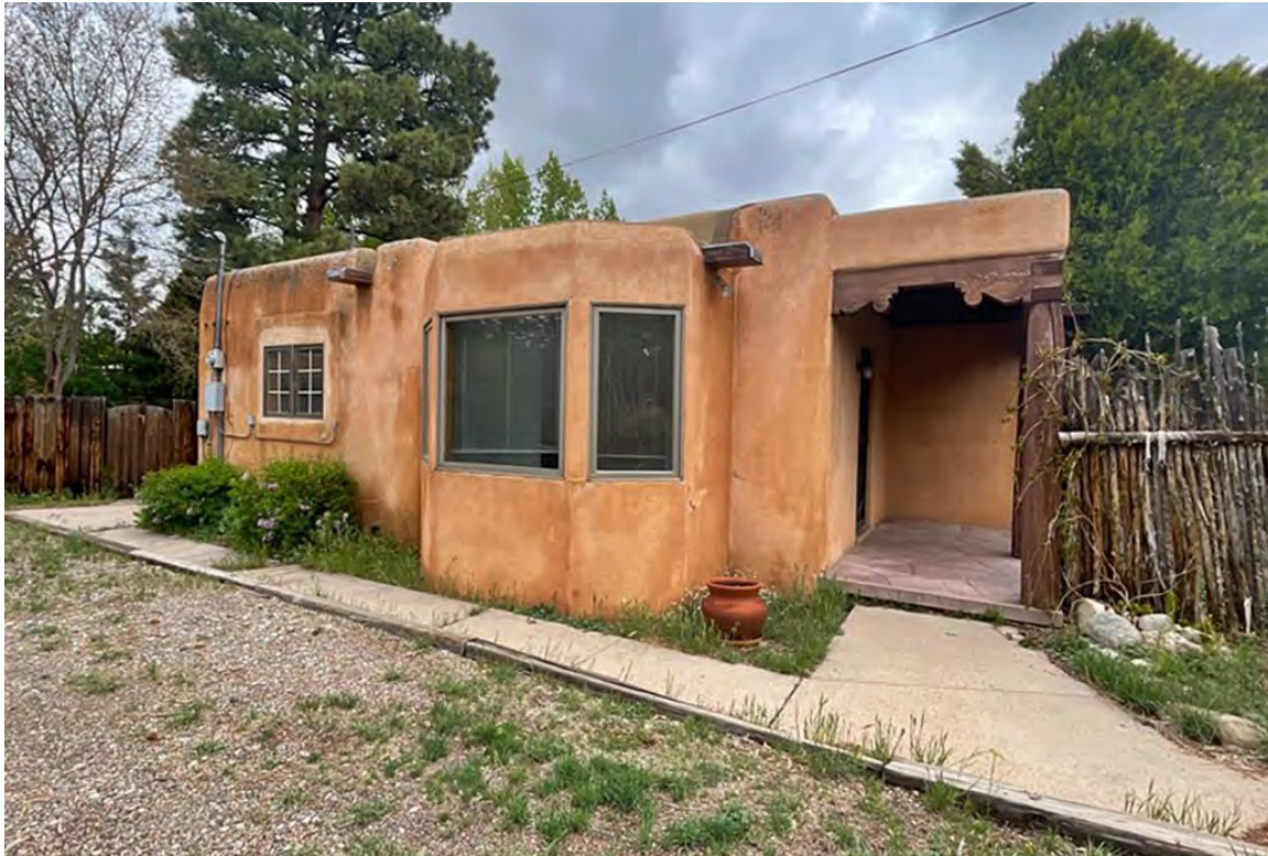
Photo 9: West elevation oblique. Camera facing northeast.
