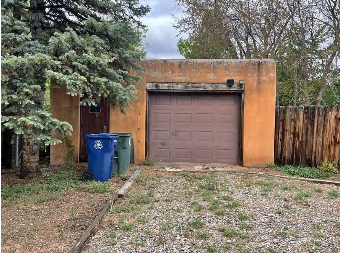
Photo 21: Garage. South elevation. Camera facing north.
