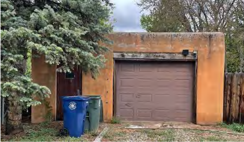
Figure 4: South Elevation of Accessory Structure
