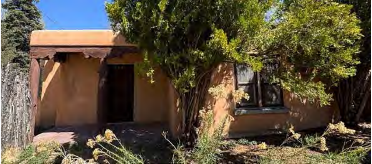
Figure 2: South Elevation of Residential Structure
