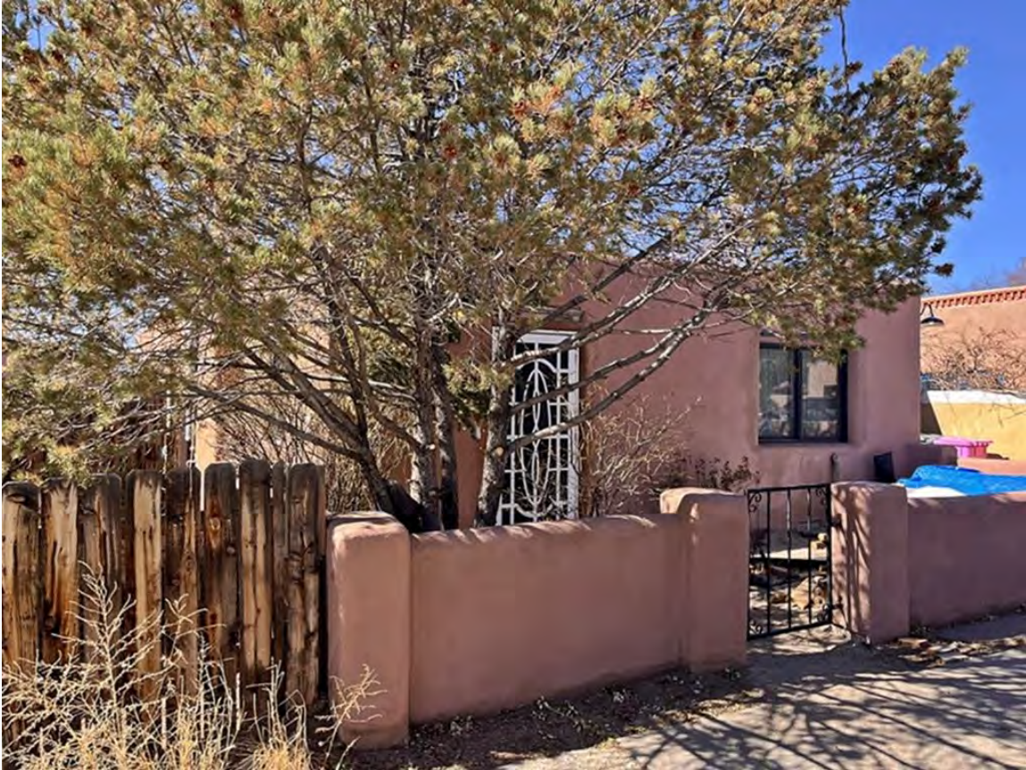
Photo 15: Front yard wall. Camera facing northeast. John W. Murphey, February 27, 2025.
