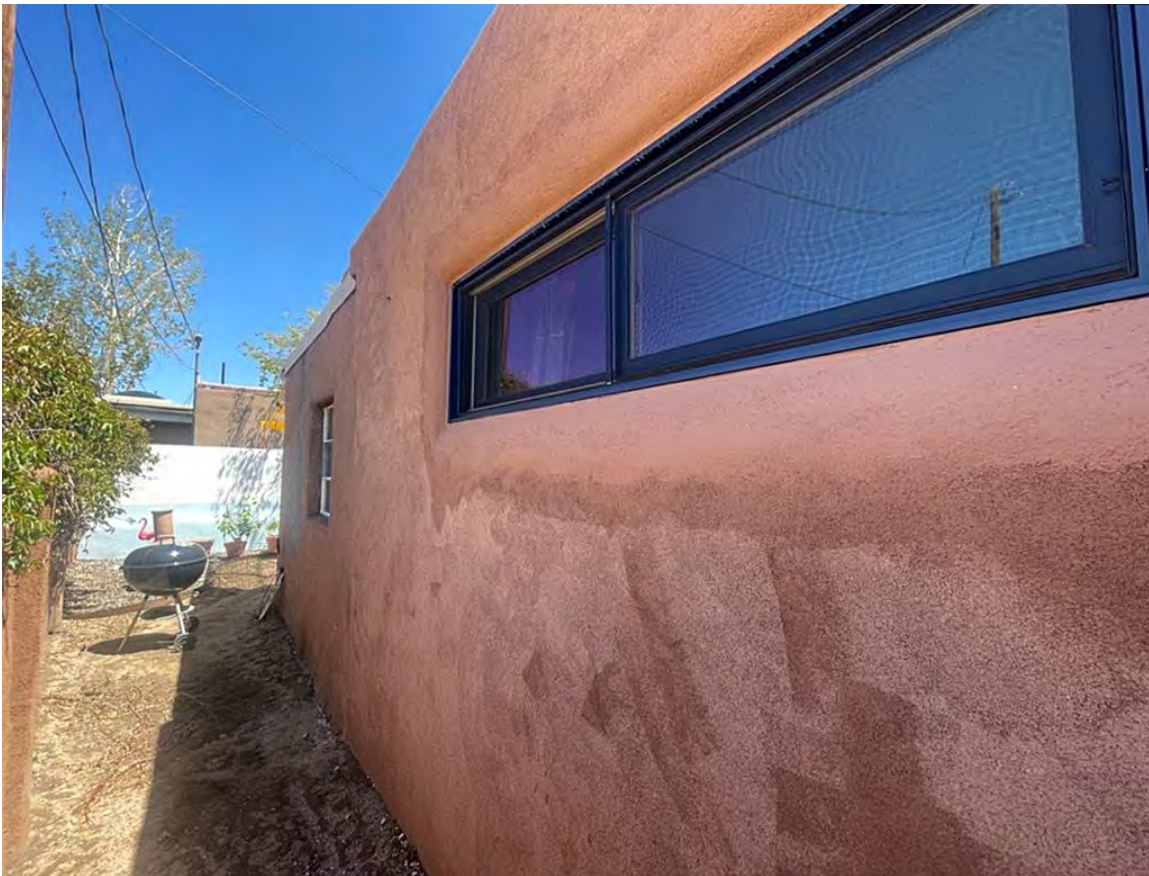
Photo 9: West elevation. Recent window at addition. Camera facing northwest.
