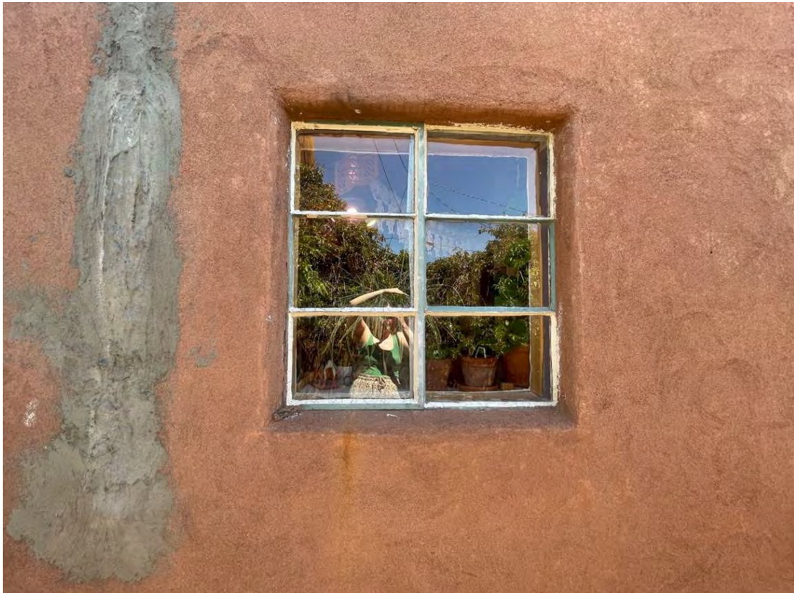
Photo 10: West elevation. Steel window at enclosed porch. Camera facing east.
