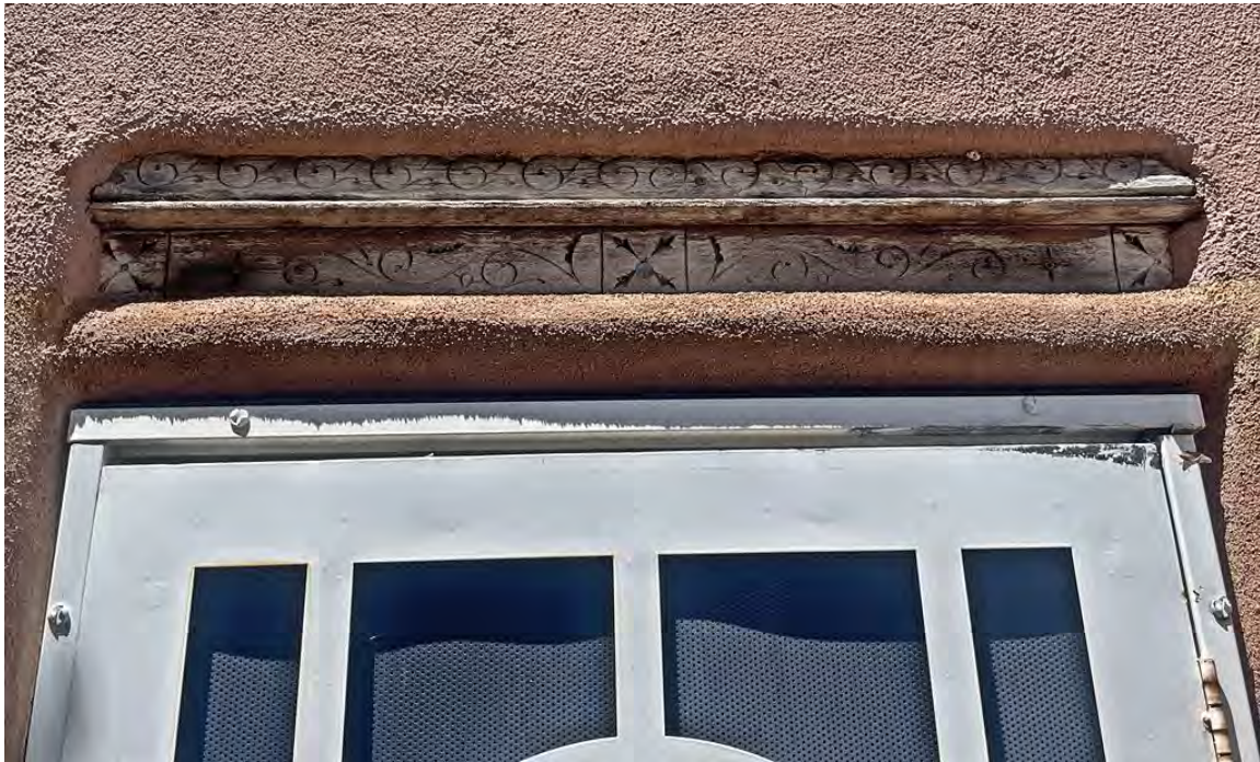
Photo 4: East elevation. Trim above front door. Camera facing up.
