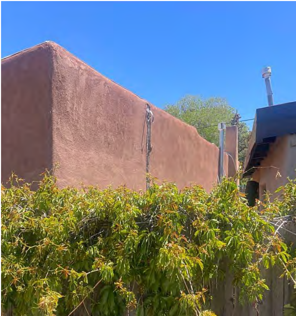
Photo 7: South elevation. West end representing addition. Camera facing northeast.
