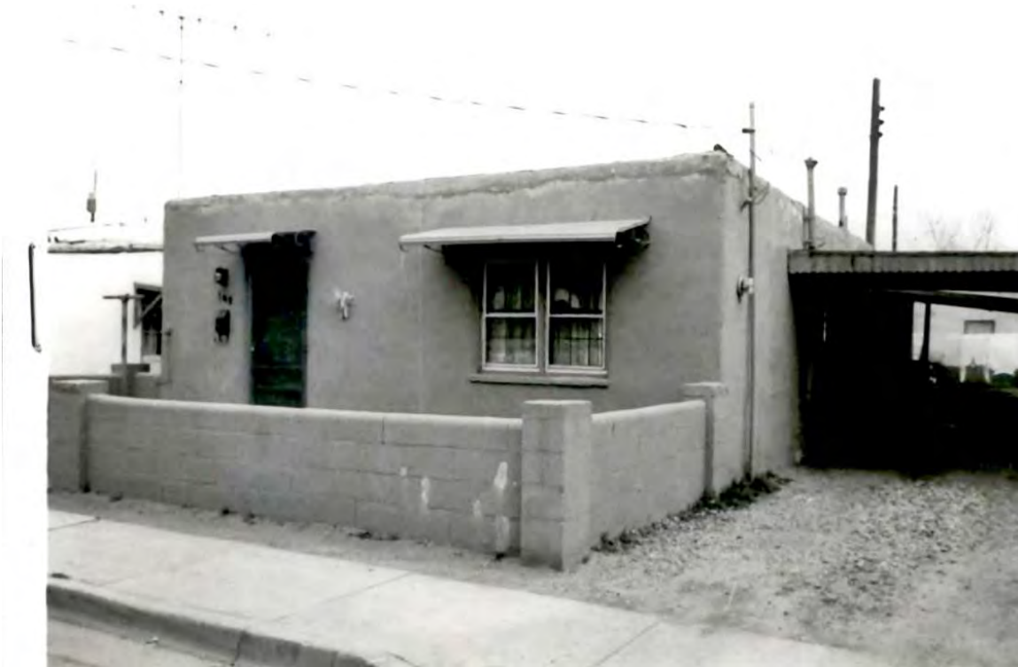
Figure 8: August 1985 Historic Building Inventory photograph. Harry Weiss, photographer. Courtesy of NMCRIS. Note paired 6/6 windows, unstuccoed yard wall, and open carport and porch.
