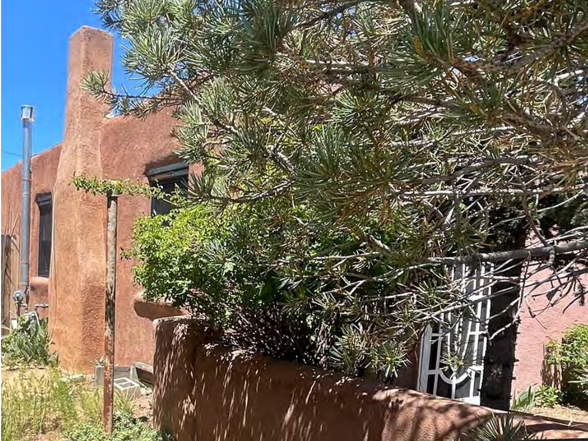
Photo 6: South elevation. East end representing original house. Camera facing northeast
