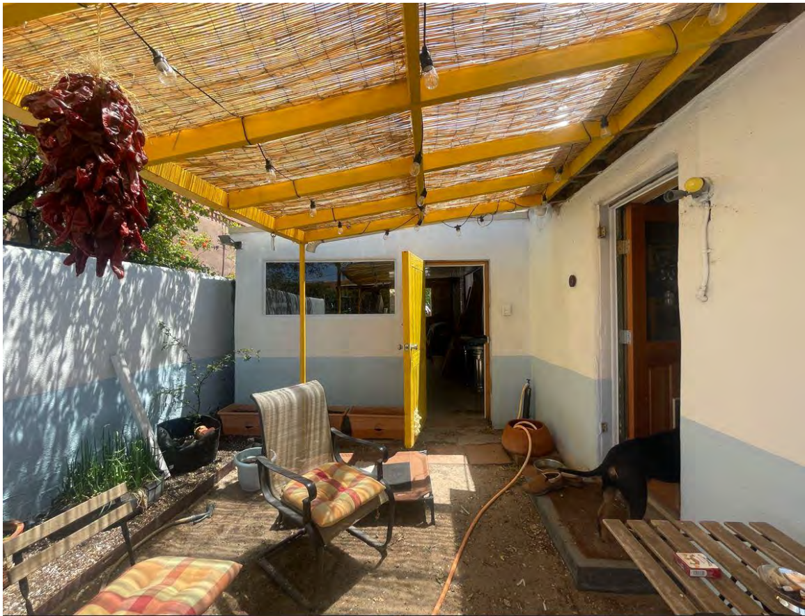
Photo 13: West elevation of enclosed carport. Camera facing east.
