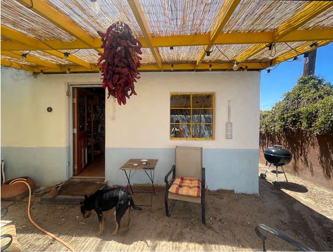
Photo 14: North elevation of enclosed porch. Camera facing south.
