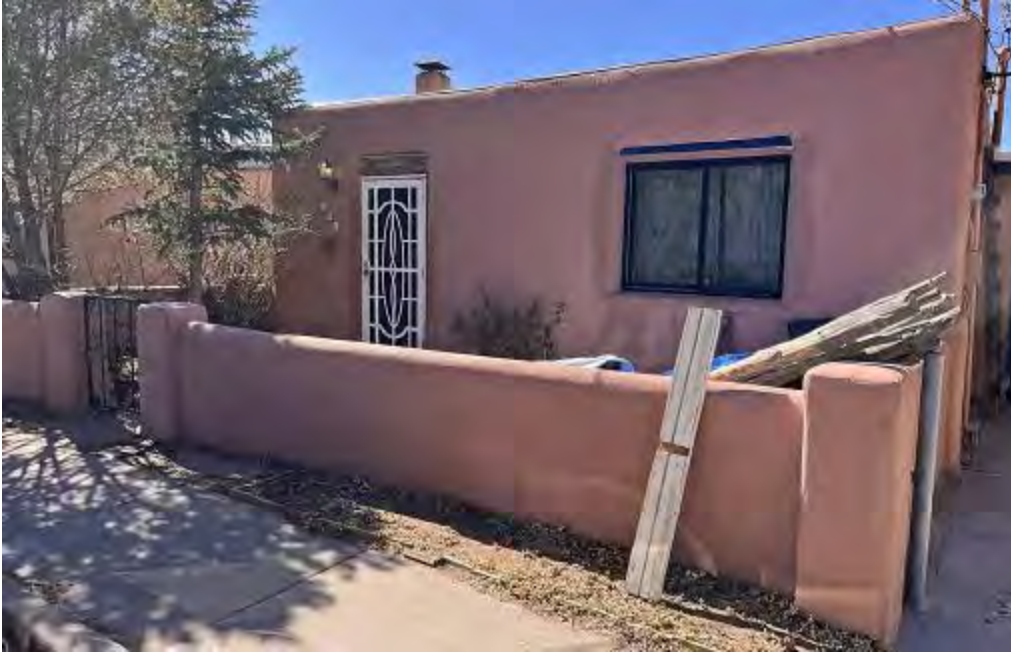
Figure 2: East elevation of Residential Structure with yard wall.
