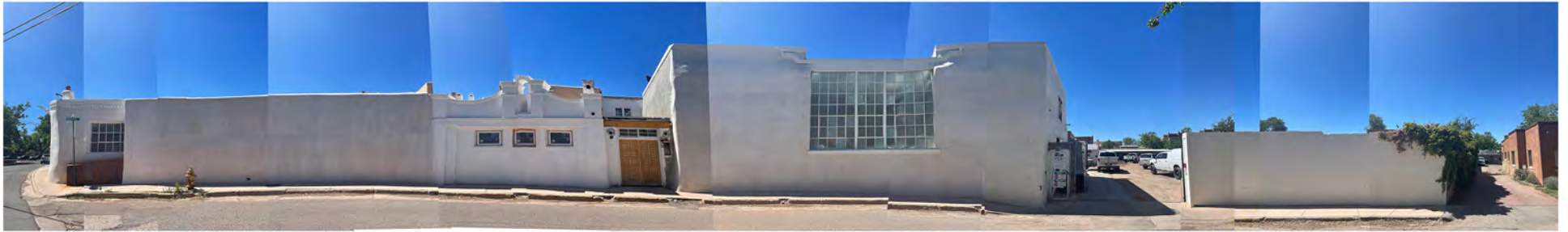
206 McKenzie Street McKenzie Street / North Elevation
