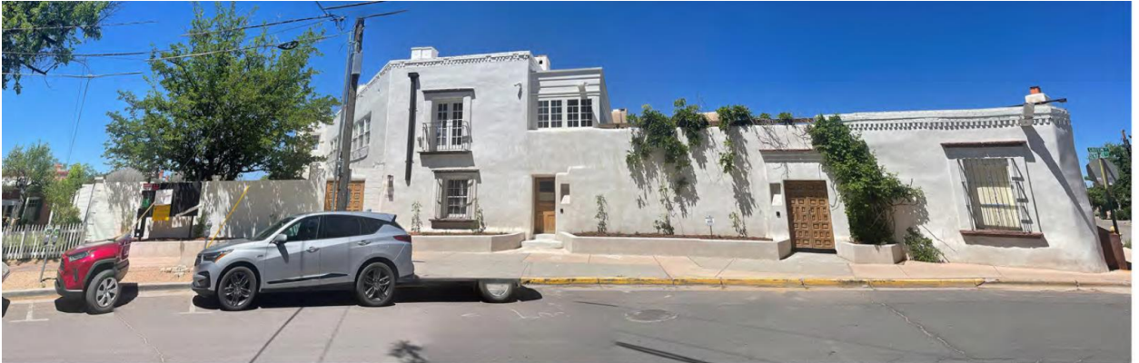
206 McKenzie Street Griffin Street / East Elevation
