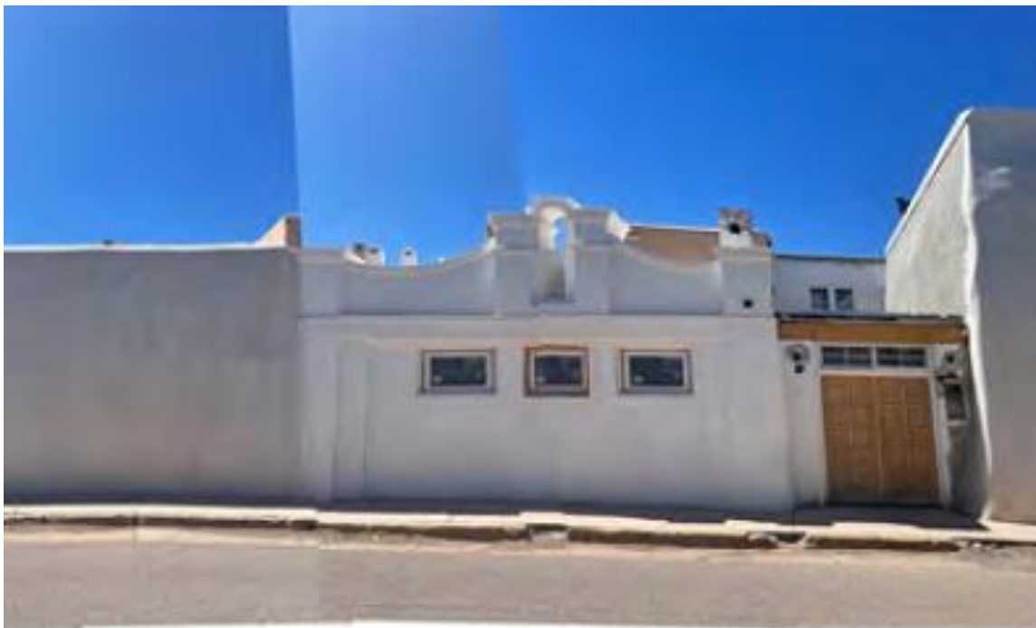
Figure 4. North Primary Facade.
