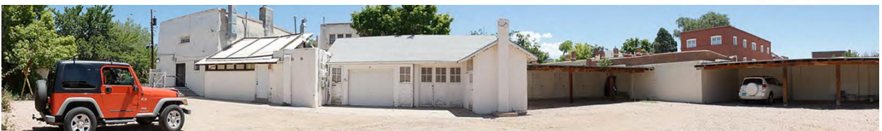
206 McKenzie Street Parking / West Elevation
