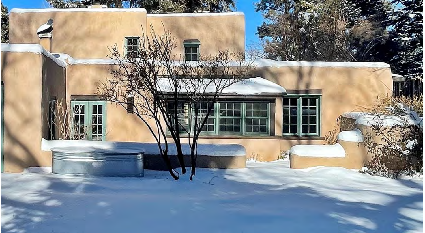
Photo 11: Partial south elevation. Primary bedroom wing (former apartment), left; infilled portal and kitchen extension, center; dining room addition, right; historic two-story core block, background. Camera facing north.
