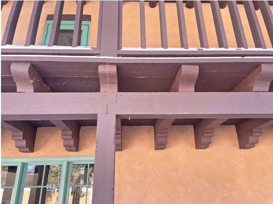
Photo 5: Supporting structure of two-tiered porch. Camera facing up.
