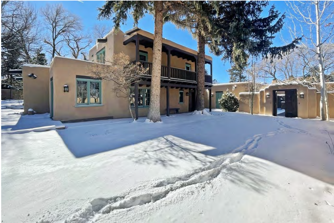
Photo 3: North elevation. Dining room addition, left; historic two-story core block, center; non-historic two-car garage and gate, right.
