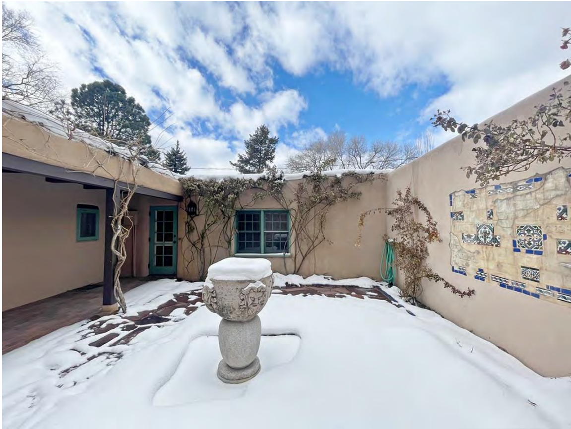
Photo 16: East elevation, former one-car garage. Camera facing west. January 14, 2024.
