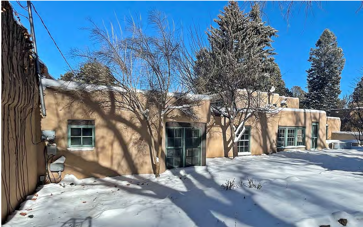
Photo 13: Full South elevation. Non-historic bump-put bathroom addition, left; primary bedroom wing, center; infilled portal and kitchen extension, right; dining room addition, extreme right. Camera facing northeast.
