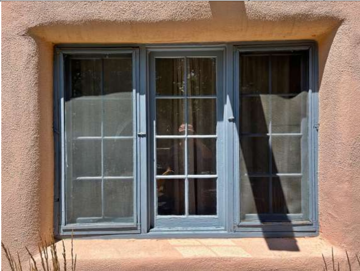
Photo 5: East elevation, assumed core block, casement windows. Camera facing west.
