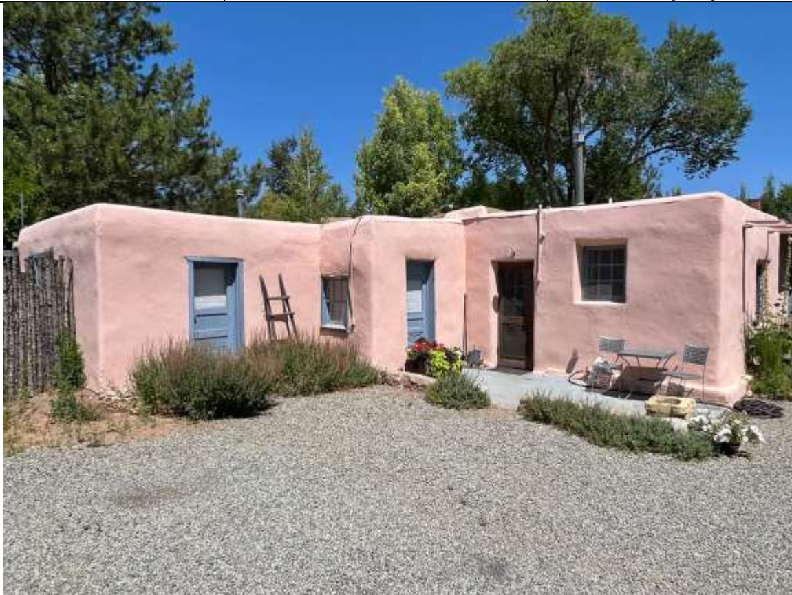
Photo 8: South elevation, assumed additions at left. Camera facing northwest.
