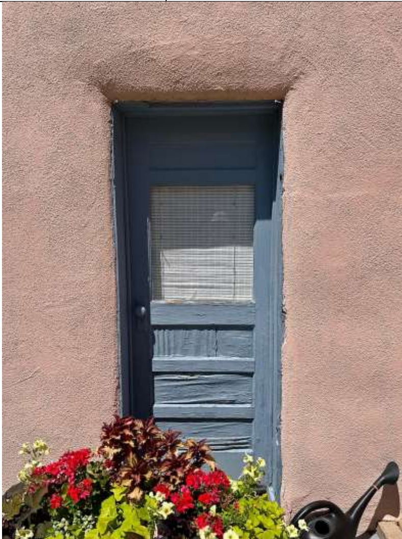
Photo 7: East elevation, assumed addition, door. Camera facing west.
