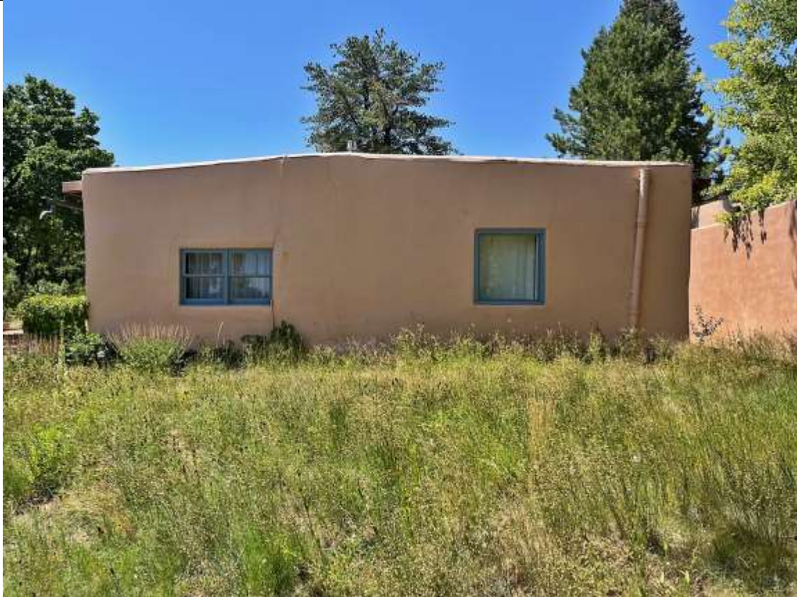
Photo 11: North elevation. Camera facing south.
