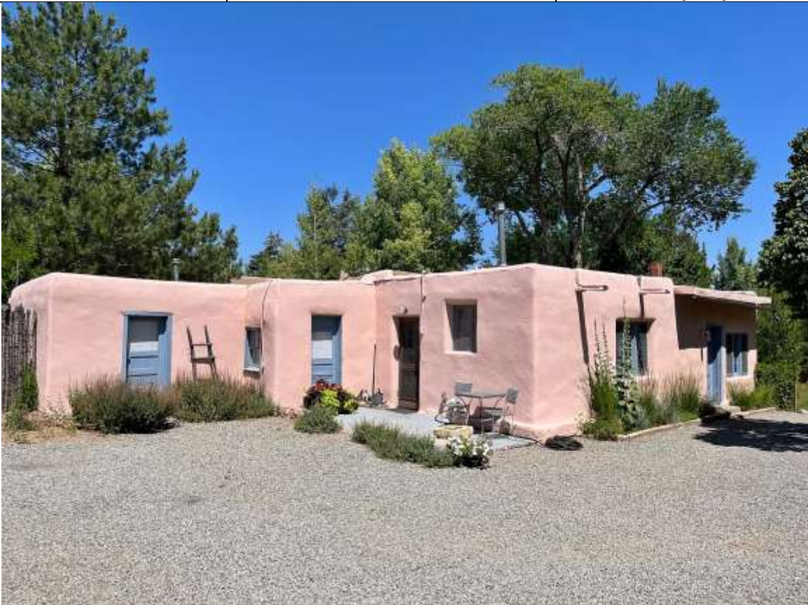
Photo 3: East elevation. Camera facing northwest.
