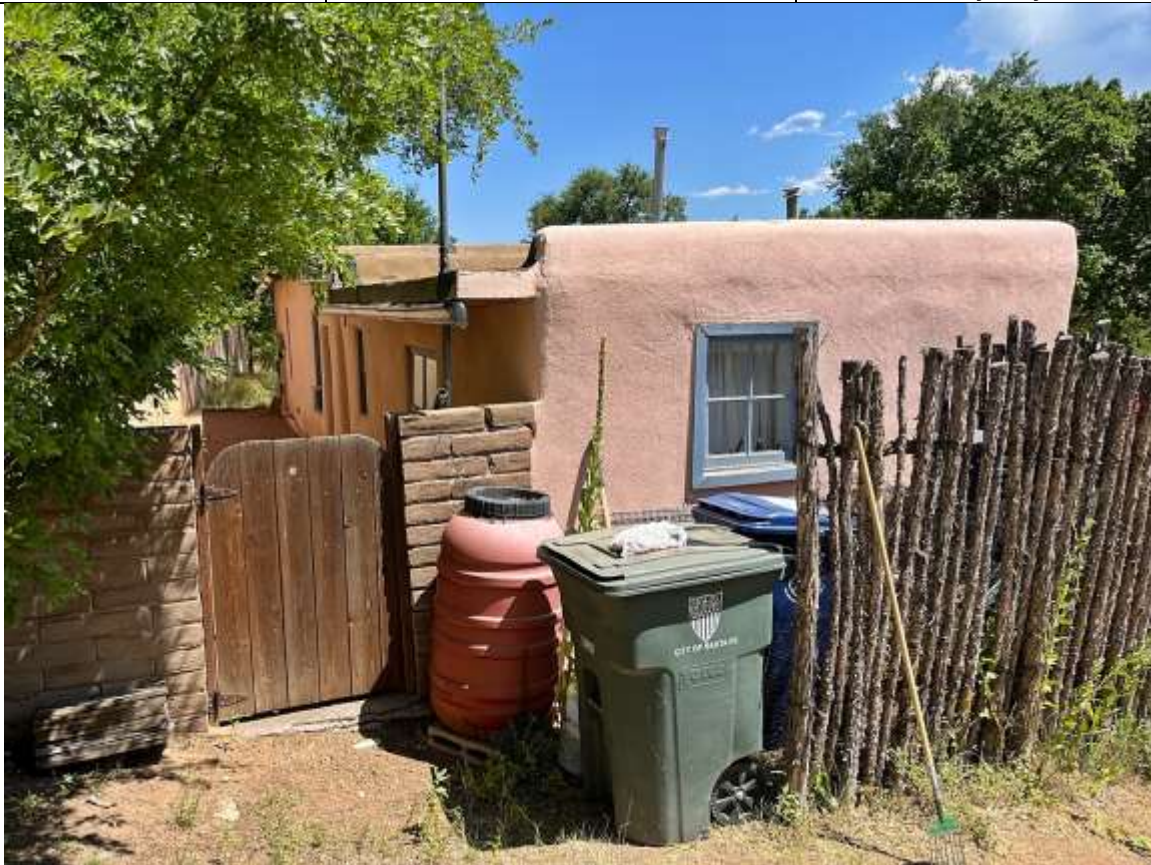
Photo 10: South elevation, assumed addition. Camera facing northeast.
