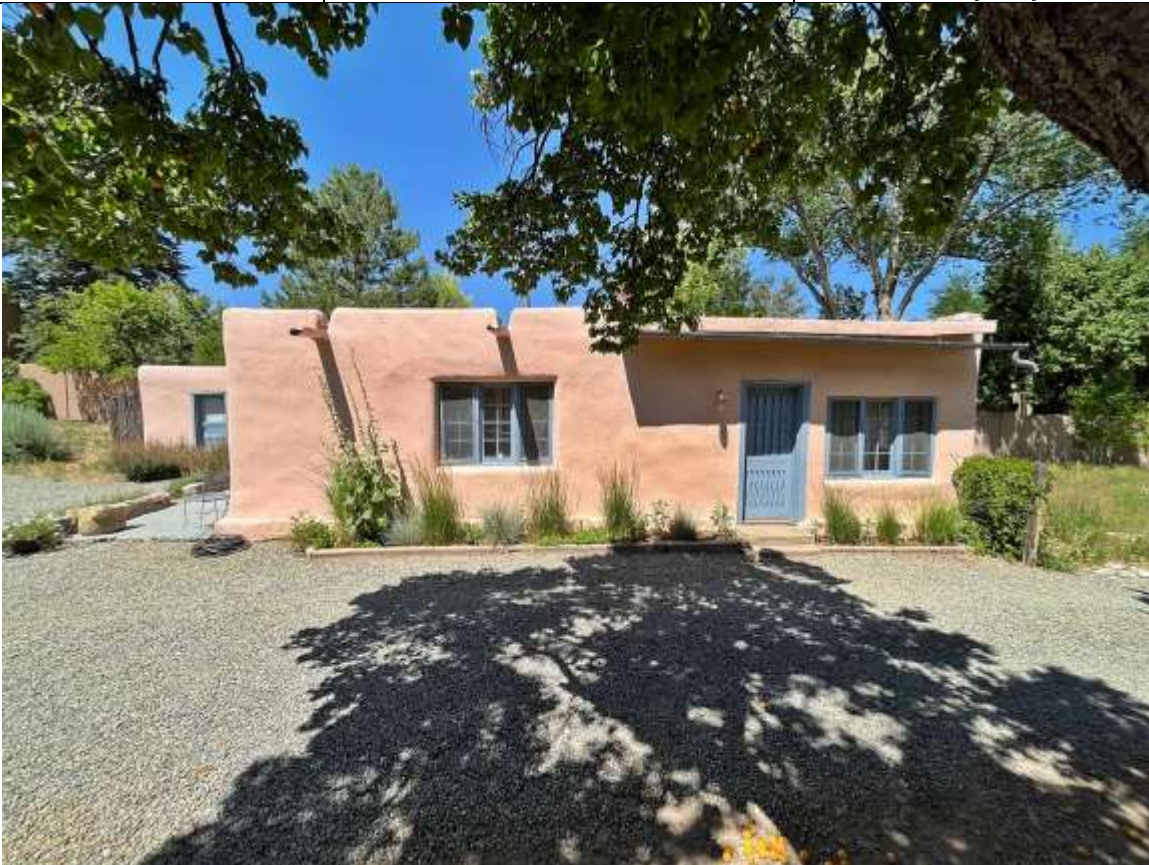
Photo 4: East elevation, assumed core block. Camera facing west.
