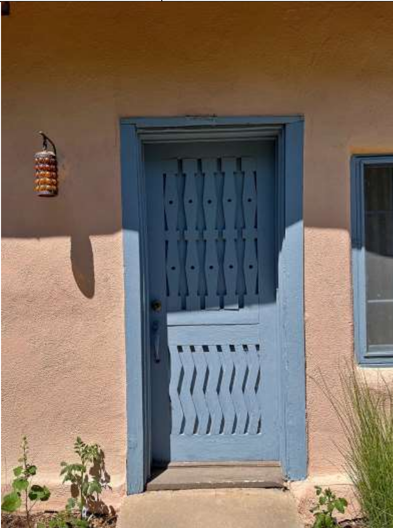
Photo 6: East elevation, assumed core block, entry door. Camera facing west.
