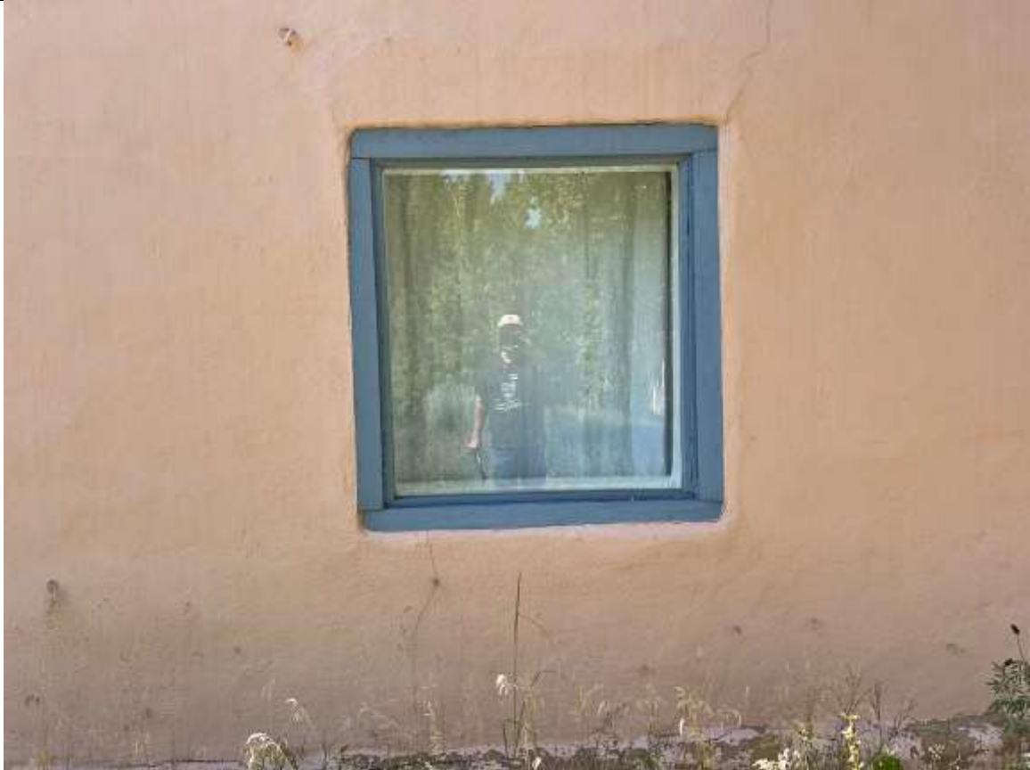
Photo 12: North elevation, assumed addition, window. Camera facing south.
