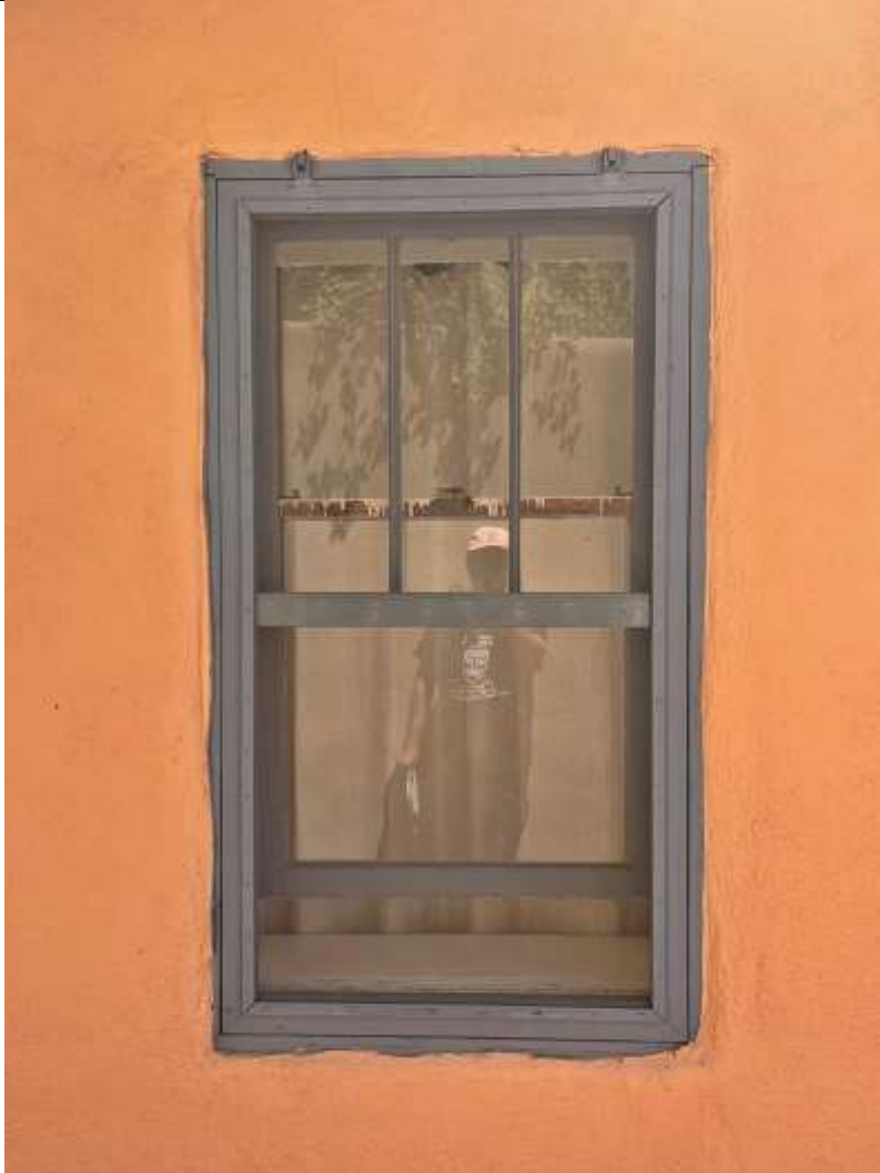
Photo 14: West elevation, typical window with screen. Camera facing east.
