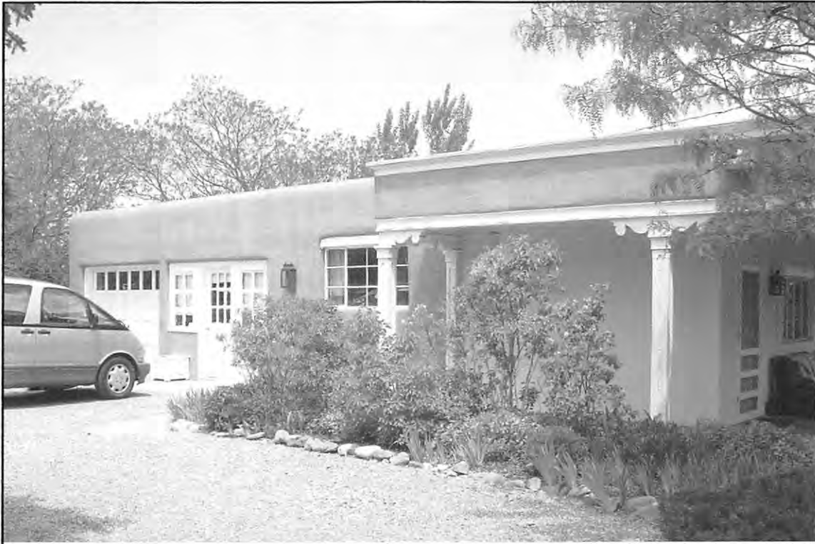
PHOTOGRAPH VIEW: south elevation
