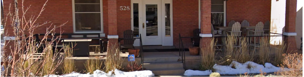
Figure 3: Railing on street facing elevation of twin structure at 528 Don Gaspar
