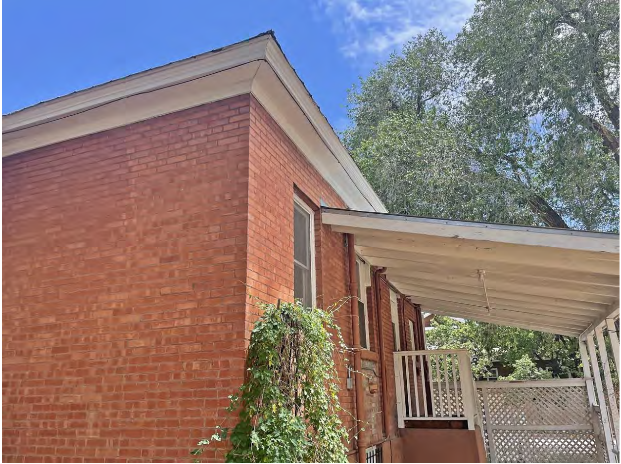
Figure 10: Porch, as viewed from north property line.
