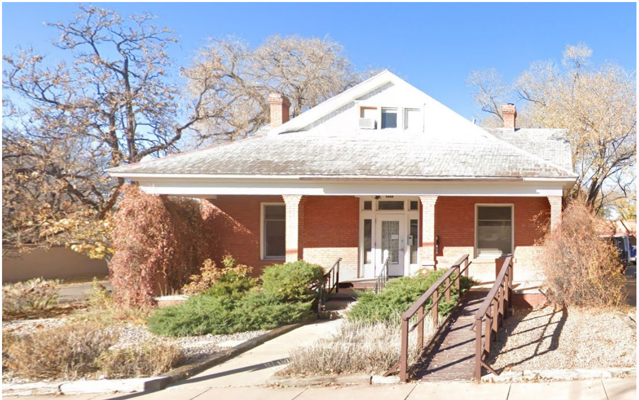
Figure 1: Front Façade of Structure prior to construction, circa November 2021
