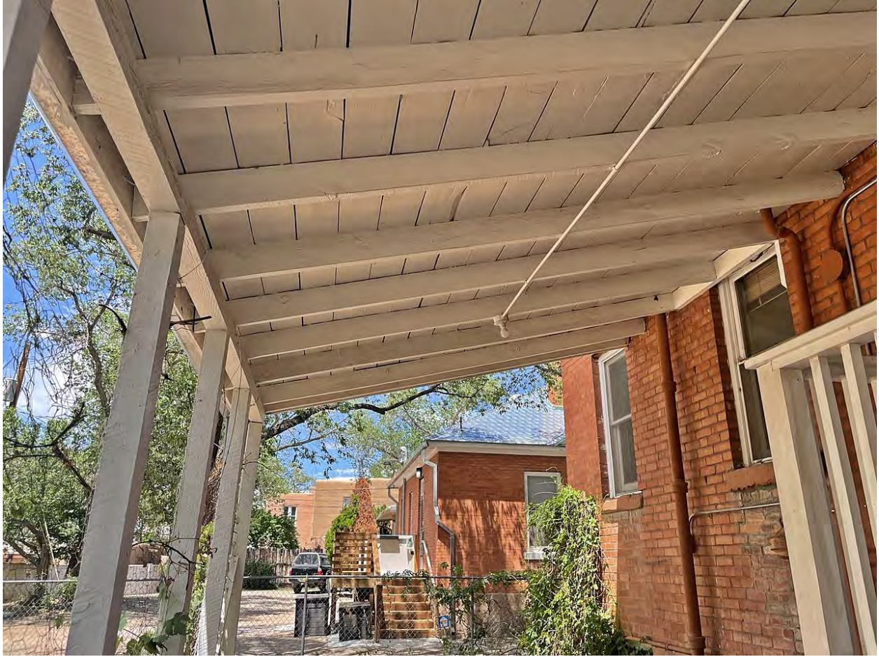
Figure 11: Porch posts and decking.
