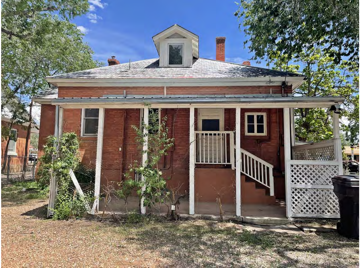
Figure 9: Porch, as viewed from parking court.
