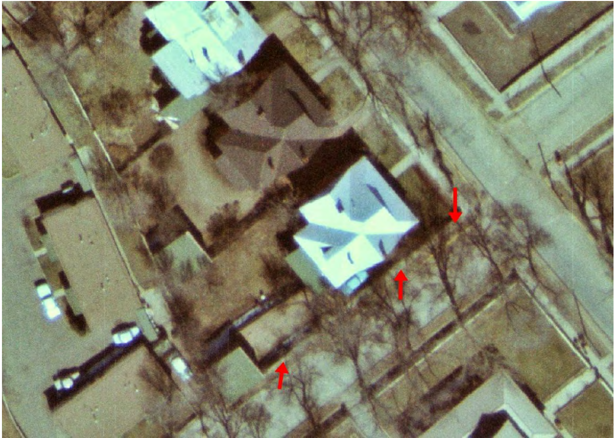
Figure 3: 1969 aerial photograph. South structure highlighted with arrows.
