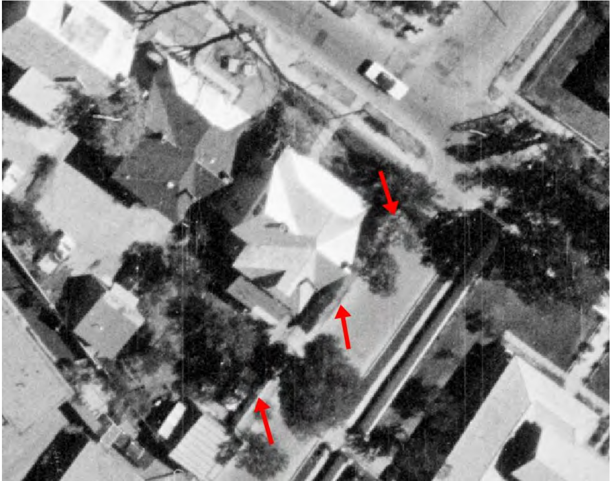
Figure 4: 1978 aerial photograph. South structure highlighted with arrows.
