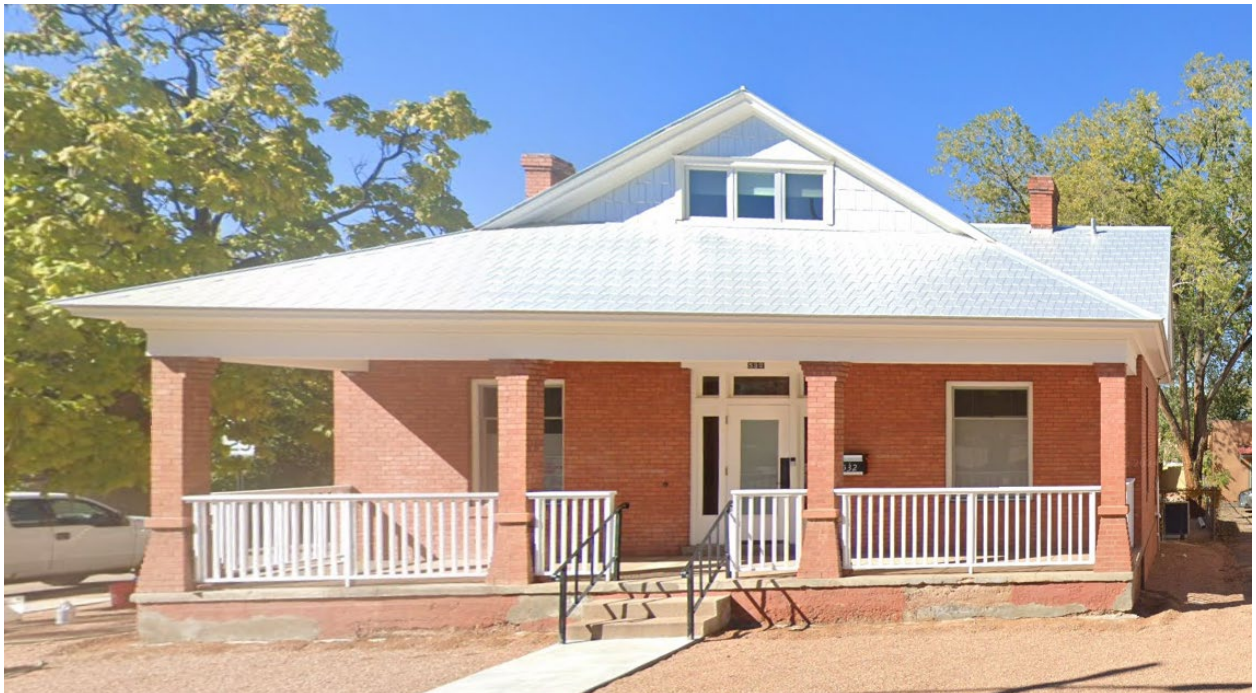
Figure 2: Alteration made in the field with the railing on the porch October 2024
