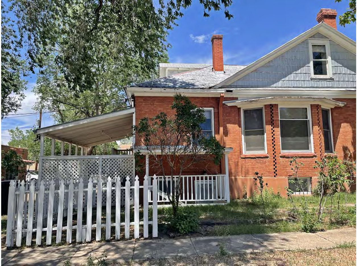
Figure 7: Porch, as viewed from West Santa Fe Avenue.
