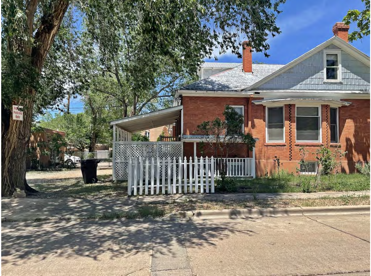
Figure 6: Porch, as viewed from West Santa Fe Avenue.
