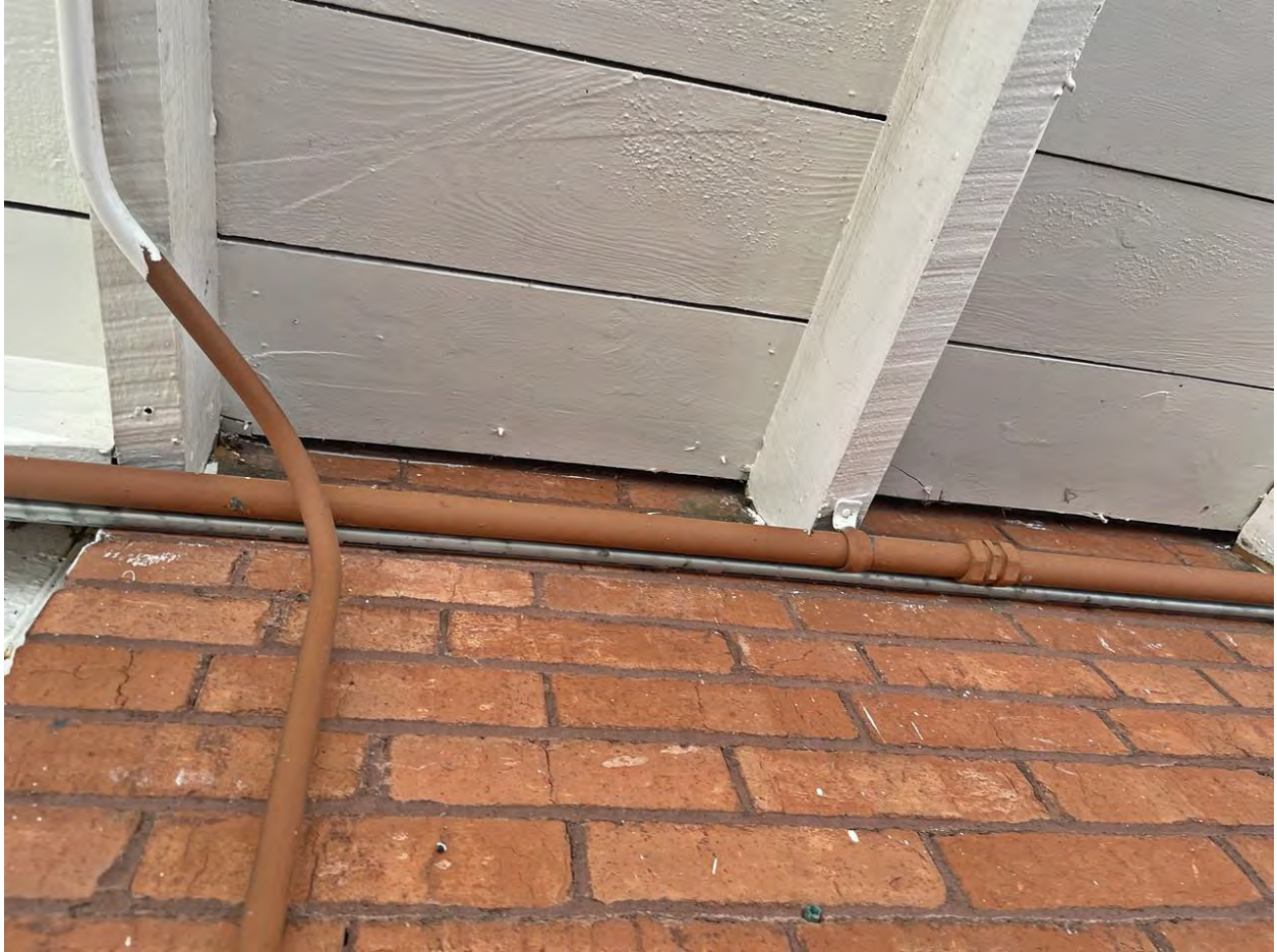
Figure 13: Porch attachment to brick house.
