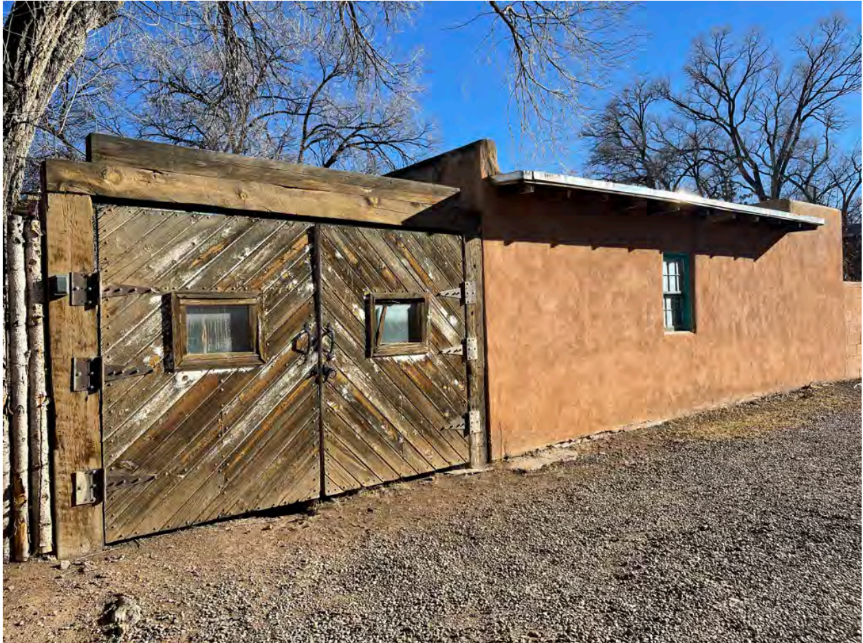
West facing façade at Access Easement
