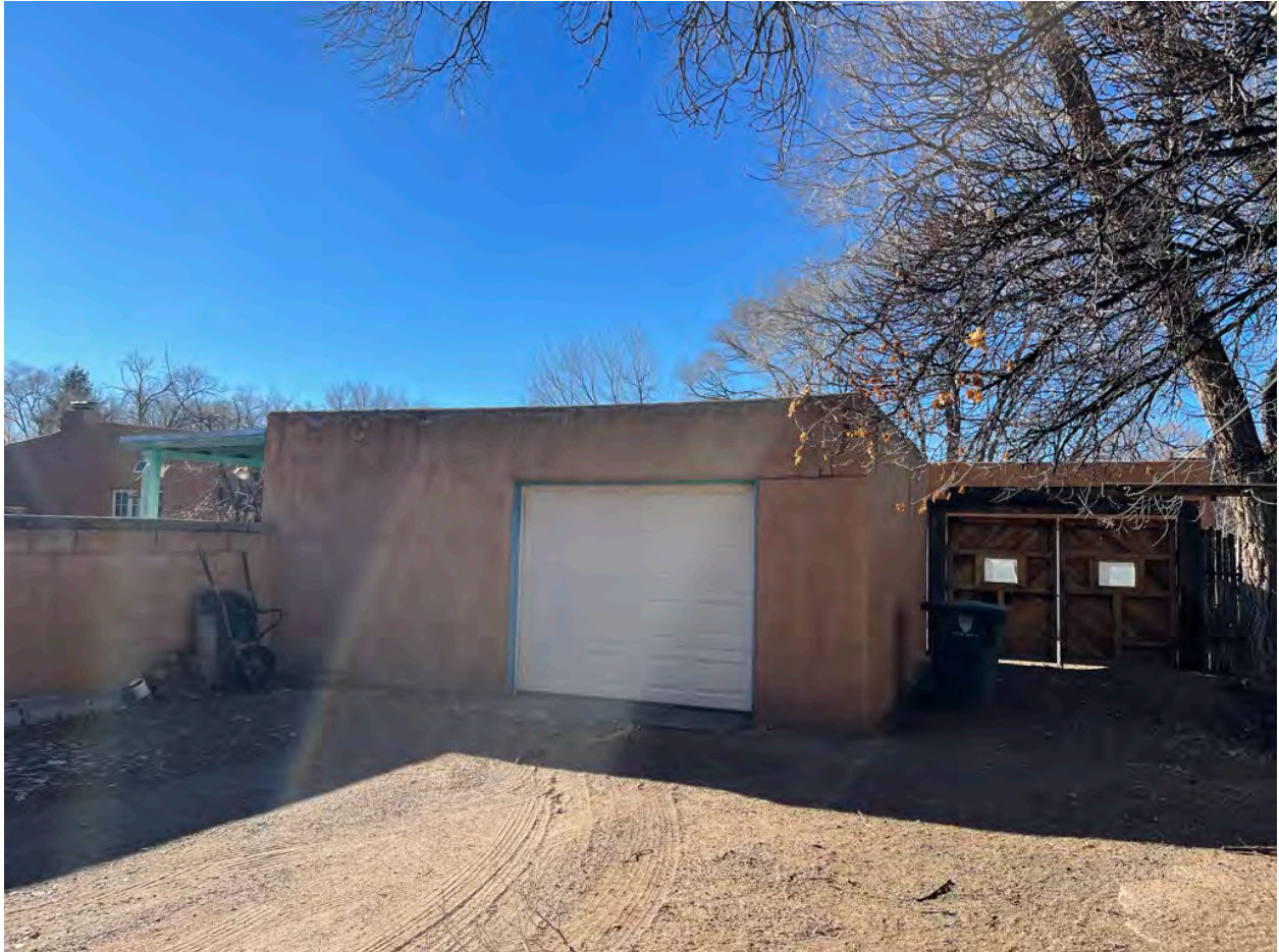
East façade of garage
