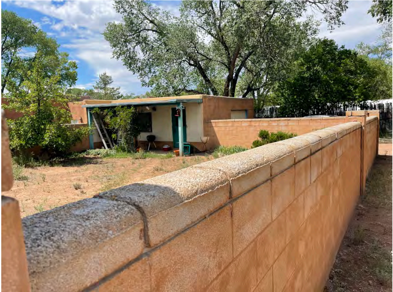
South façade of Garage
