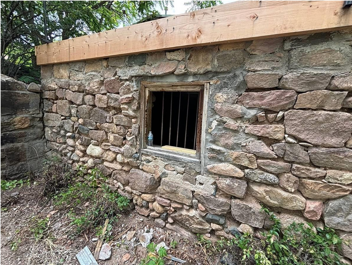
Photo 15: Stone structure. South elevation. Camera facing northwest. M. Kay, August 14, 2024.
