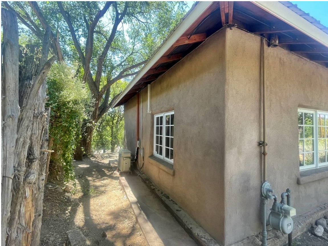
Photo 9: East elevation oblique. This façade likely represents original, unaltered construction. Camera facing southwest.
