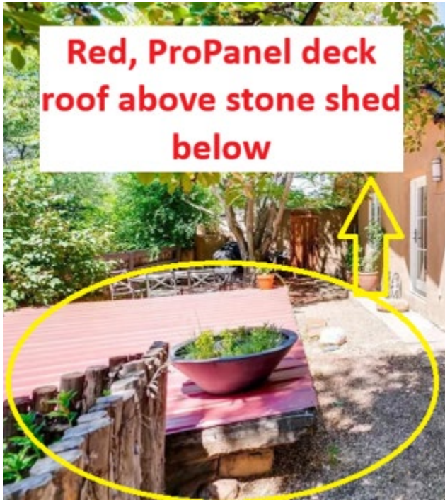
Figure 6: Previous red panel roof on the shed
