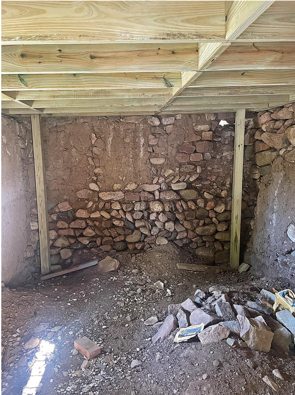
Photo 17: Stone structure. Interior. Camera facing west.
