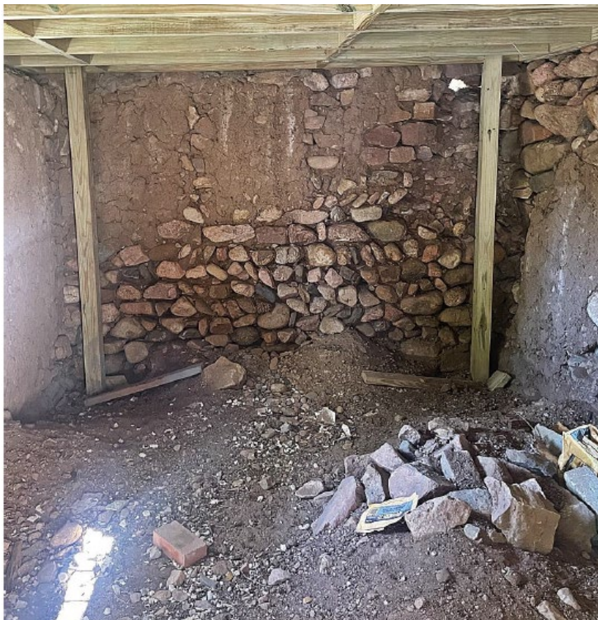
Figure 5: Stone shed structure interior
