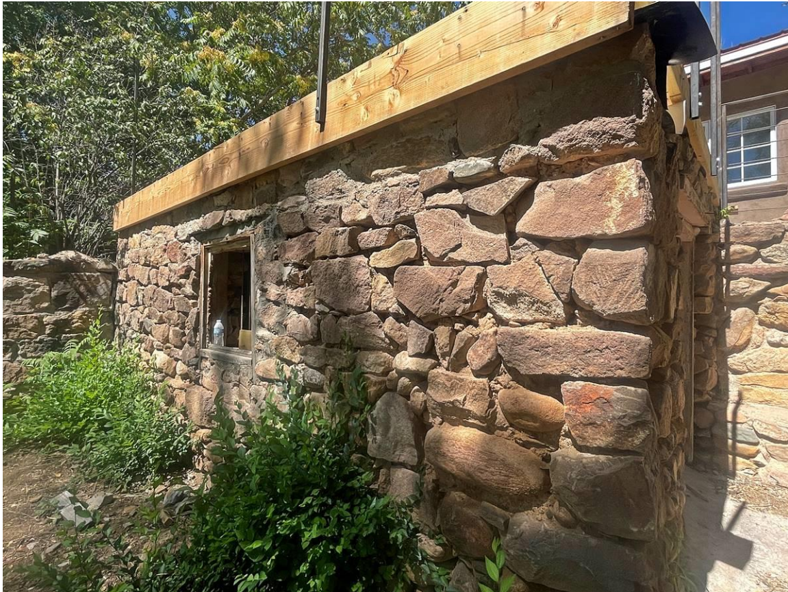
Photo 14: Stone structure. South elevation. Camera facing northwest.
