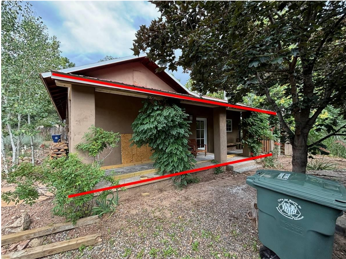
Photo 3: West elevation. Camera facing southeast. Craftsman-style porch (highlighted) postdates 1978. M. Kay, August 14, 2024.
