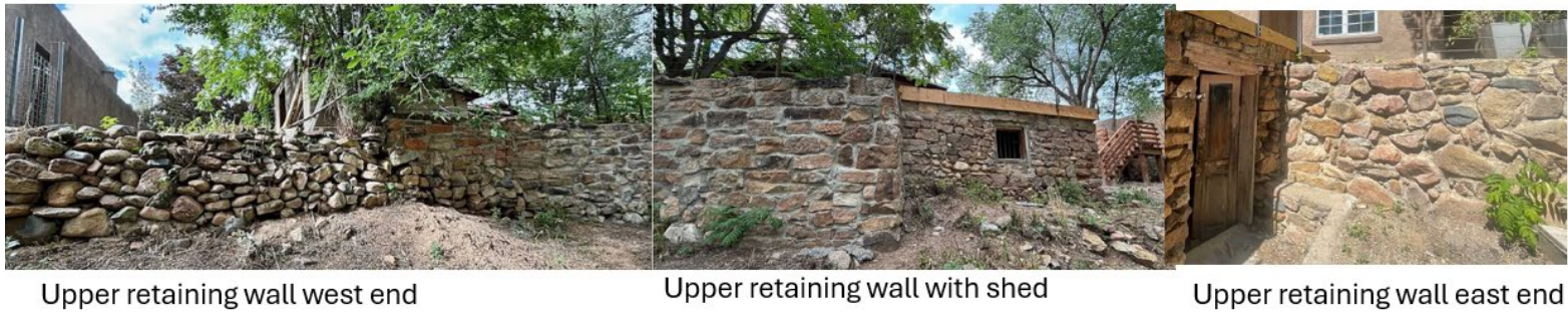
Figure 2: Upper retaining wall which shows in the 1960 aerial photograph
