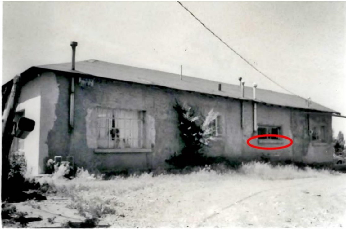
Figure 10: Copy of July 7, 1983, HBI survey photo taken by Michael Belshaw. Note presence of steel windows and lug sill at kitchen window (circle). Courtesy of NMCRIS.
