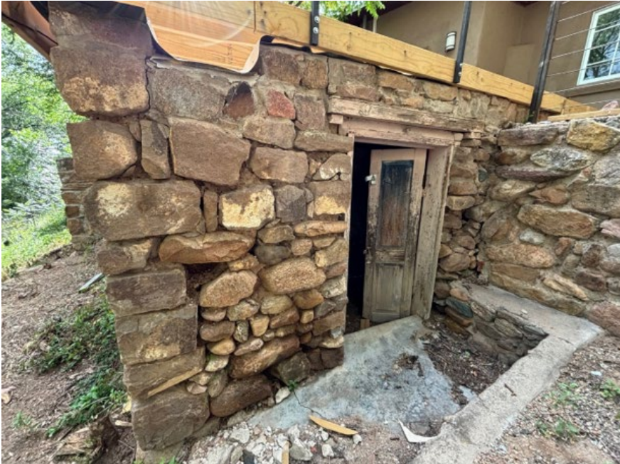
Figure 4: Exterior of the Shed
