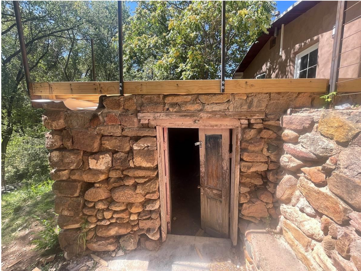
Photo 13: Stone structure. East elevation. Camera facing west.
