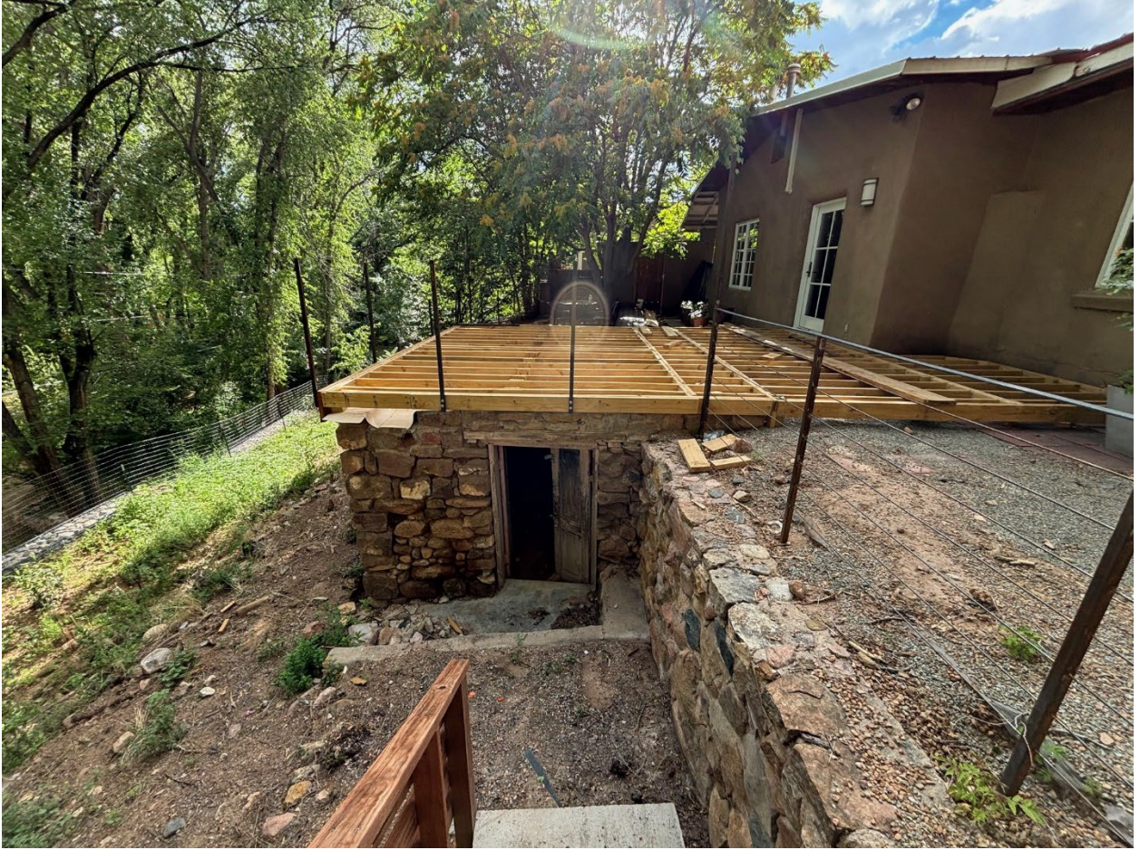
Another picture of the deck floating above the shed
