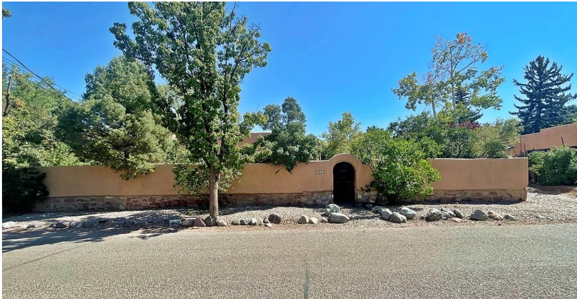
Photo 2: Front wall taken from street. Camera facing east.
