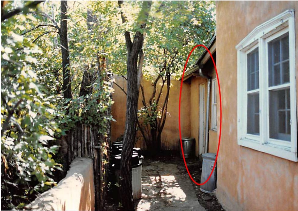
Figure 12: 1987 photograph east end of north elevation. Circle indicates change of wall position and fenestration. Compare with Photo 12. Courtesy of City of Santa Fe Historic Preservation Division.
