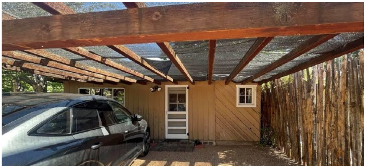
Figure 2: Guesthouse: west elevation under carport
