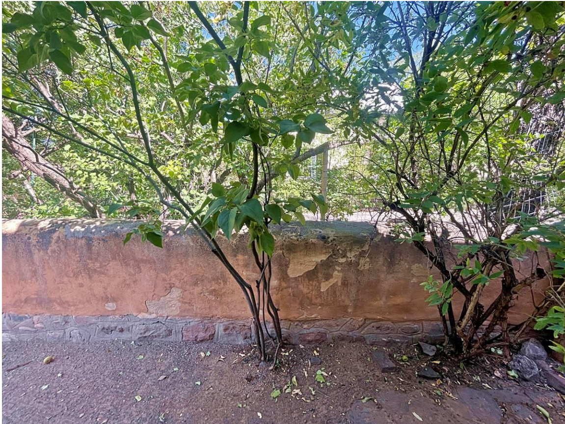
Photo 18: North property wall. Camera facing north.
