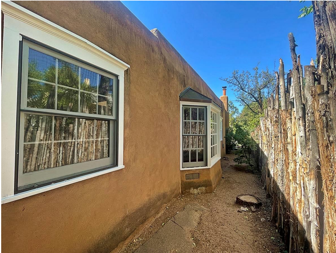
Photo 11: North elevation, east end. Camera facing southwest.
