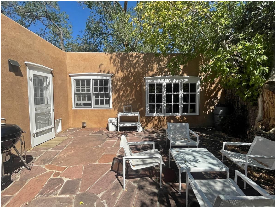
Photo 5: South elevation, primary bedroom suite. Camera facing north.
