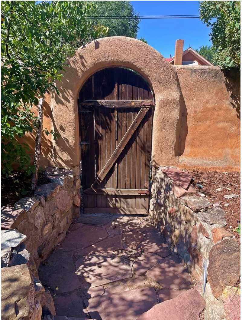
Photo 16: Front wall, entry gate. Camera facing west.
