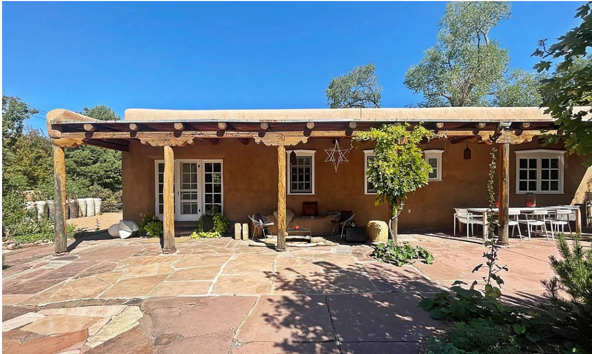
Photo 3: South elevation, west end. Camera facing north.
