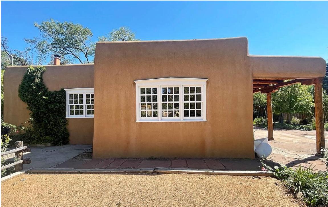
Photo 7: West elevation. Camera facing east.
