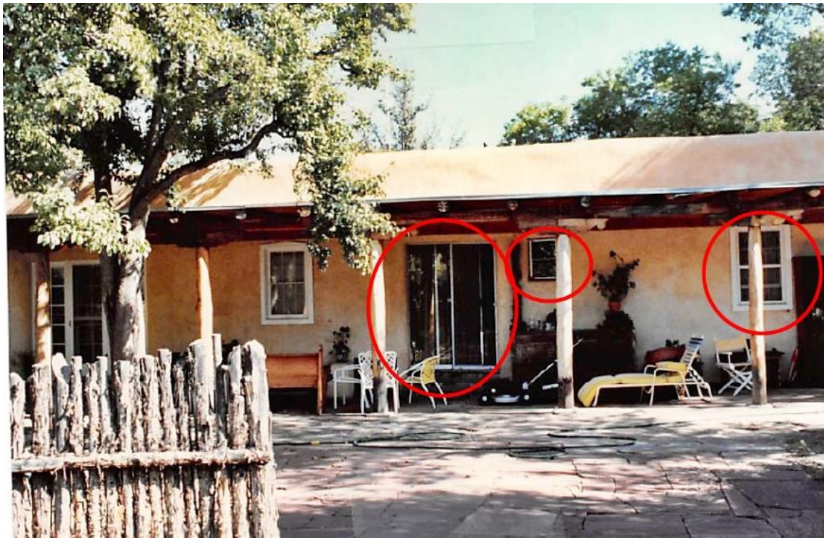
Figure 9: 1987 photograph of south elevation. Circles indicate fenestration that was changed by either elimination or enlargement of opening. Compare with Photo 3. Courtesy of City of Santa Fe Historic Preservation Division.
