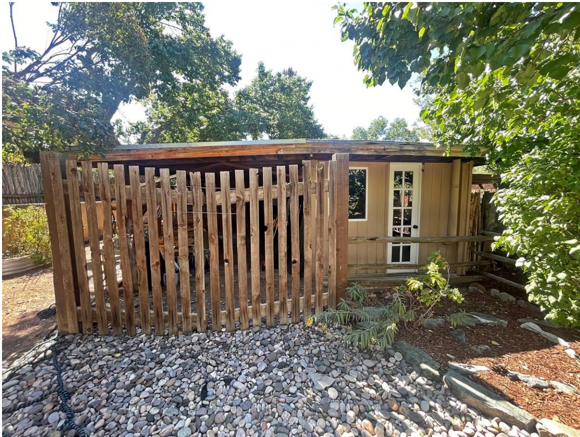
Photo 14: Guesthouse, north elevation. Camera facing south.
