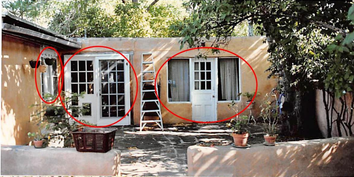
Figure 10: 1987 photograph of south elevation, primary bedroom suite. Circles indicate fenestration that was changed by new openings. Compare with Photos 5 & 6. Courtesy of City of Santa Fe Historic Preservation Division.
