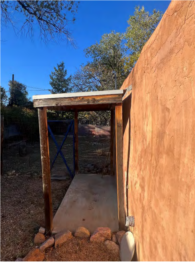
Existing Detached Portal – West Side Elevation
