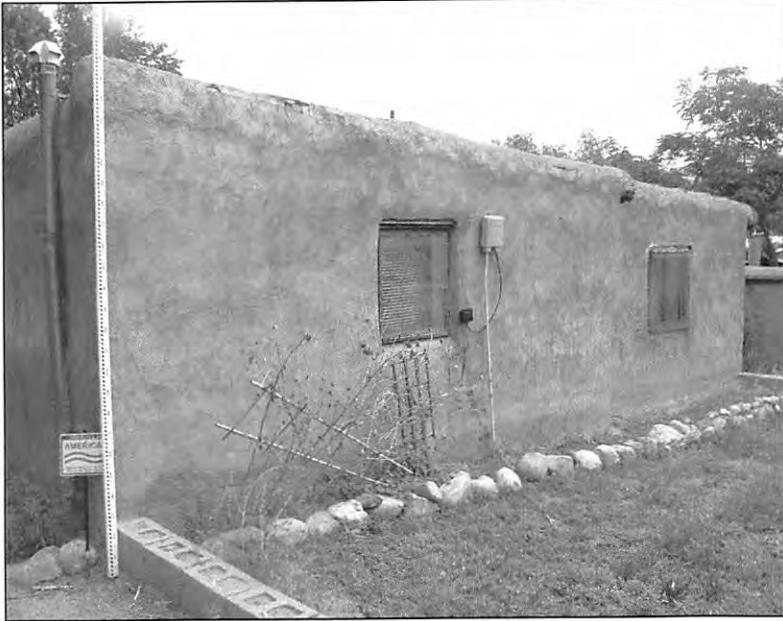
4. View northeast of south elevation. Concrete block stem wall is a structural, post-1958 alteration . Elevation at southwest corner measures 2.5 meters (8.2 feet), (ArcCom 07-20-06).
