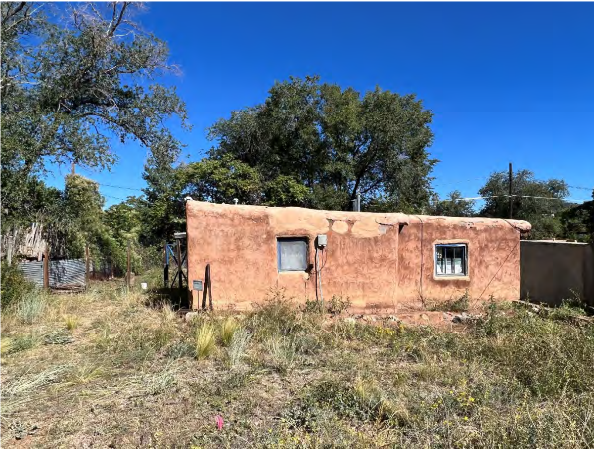
South Side – Residence Front Elevation
