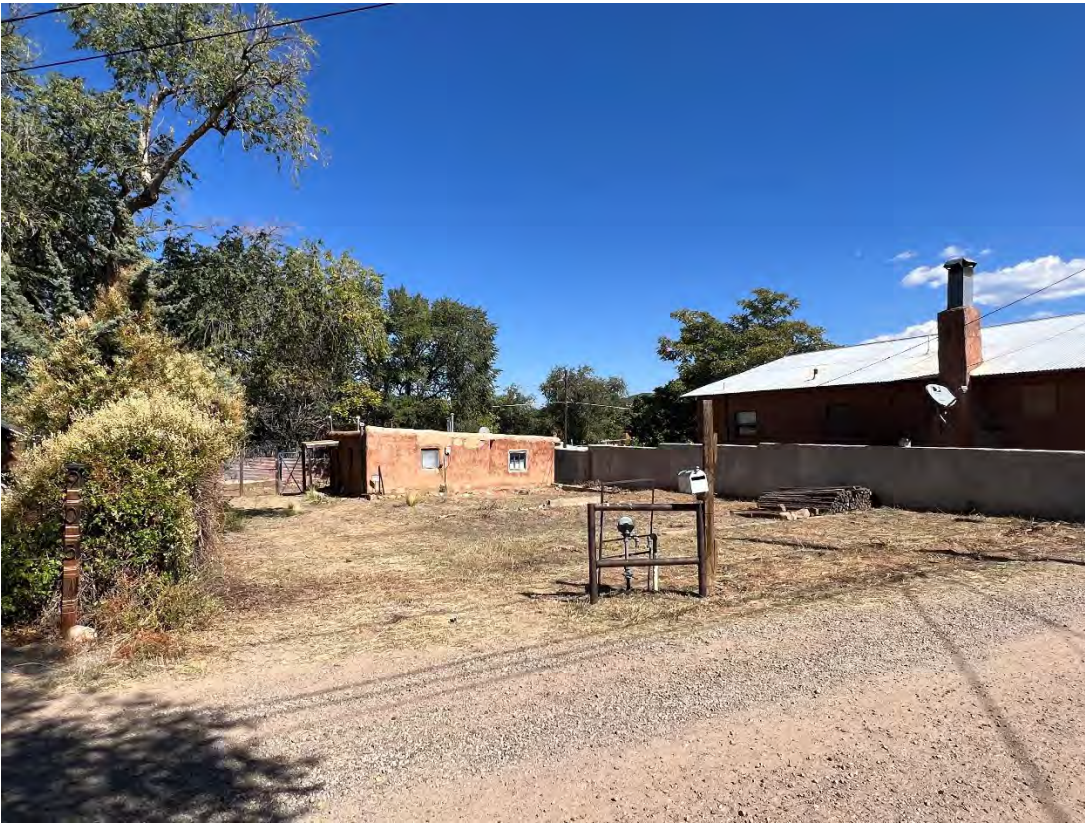
Don Miguel Place – Looking North East
