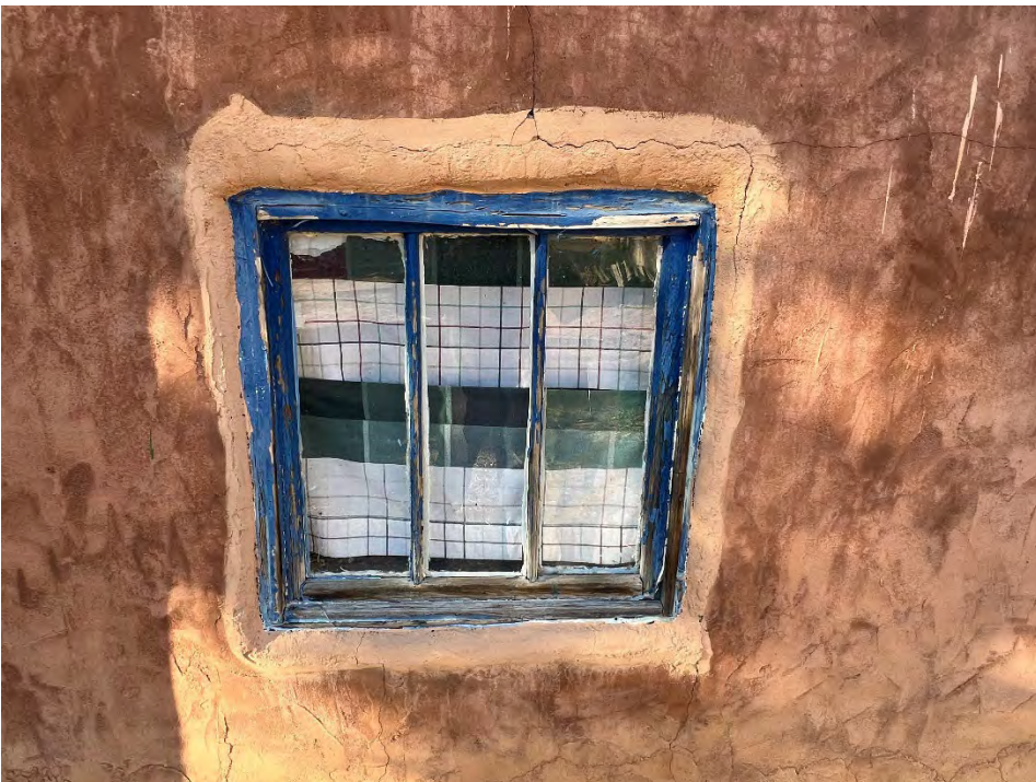
Existing Window - South Front Elevation
