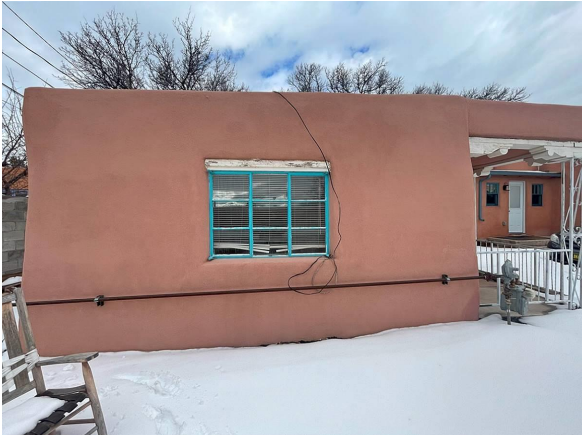
Photo 10: South elevation. Camera facing north.
