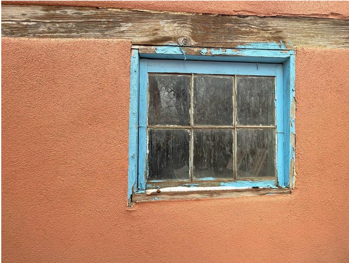
Photo 14: East elevation. Camera facing northwest.
