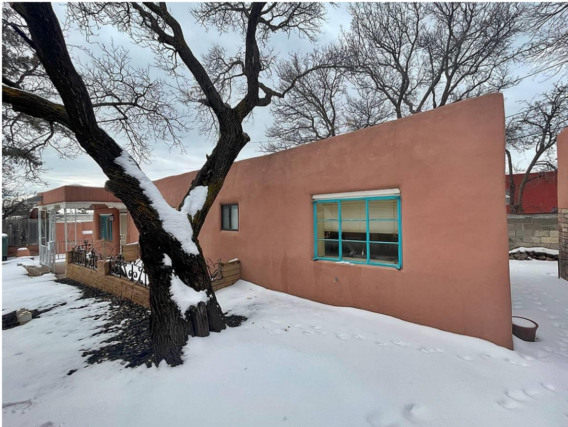
Photo 6: East elevation. Camera facing southwest.
