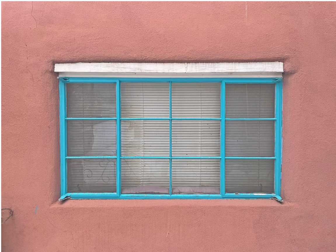
Photo 5: East elevation, bedroom window. Camera facing west.
