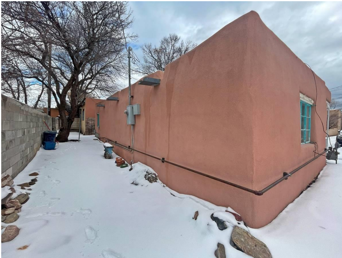
Photo 11: West and south elevations. Camera facing northeast.
