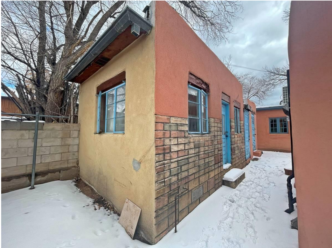
Photo 13: West and south elevations. Camera facing northeast.
