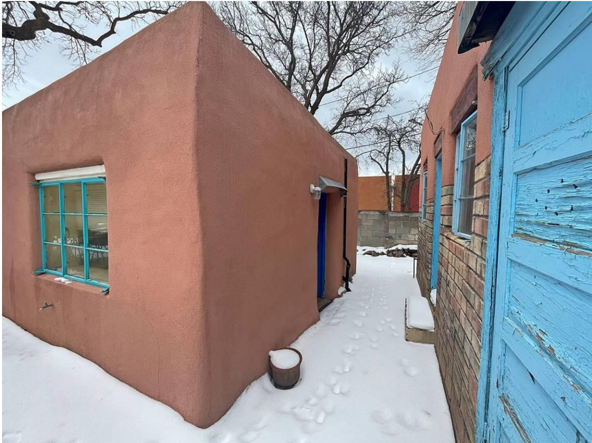
Photo 7: East and north elevations. Camera facing southwest.
