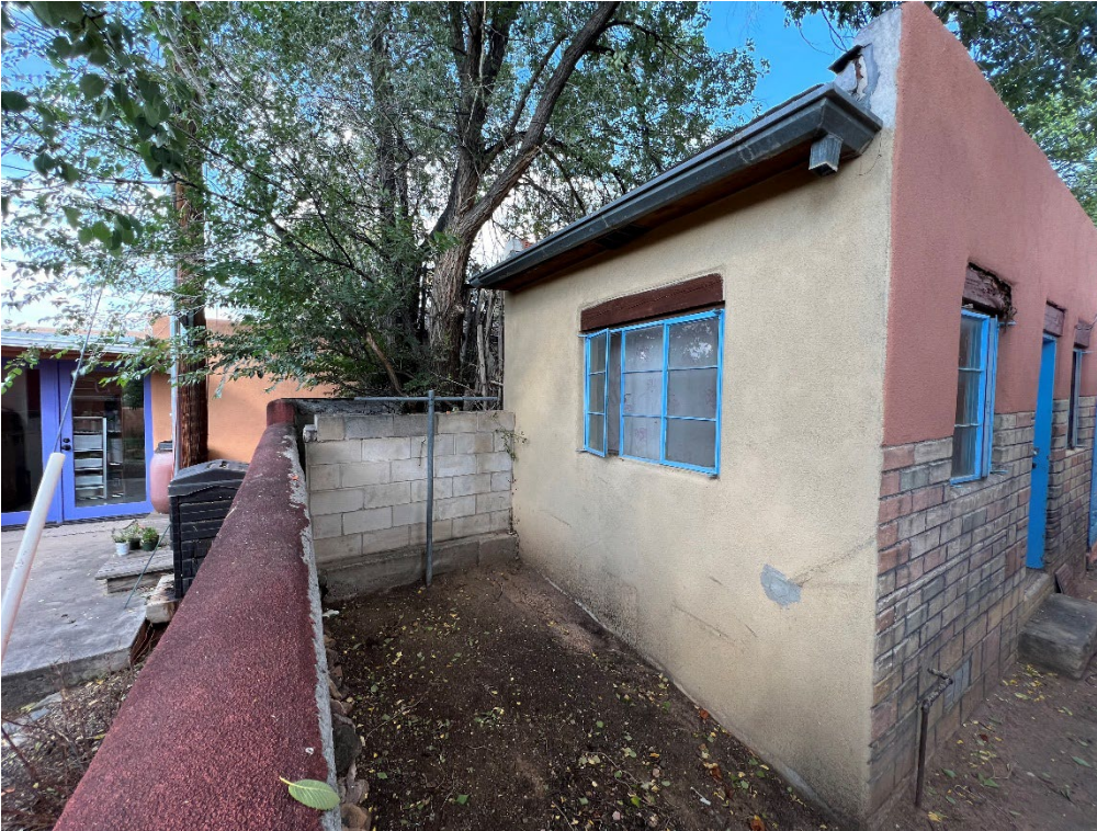
Storage Building – West Side Elevation
