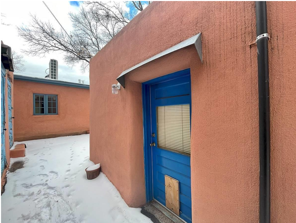
Photo 8: North elevation, entry. Camera facing southeast.
