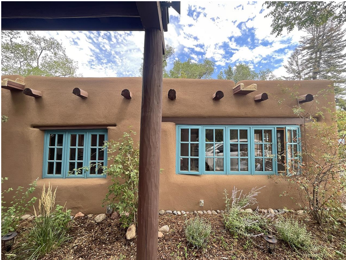
Photo 8: South elevation. Original portion of building after renovation. Camera facing north.
