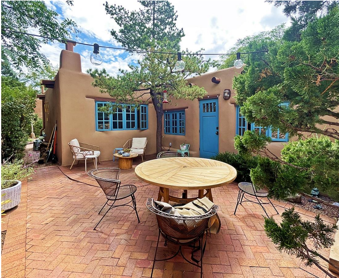
Photo 13: North elevation at courtyard. Original portion of building. Camera facing southeast.
