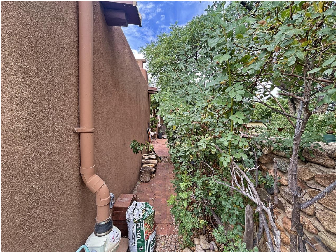
Photo 15: North elevation. Original portion of building. Camera facing west.
