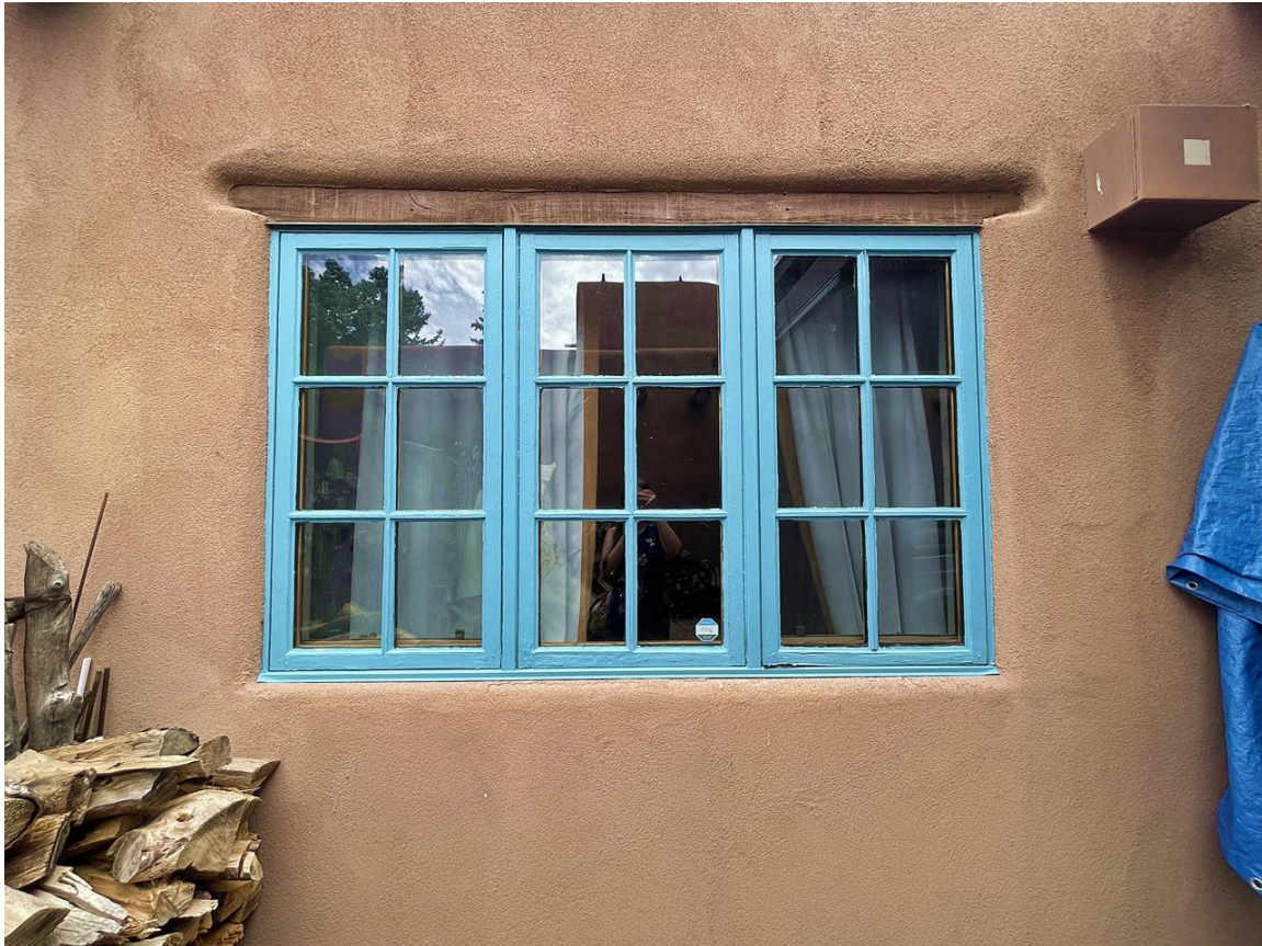
Photo 10: South elevation. Mid-1970s addition, window detail. Camera facing north.
