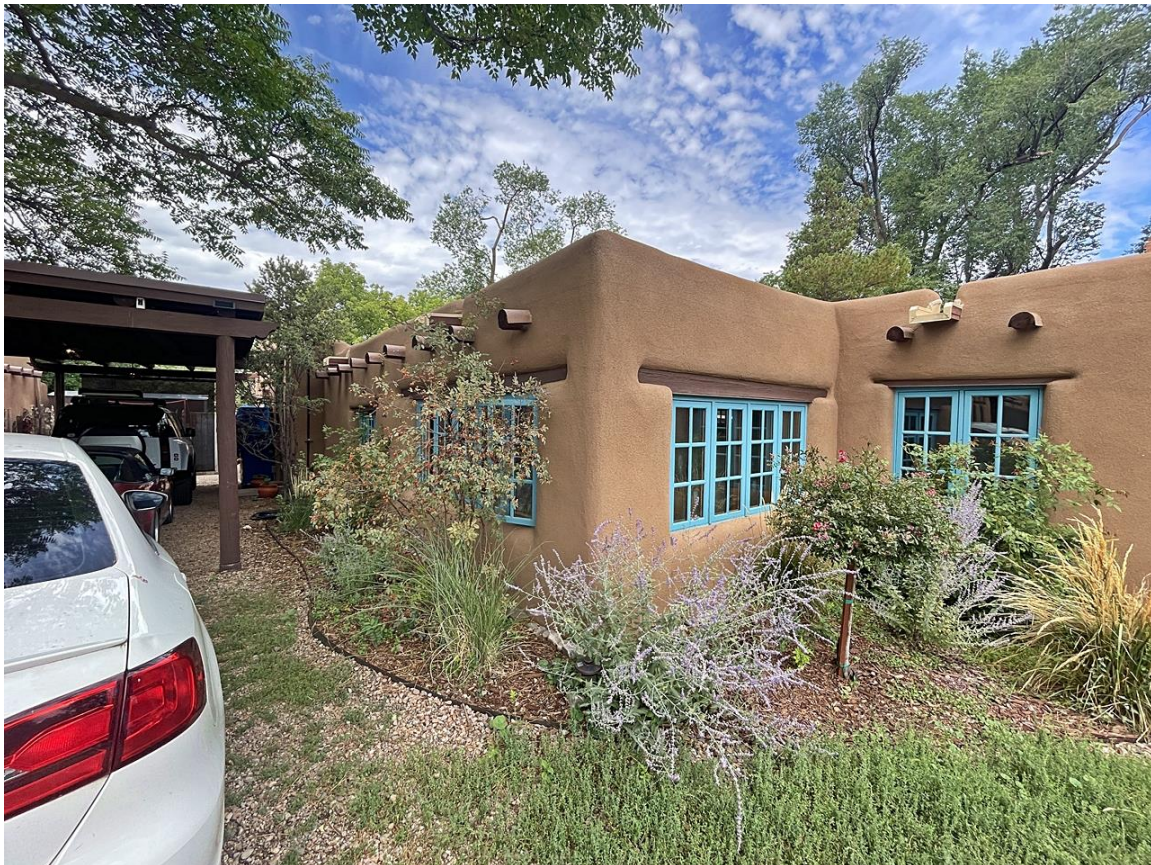
Photo 7: South elevation oblique and recent carport at left. Camera facing northwest.
