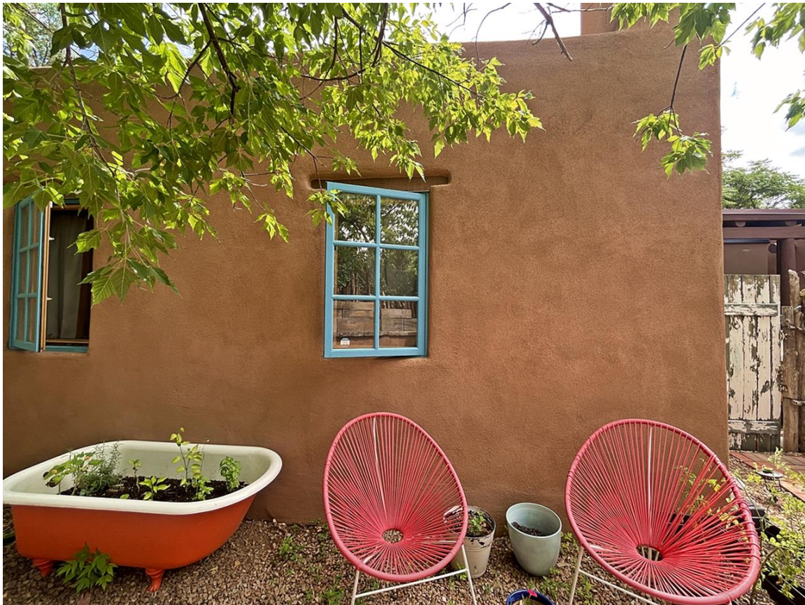
Photo 12: West elevation. Mid-1970s addition, south end. Camera facing east.
