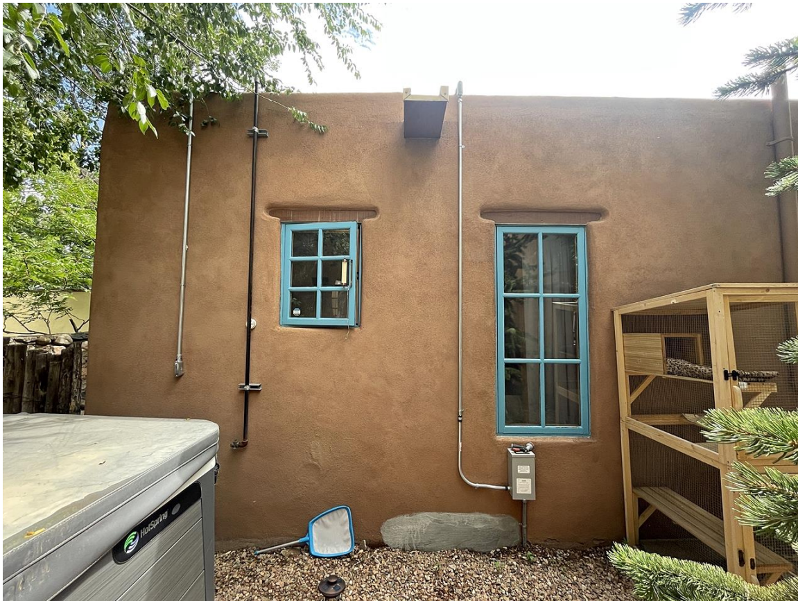
Photo 11: West elevation. Mid-1970s addition, north end. Camera facing east.
