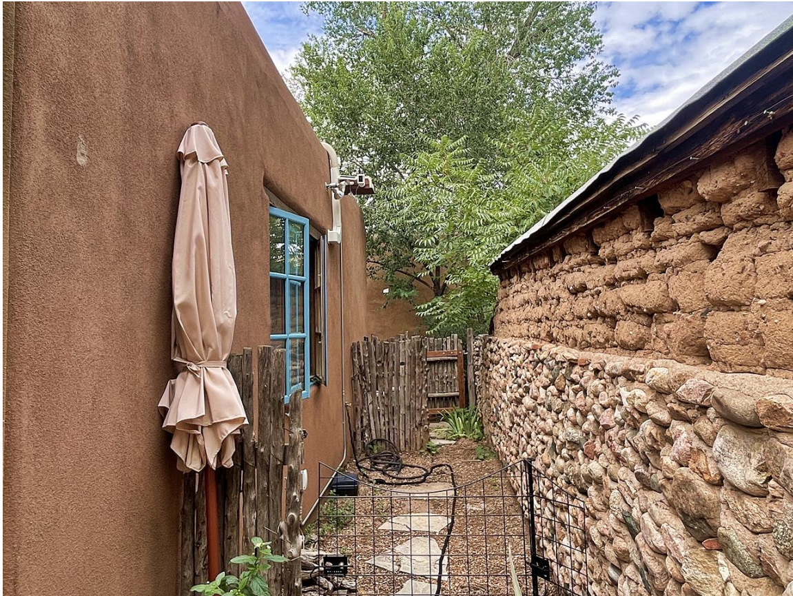
Photo 16: North elevation. Mid-1970s addition. Camera facing west.
