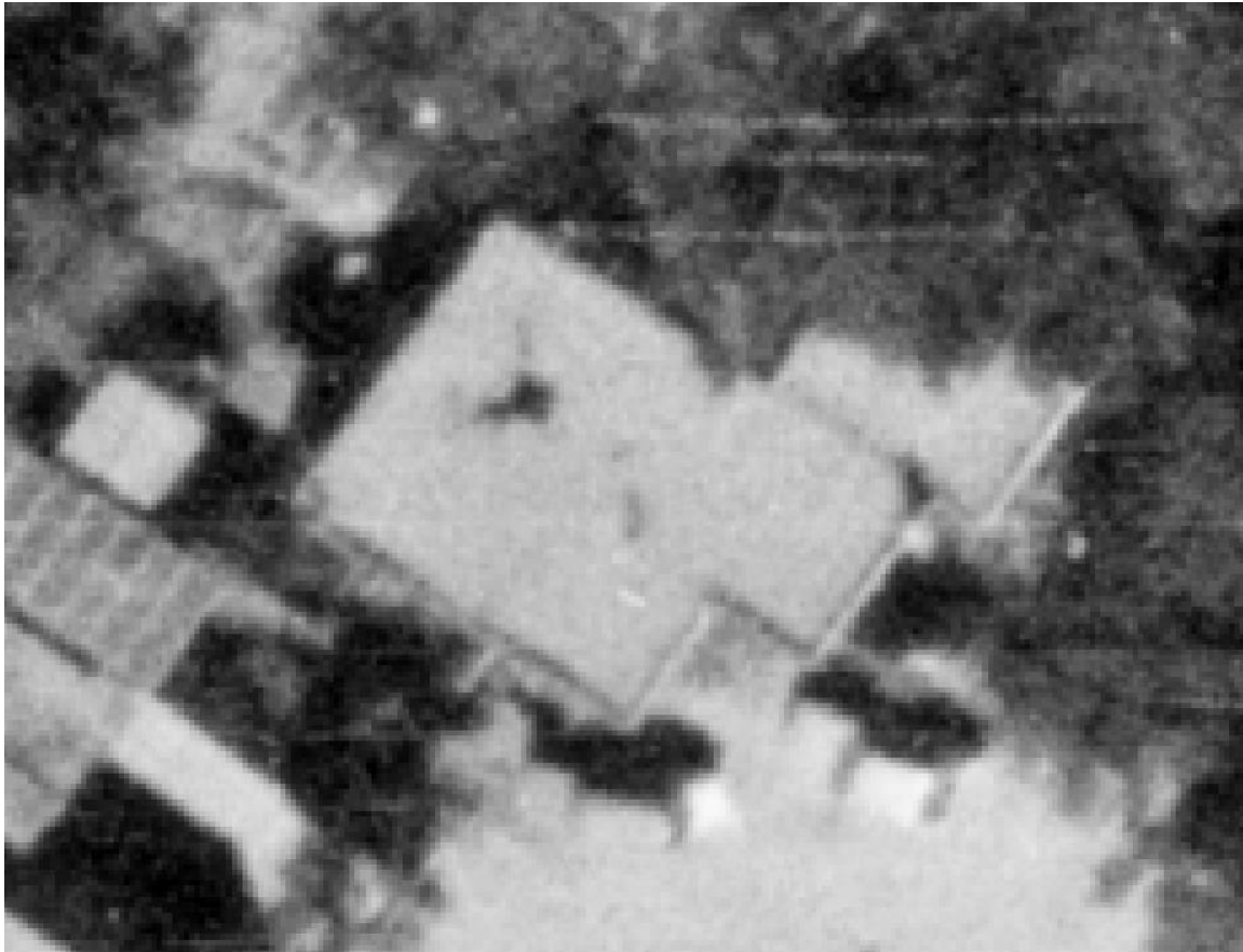
Figure 8: September 11, 1978, aerial photograph. Note absence of present west addition.
