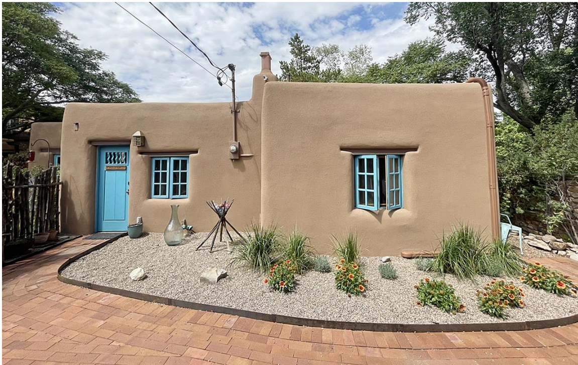
Photo 5: East elevation at entry. Camera facing west.
