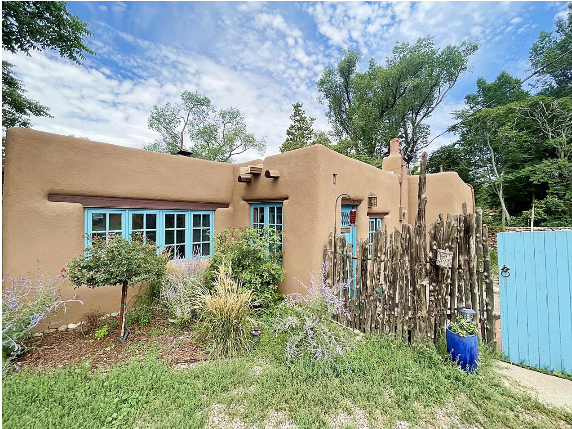
Photo 4: East elevation oblique. Camera facing northwest.
