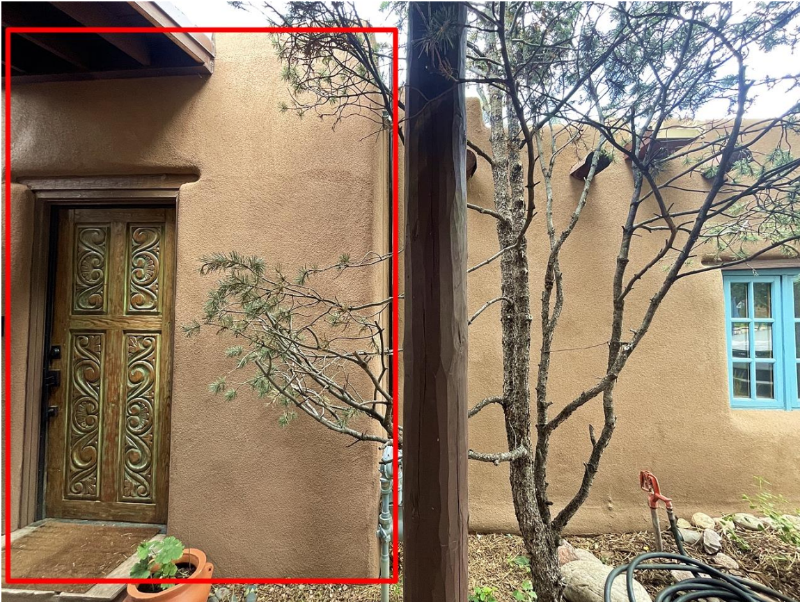
Photo 9: South elevation. Mid-1970s addition highlighted in red. Camera facing north.
