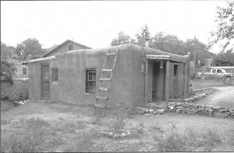
2. View south of north (left) and west (right) elevation. Frame portal on west elevation is a post-1958 alteration (ArcCom 07-20-06).
