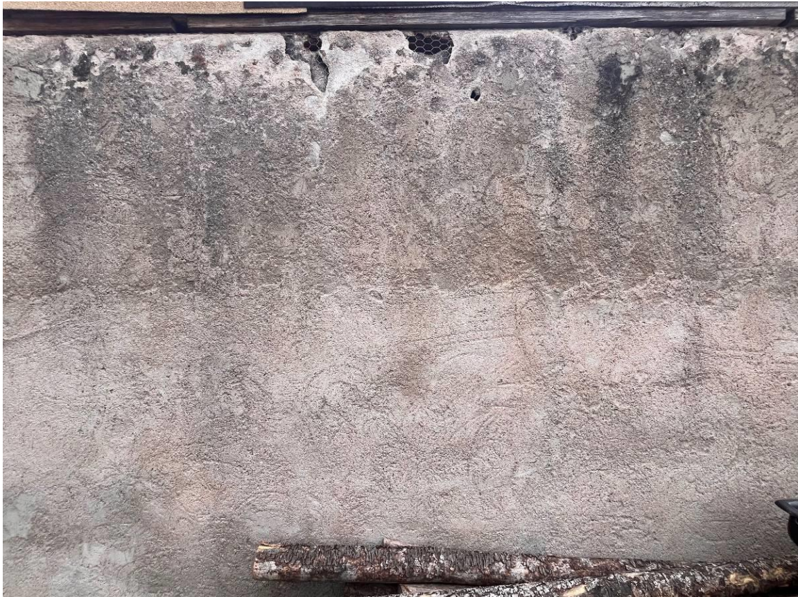
Photo 11: North elevation. Camera facing southeast.
