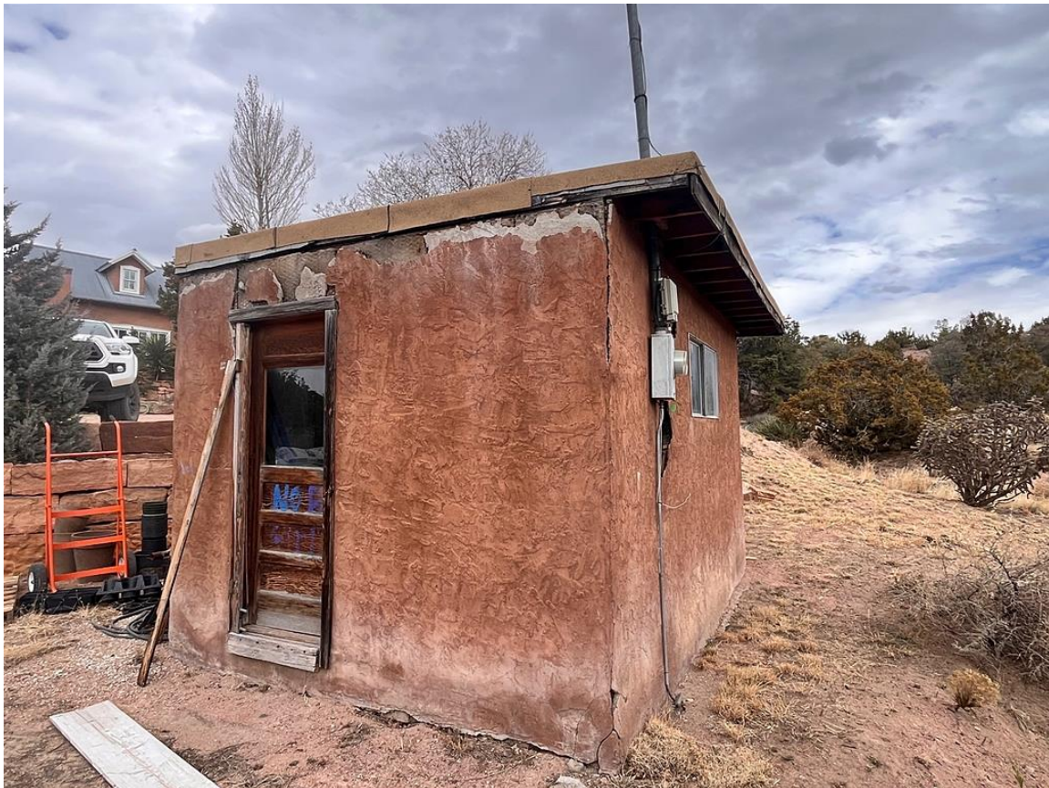
Photo 8: West and south elevations. Camera facing northeast.
