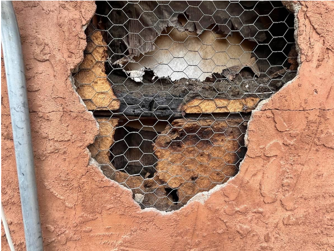
Photo 6: Break in south elevation revealing construction technique. Camera facing north.
