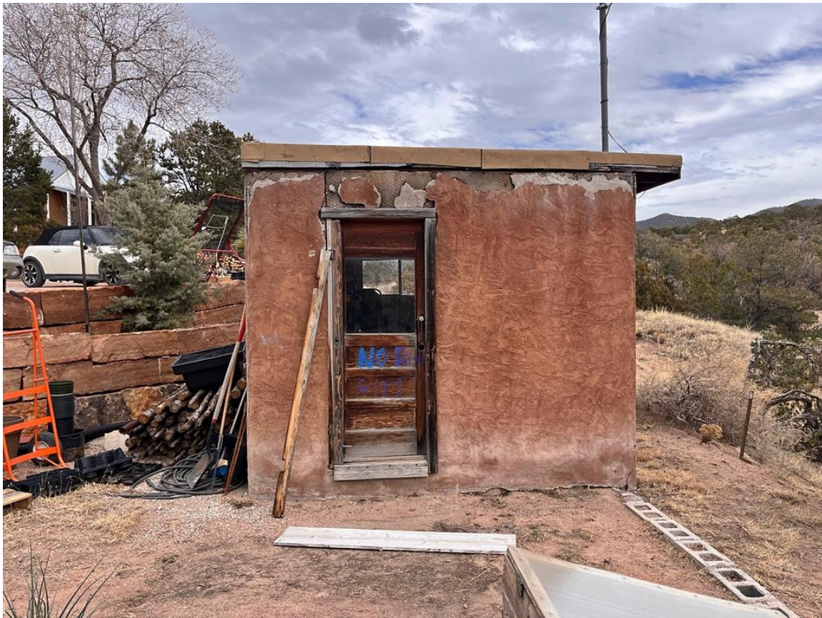
Photo 5: West elevation. Camera facing northeast.
