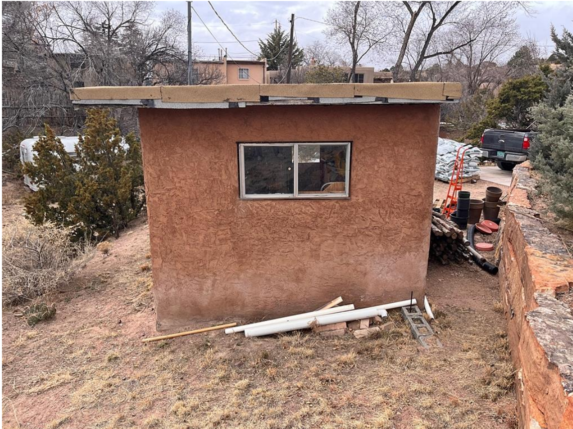
Photo 10: East elevation. Camera facing southwest.
