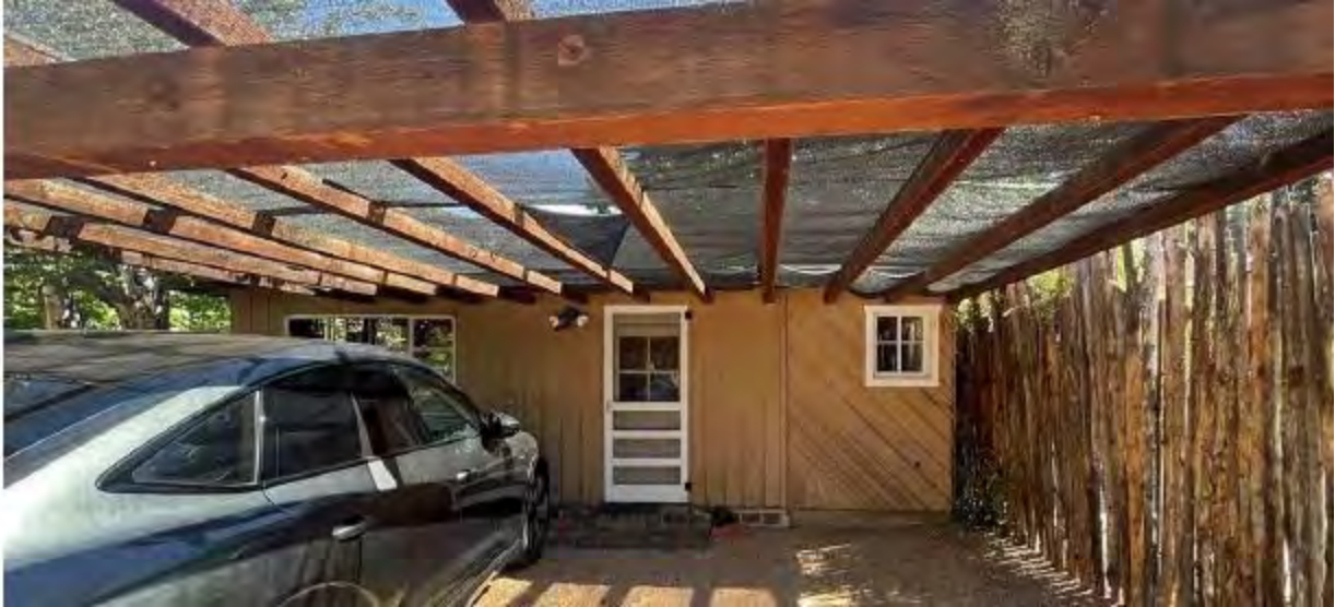
Figure 2: Guesthouse: west elevation under carport
