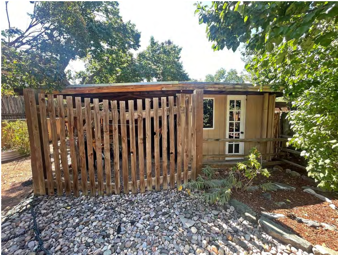
Photo 14: Guesthouse, north elevation. Camera facing south.
