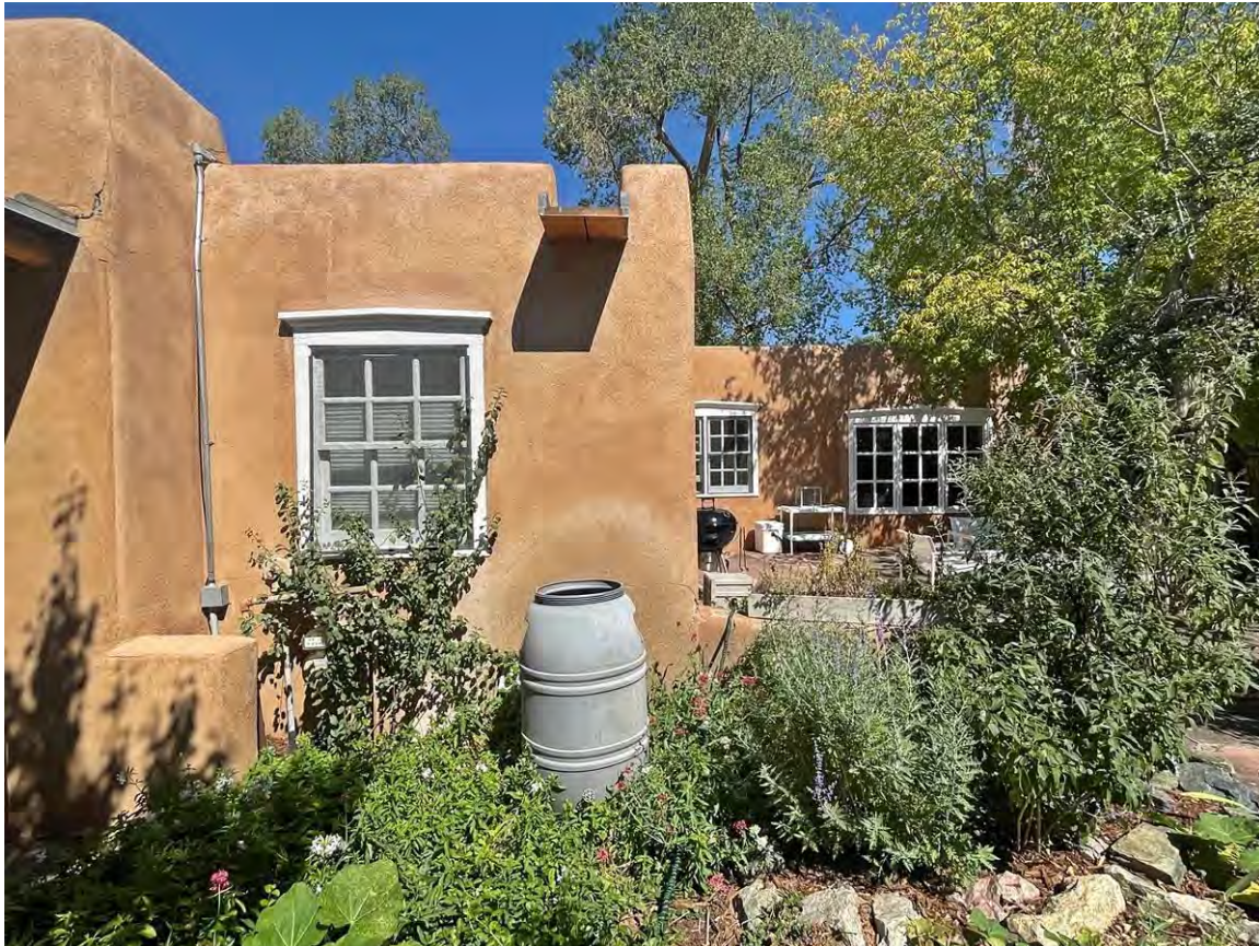
Photo 4: South elevation, east end and presumed enclosed porch. Camera facing north.
