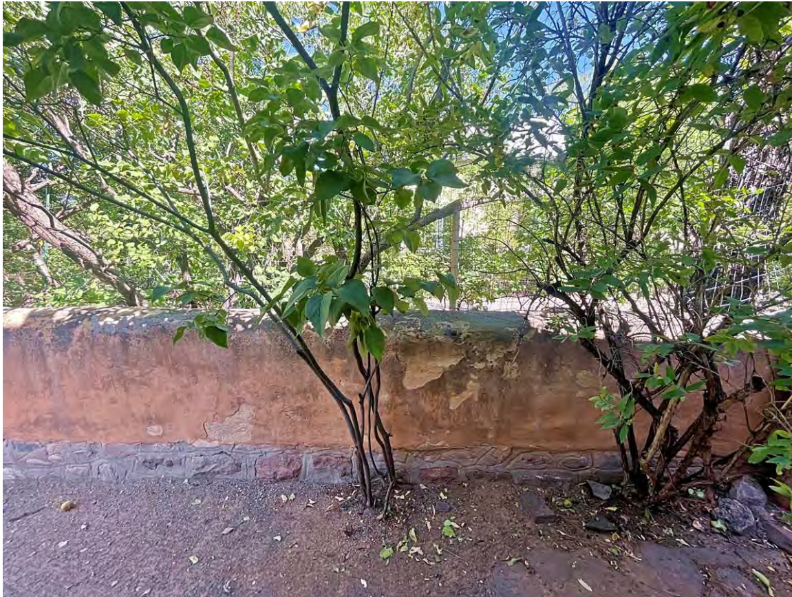
Photo 18: North property wall. Camera facing north.
