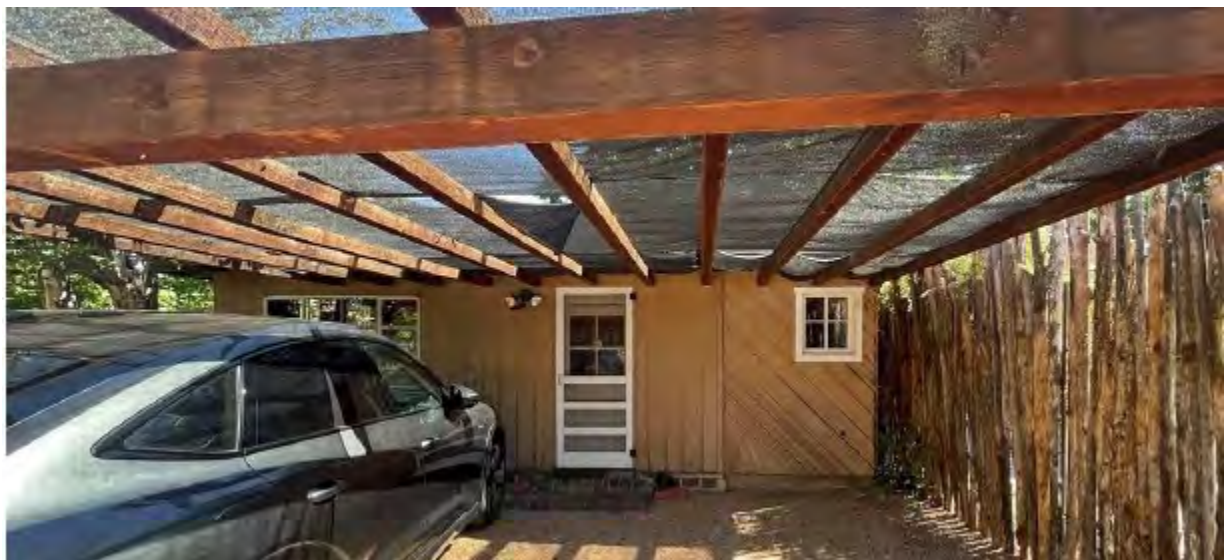
Figure 2: Guesthouse: west elevation under carport
