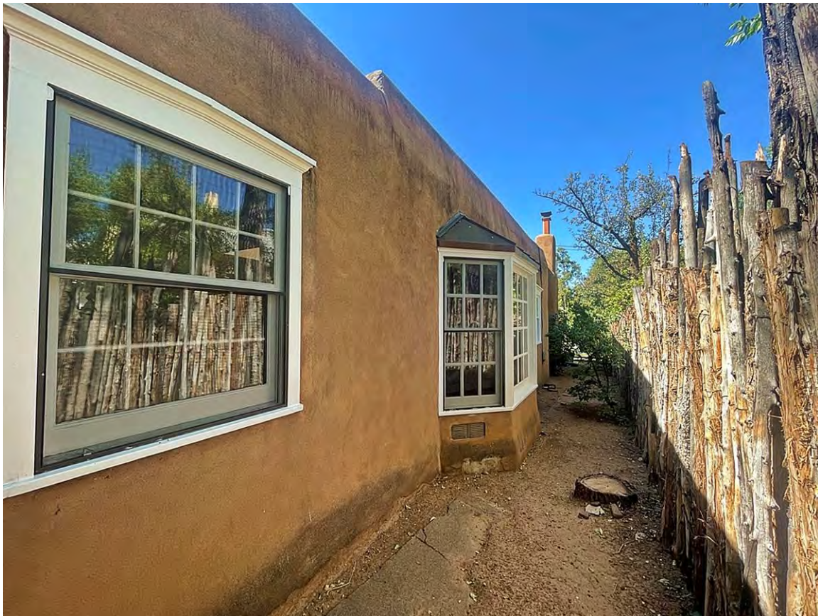
Photo 11: North elevation, east end. Camera facing southwest.
