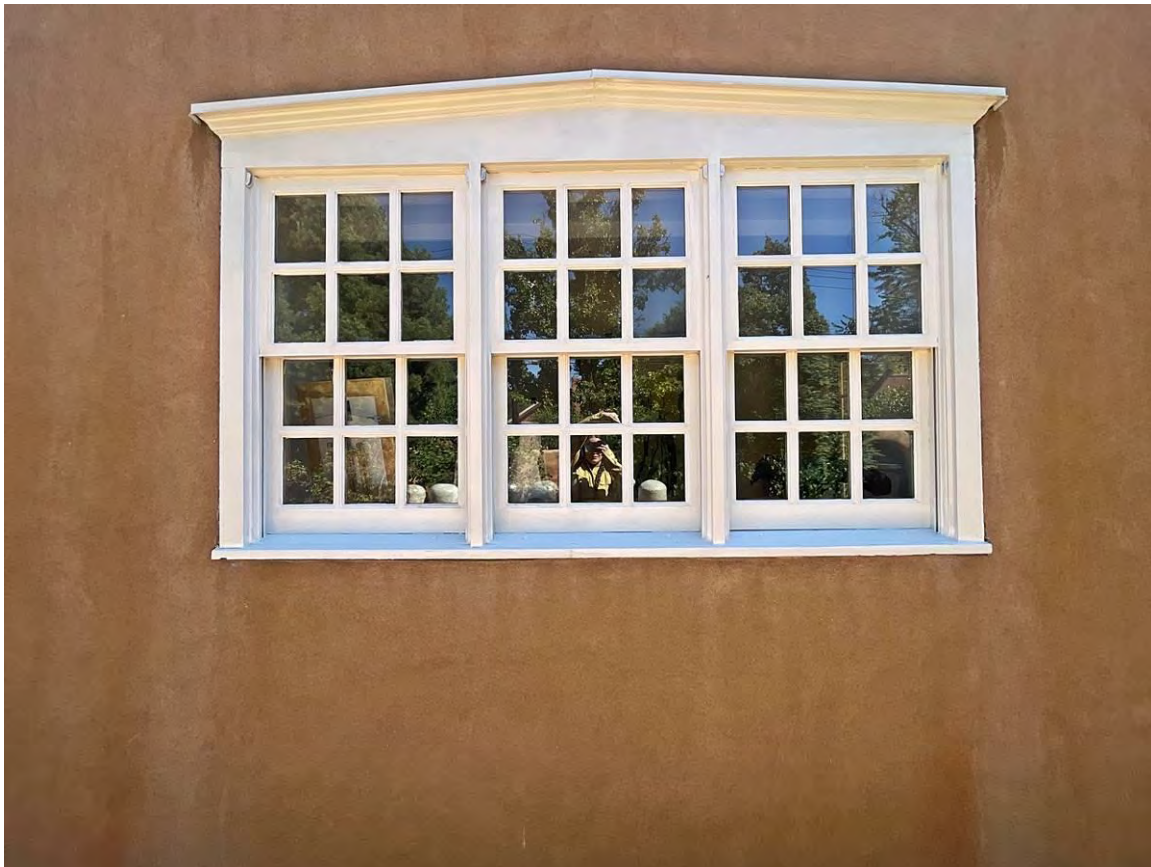
Photo 8: West elevation, detail of right (south) window. Camera facing east.
