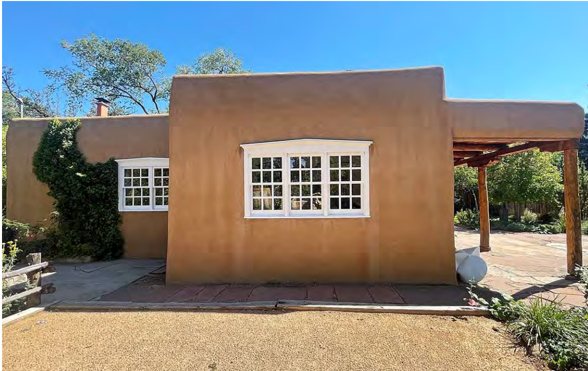
Photo 7: West elevation. Camera facing east.
