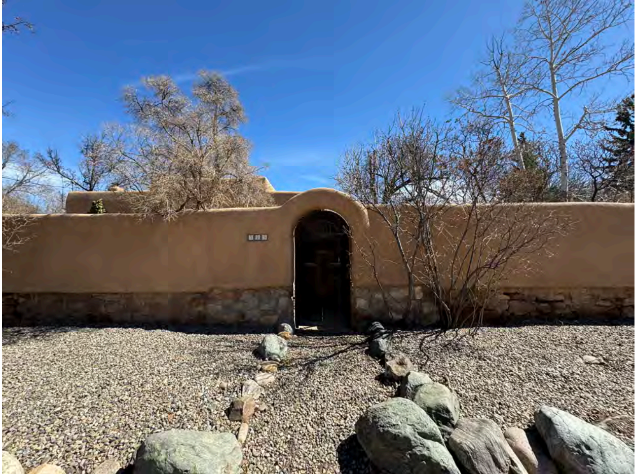
Pedestrian entrance facing west and Garcia Street, formally the car entrance. Notice different stone and grout pattern.
