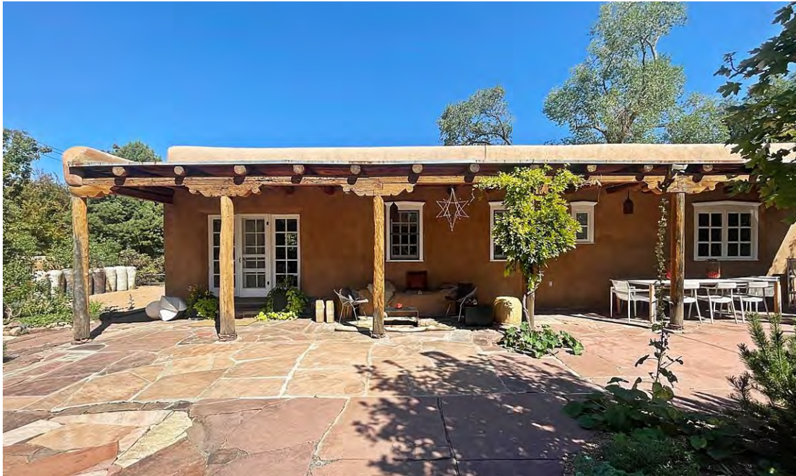
Photo 3: South elevation, west end. Camera facing north.
