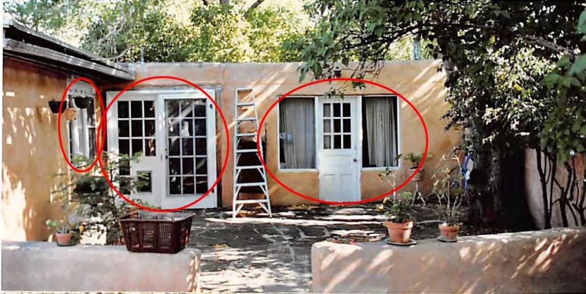
Figure 10: 1987 photograph of south elevation, primary bedroom suite. Circles indicate fenestration that was changed by new openings. Compare with Photos 5 & 6. Courtesy of City of Santa Fe Historic Preservation Division.
