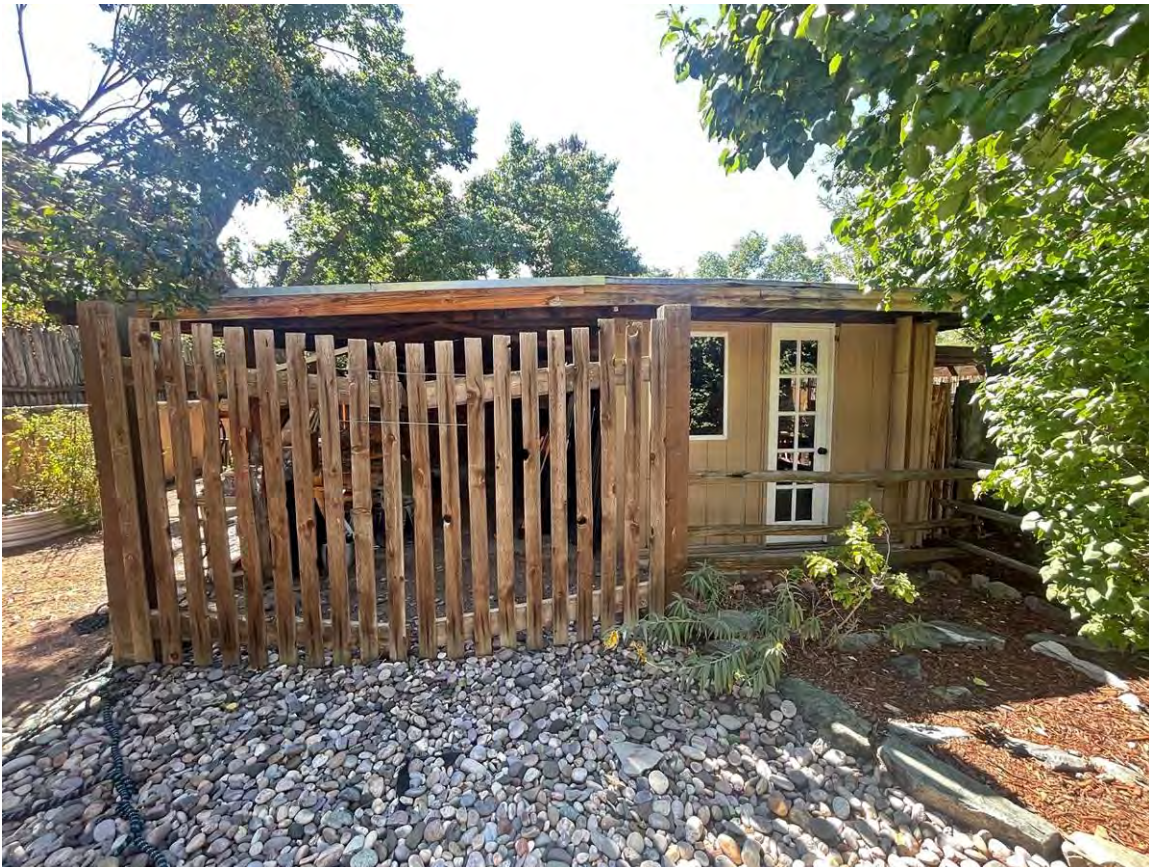
Photo 14: Guesthouse, north elevation. Camera facing south.
