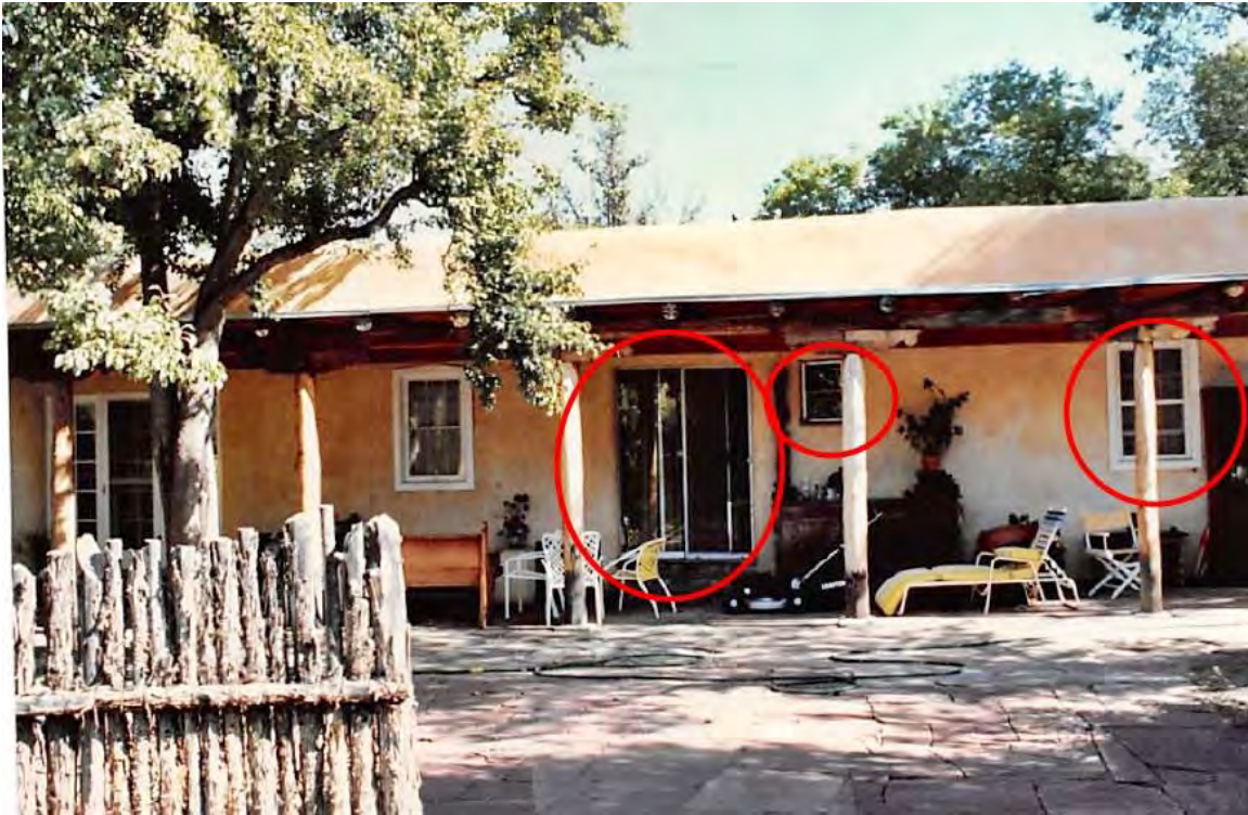
Figure 9: 1987 photograph of south elevation. Circles indicate fenestration that was changed by either elimination or enlargement of opening. Compare with Photo 3. Courtesy of City of Santa Fe Historic Preservation Division.
