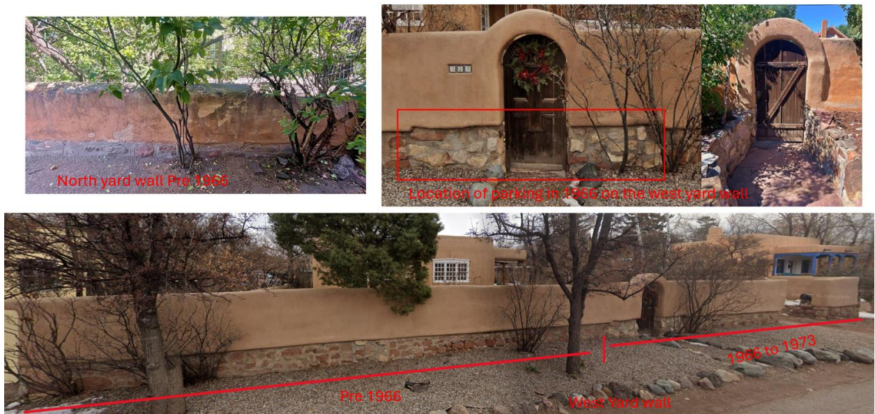
Figure 3: Yardwalls with construction dates
