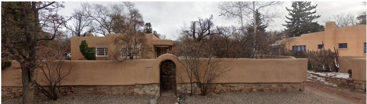
Figure 1: East elevation with front yard wall
