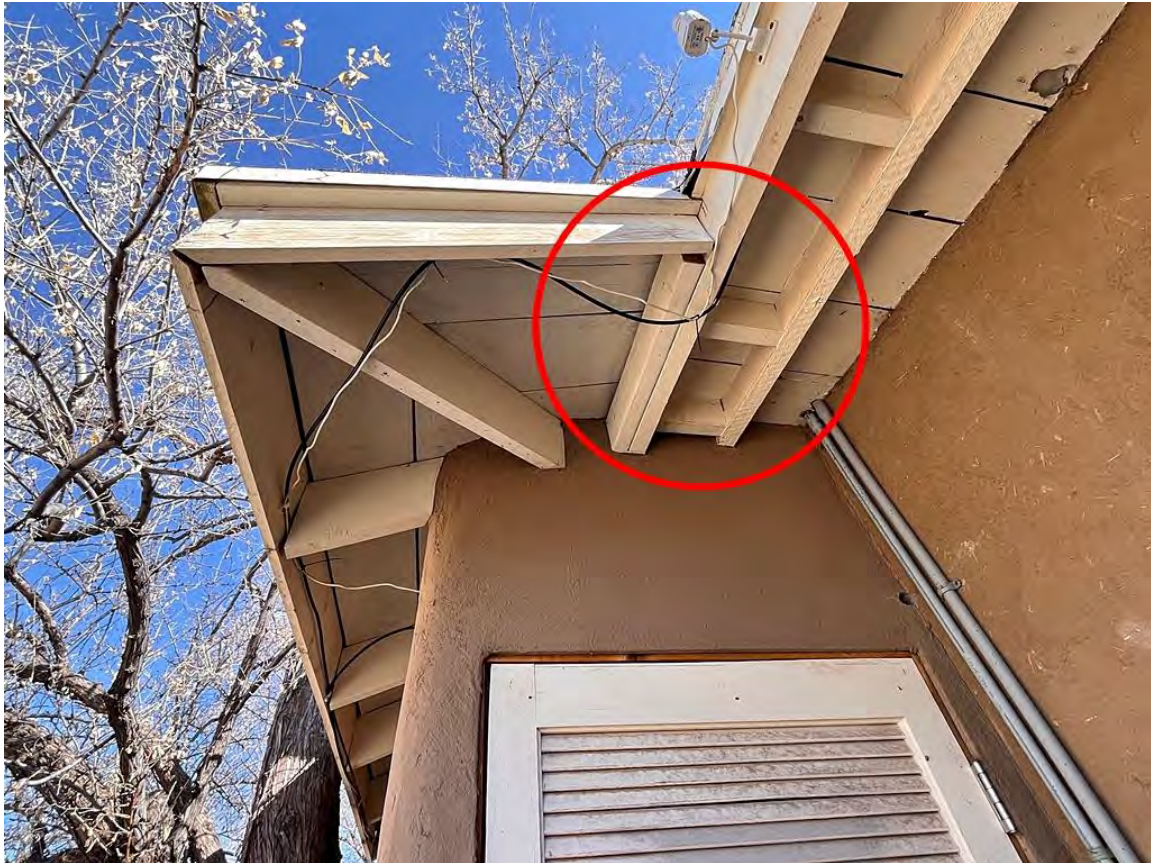
Photo 11: North elevation. Juncture of original building and porch. Camera facing up.
