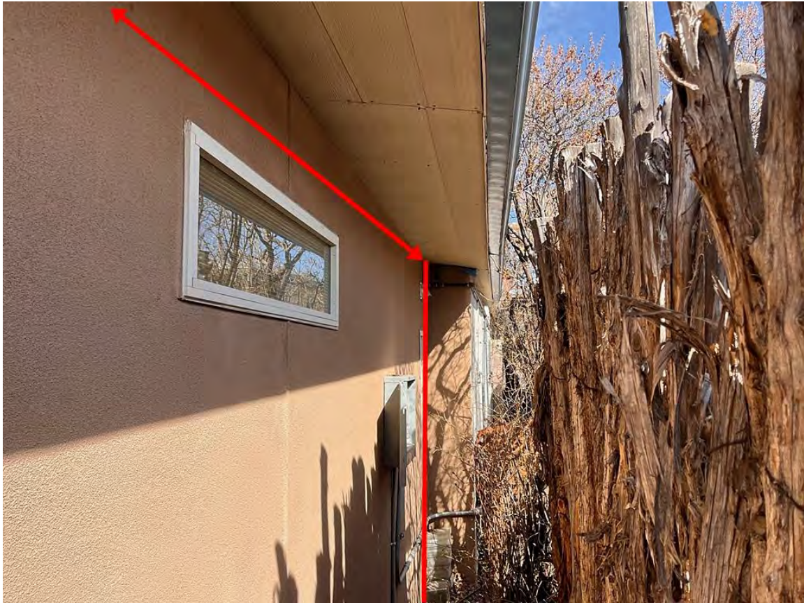
Photo 34: South elevation of extended carport. Camera facing east.
