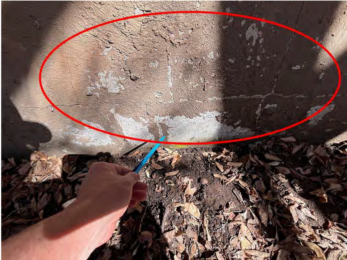
Photo 17: West elevation. CMU construction of post-1978 porch extension. Camera facing down.
