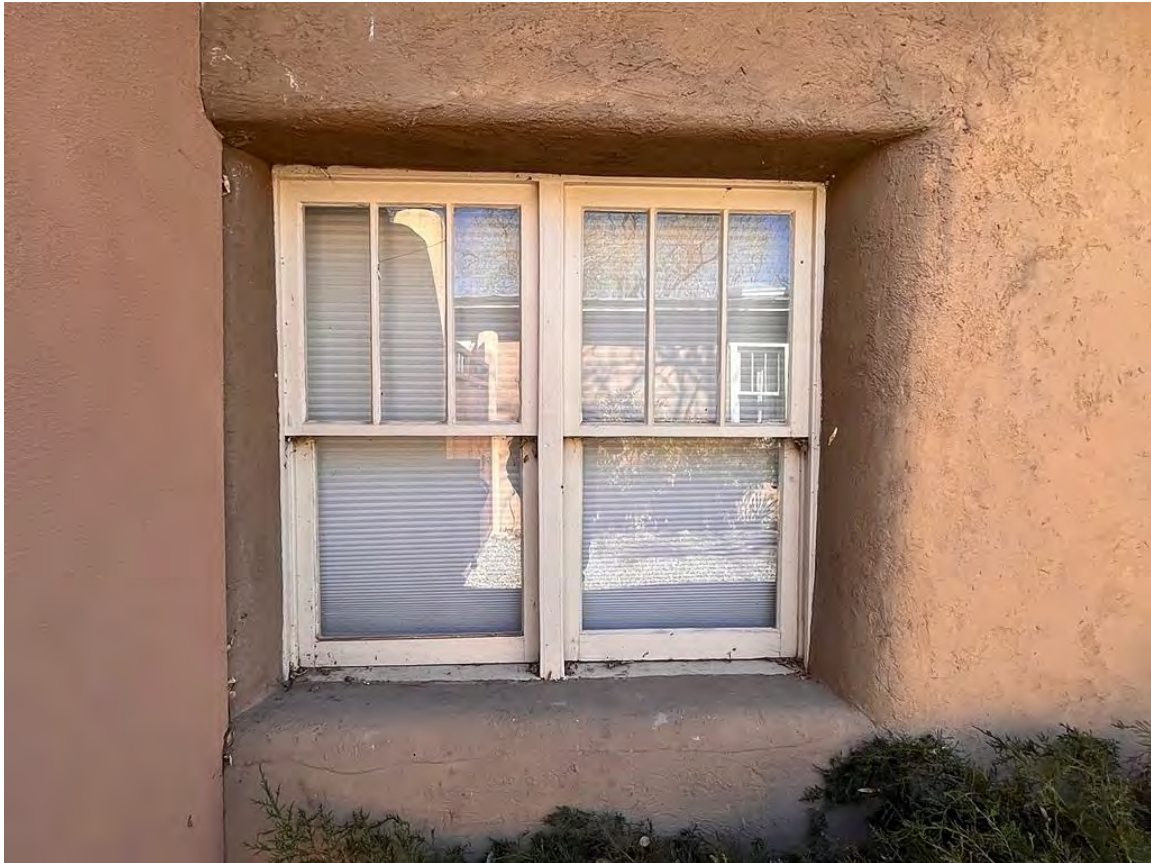
Photo 9: North elevation of original building. Window detail. Camera facing south.
