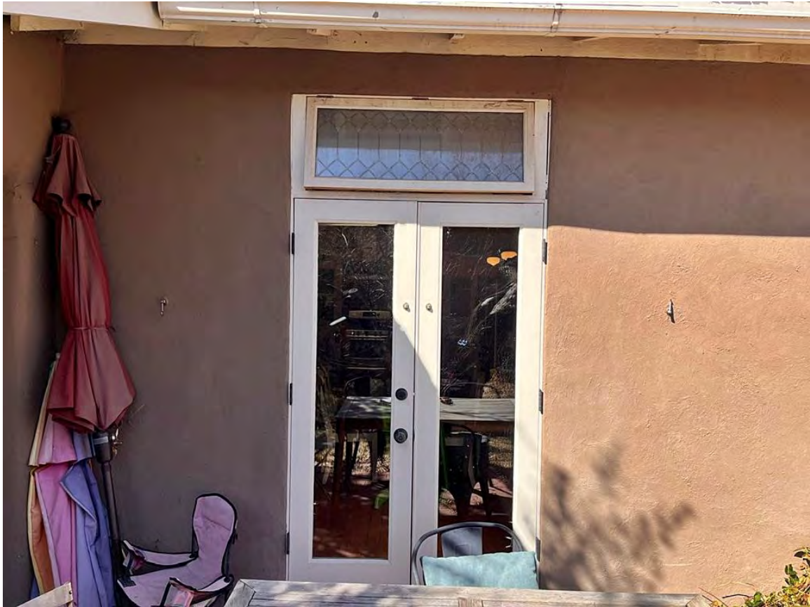
Photo 23: South elevation. Non-historic door. Camera facing north.
