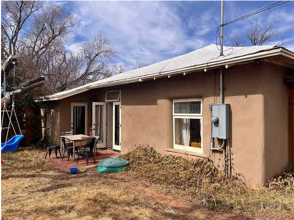
Photo 20: South elevation. Camera facing northwest.
