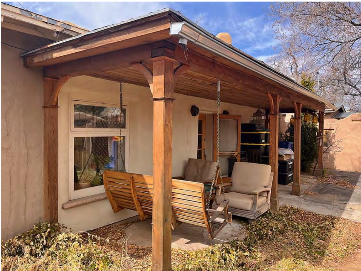
Photo 3: East elevation. Camera facing northwest.
