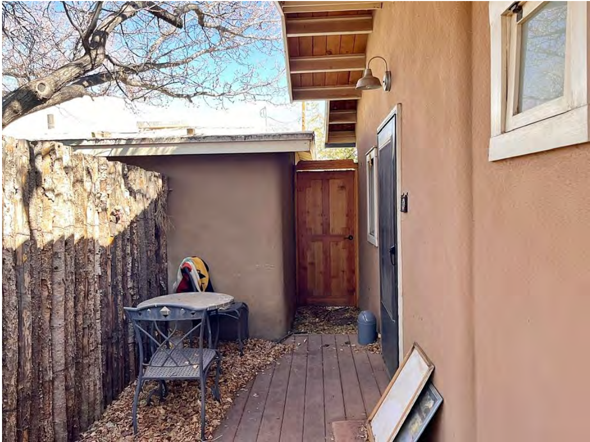
Photo 27: North elevation oblique, right. Camera facing east.
