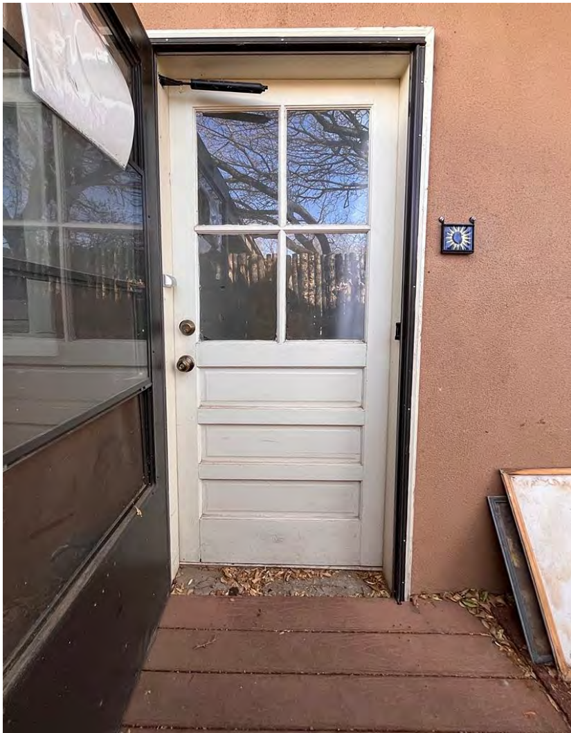
Photo 29: North elevation. Door detail. Camera facing south.
