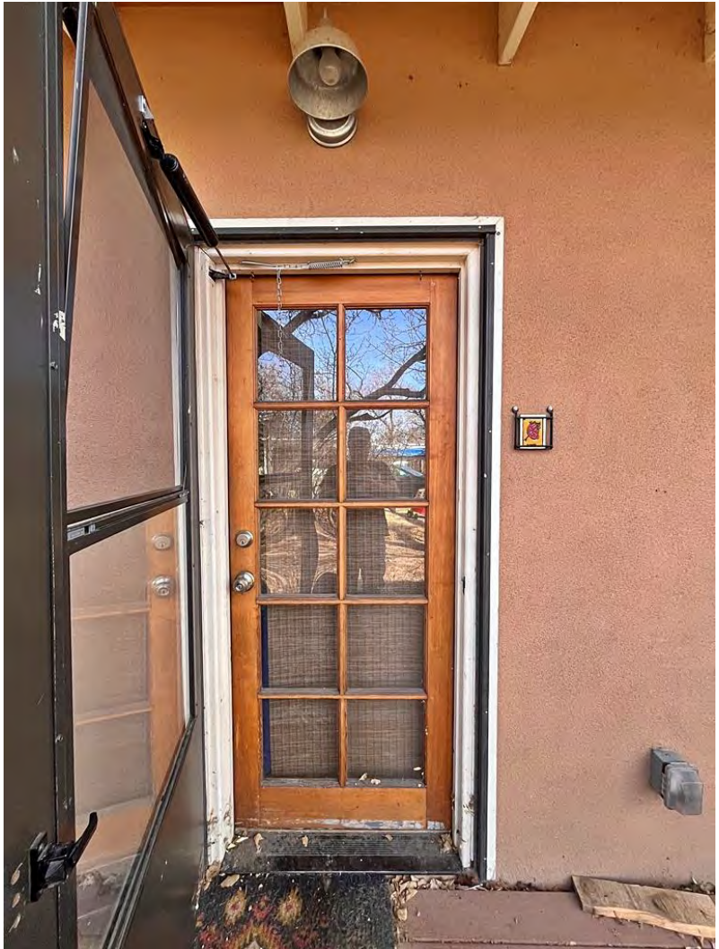
Photo 30: North elevation. Window detail. Camera facing south.
