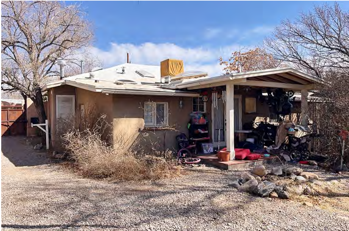
Photo 14: West elevation. Camera facing southeast.
