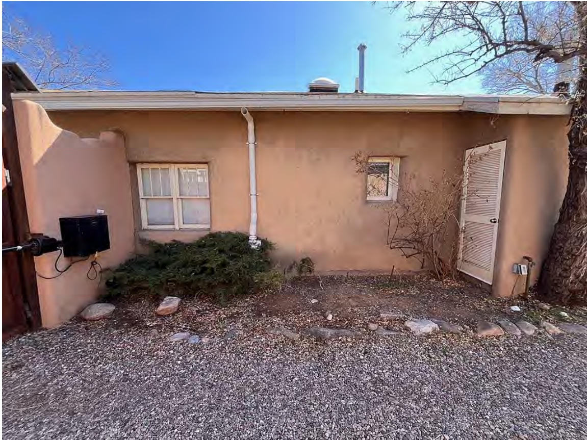
Photo 8: North elevation of original building. Camera facing south.
