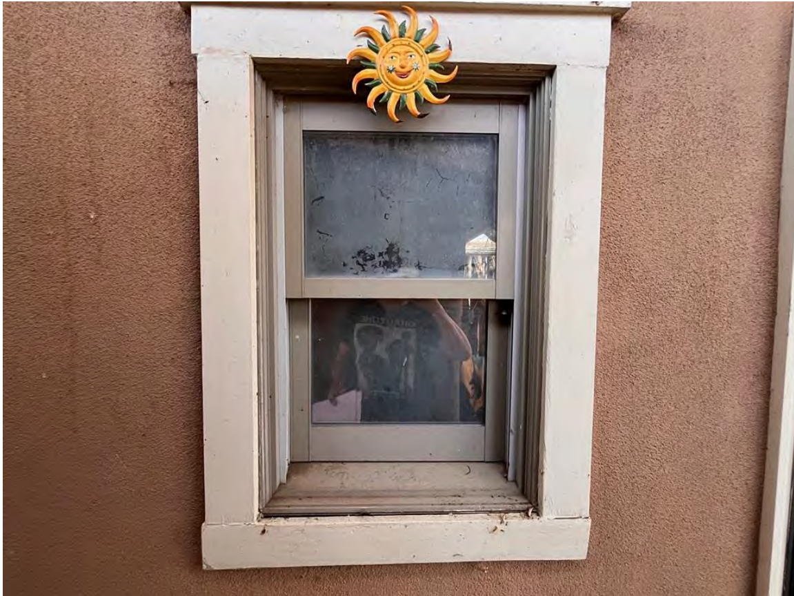
Photo 28: North elevation. Window detail. Camera facing south.
