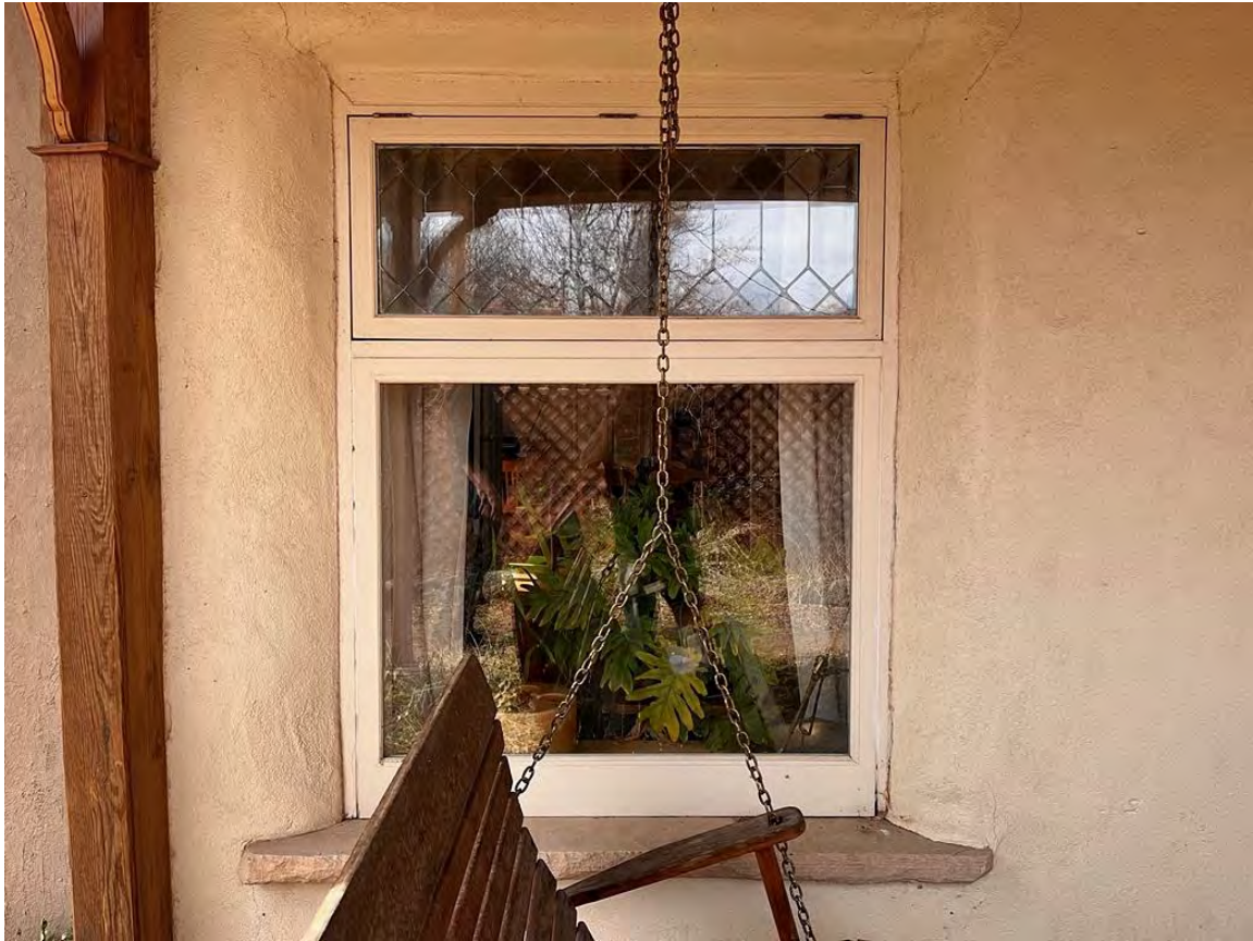
Photo 5: East elevation. South window. Camera facing west.
