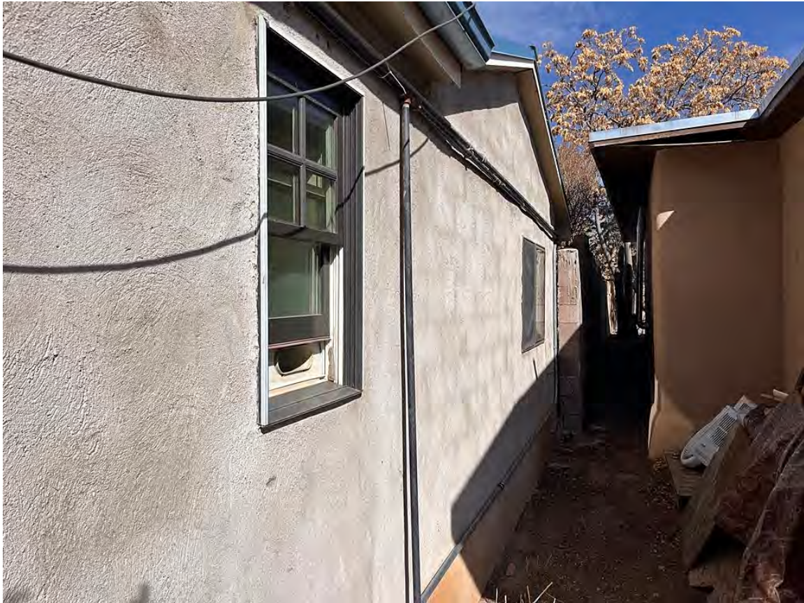
Photo 33: South elevation of ADU. Camera facing northeast.
