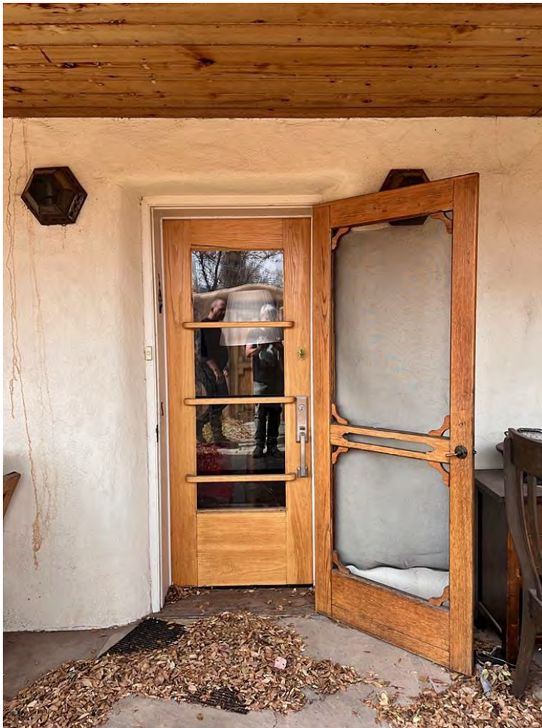
Photo 4: East elevation. Entry door. Camera facing west.
