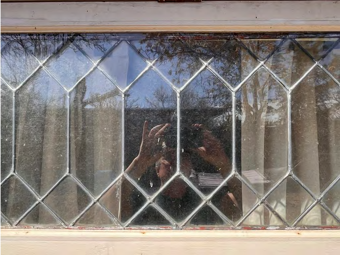
Photo 7: Detail of leaded lozenge pattern awning unit sash.
