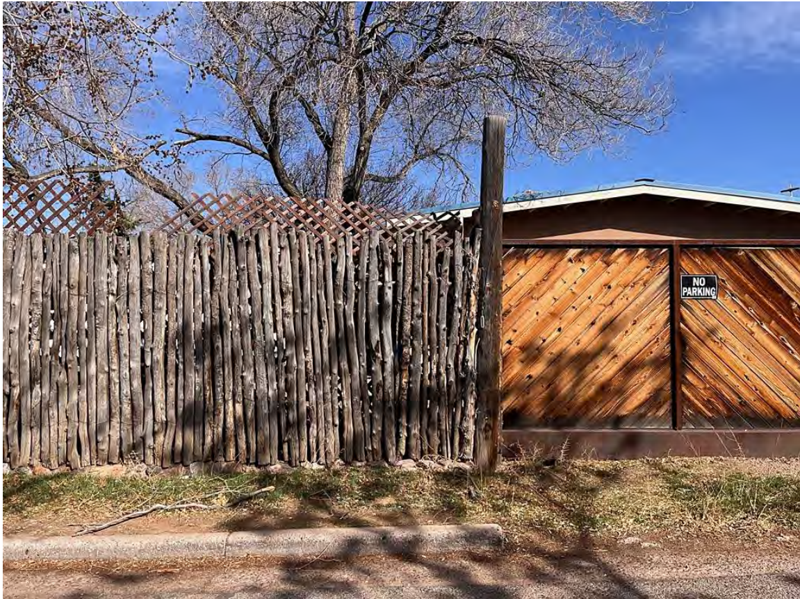
Photo 37: Latilla fence and gate along Ambrosio Street. Camera facing east.
