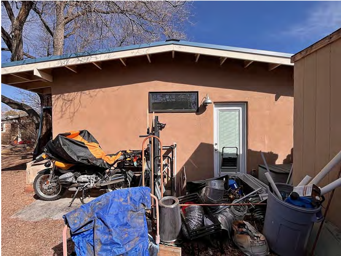
Photo 32: West elevation of extended carport. Camera facing east.
