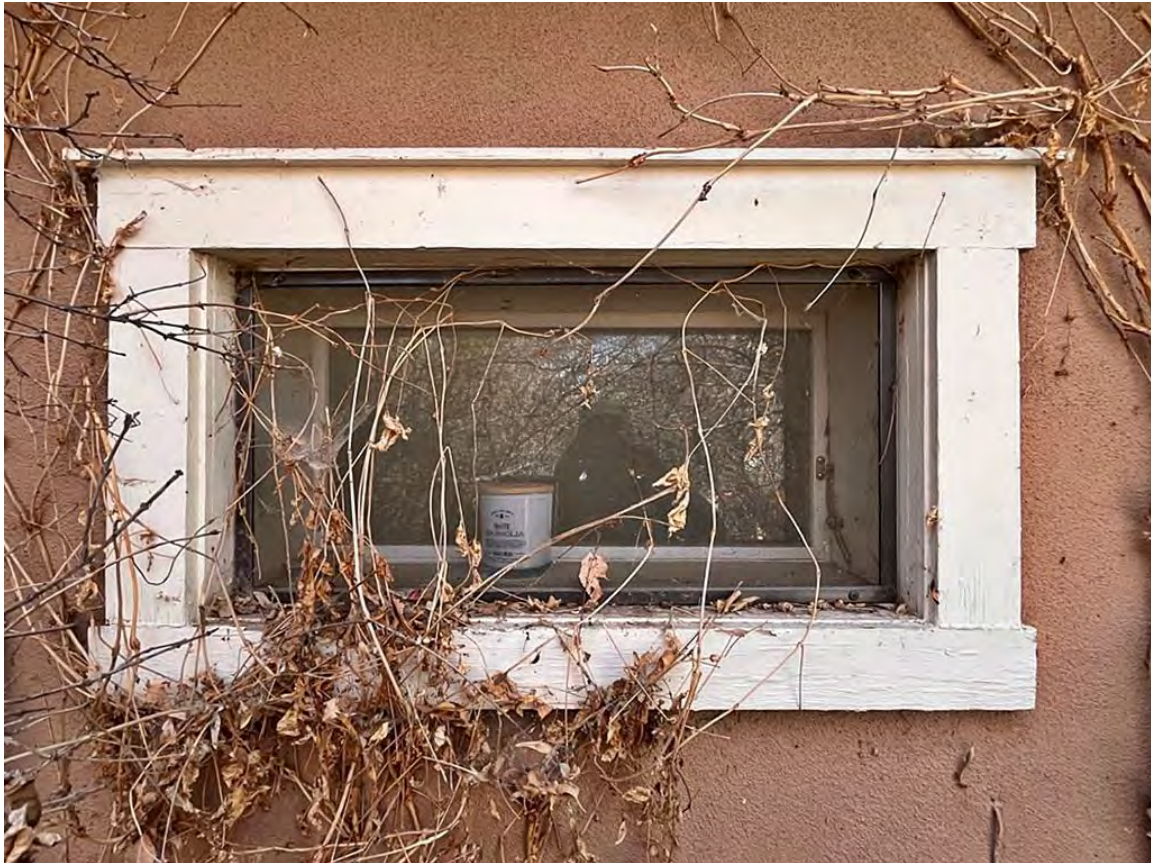
Photo 26: East elevation. Window detail. Camera facing west.
