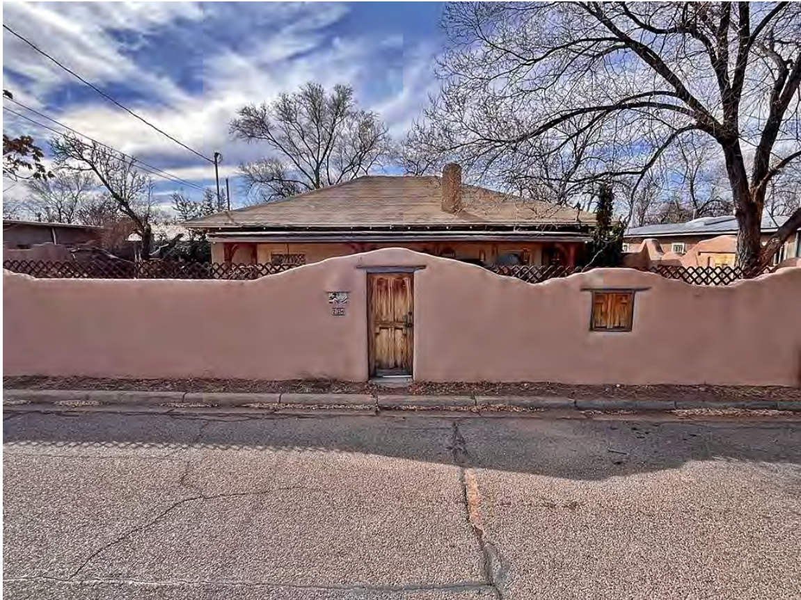
Photo 35: Street wall. Camera facing west. Photo taken with ladder.
