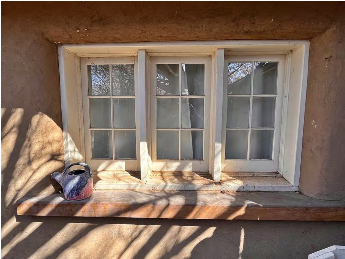
Photo 19: West elevation. Window detail of post-1978 porch extension. Camera facing east. Note exaggerated wood sill.
