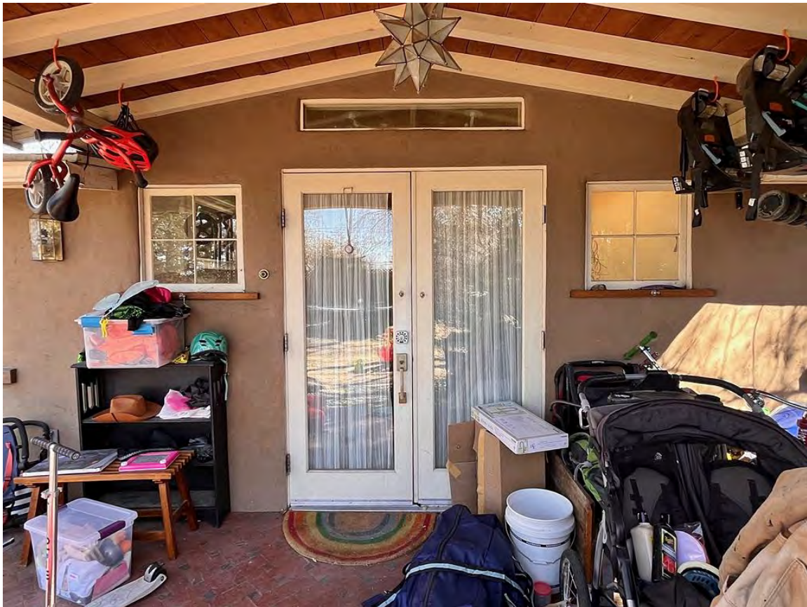
Photo 16: West elevation. Recent porch and mudroom. Camera facing east.
