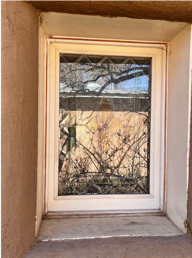
Photo 10: North elevation of original building. Window detail. Camera facing south.
