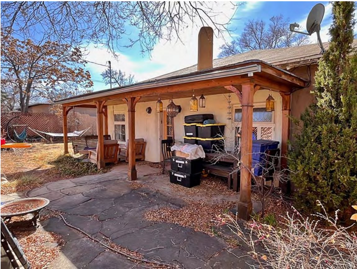
Photo 2: East elevation. Camera facing southwest.
