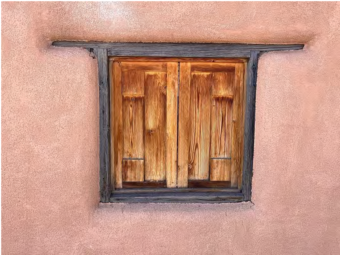
Photo 36: Street wall “window.” Camera facing west.
