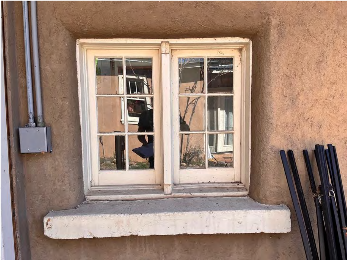
Photo 12: North elevation of enclosed porch. Window detail. Camera facing south.
