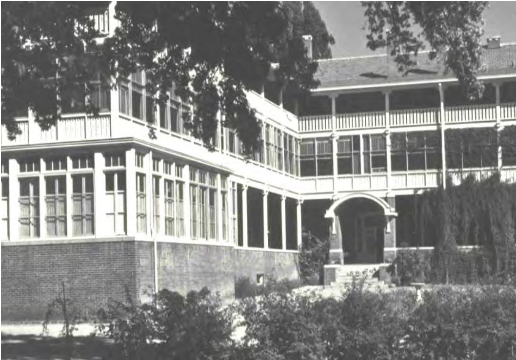
Exhibit 3. Marian Hall West Facade double-door entry, historic photo circa 1950
