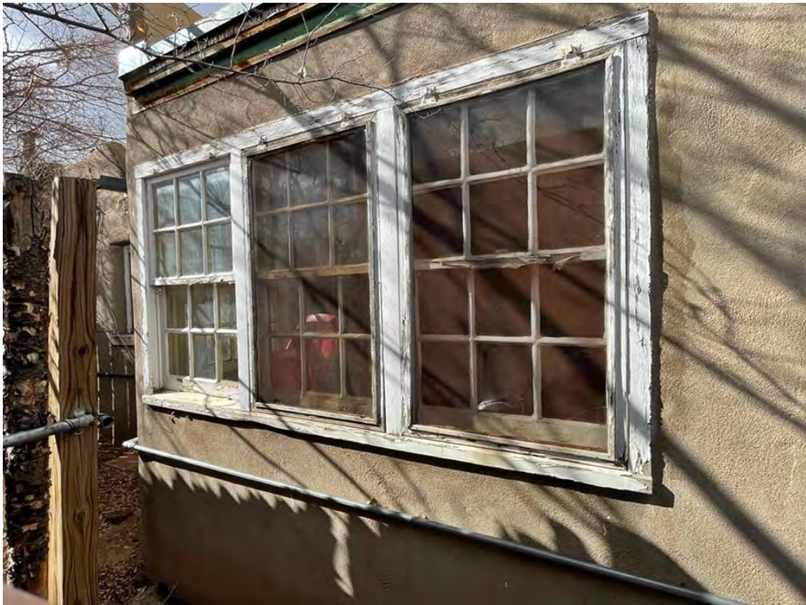
Photo 15: East elevation. Windows at the northeast corner. Camera facing west. Michael Zimmer, January 29, 2025.
