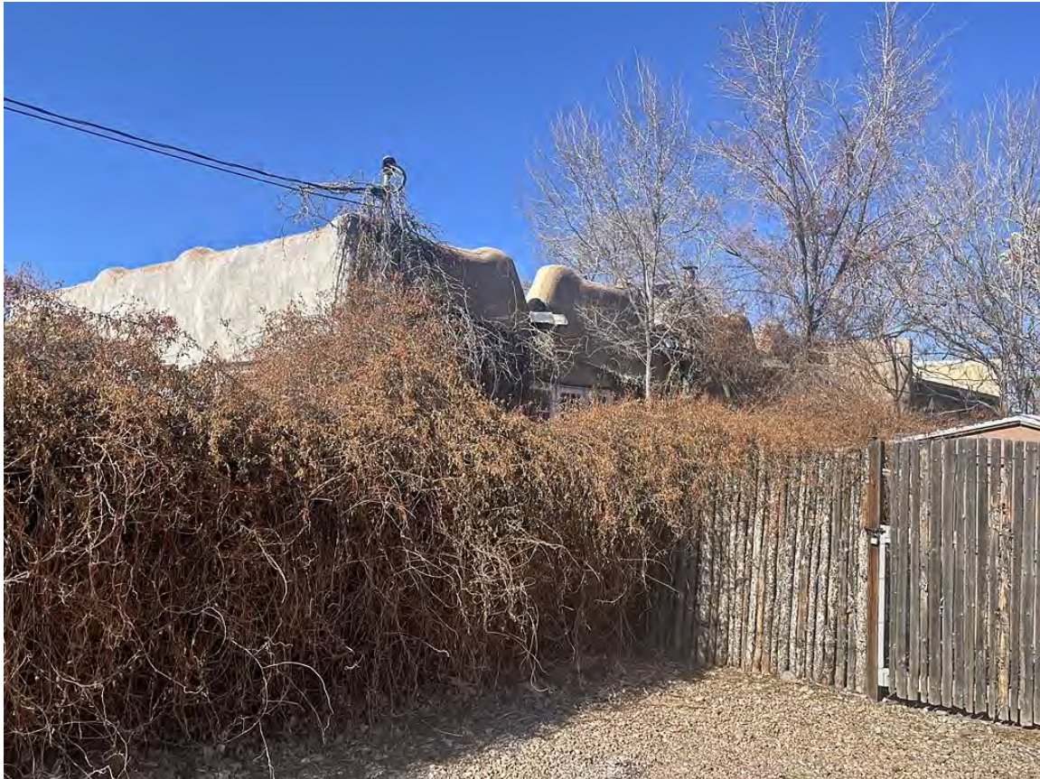
Photo 11: East elevation oblique. Camera facing northwest.
