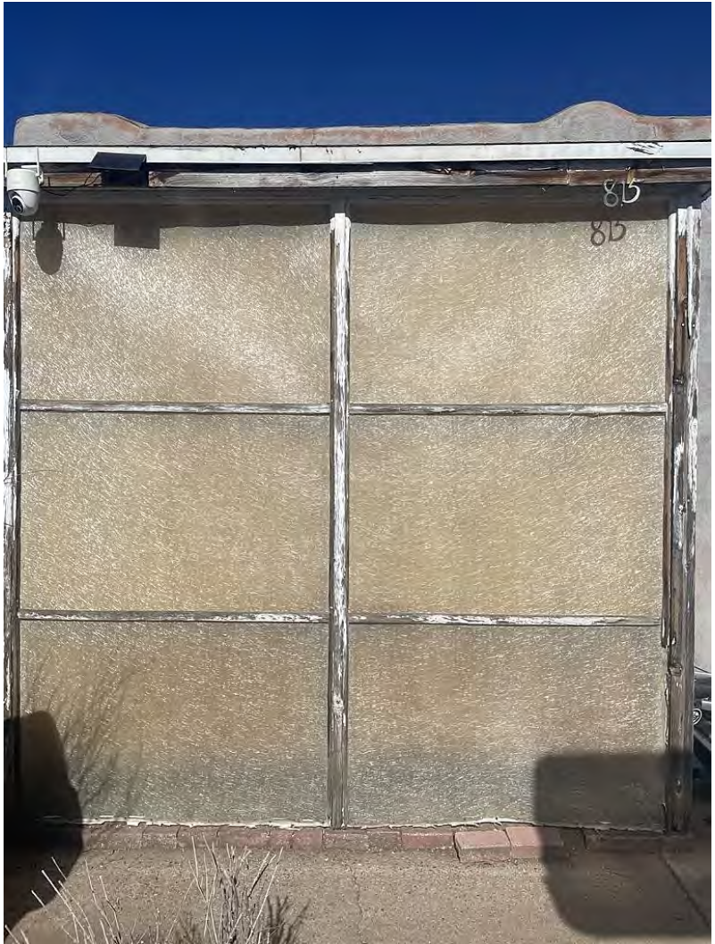
Photo 3: South (front) façade. Attached solar greenhouse. Camera facing north.
