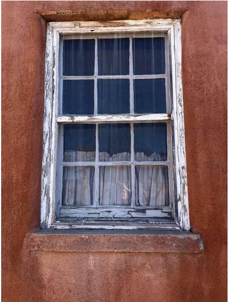
Photo 8: West elevation. Window detail. Camera facing east.
