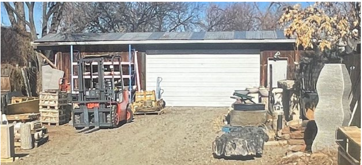
Figure 3: Garage Structure (photo courtesy of 2025 HCPI)
