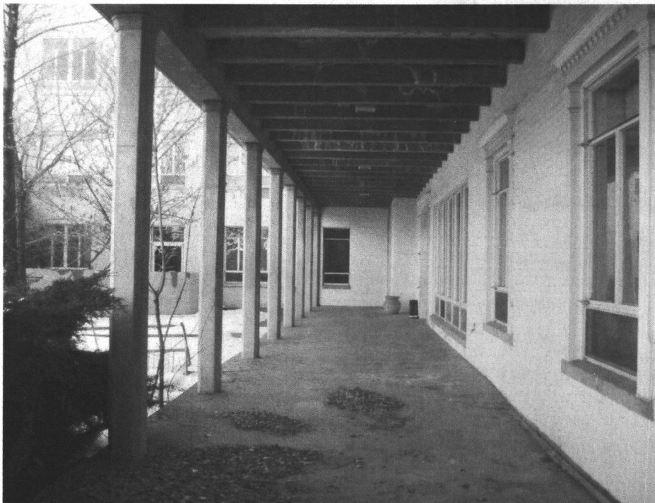
Figure 9: The entry portal at the entry off Palace. Note the chamfered capitals and columns, the natural concrete sills on the Windows (a detail found throughout the building), and the classical detail topping the windows.
