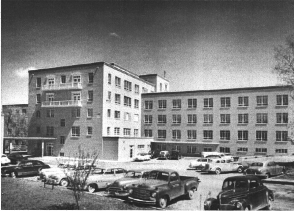
Figure 16: A 1950's view of the South wing with classical details on the upper floors that unify this elevation. Note the canopy connecting the Boiler Building now also serves as pipe rack for the steam heating system.
