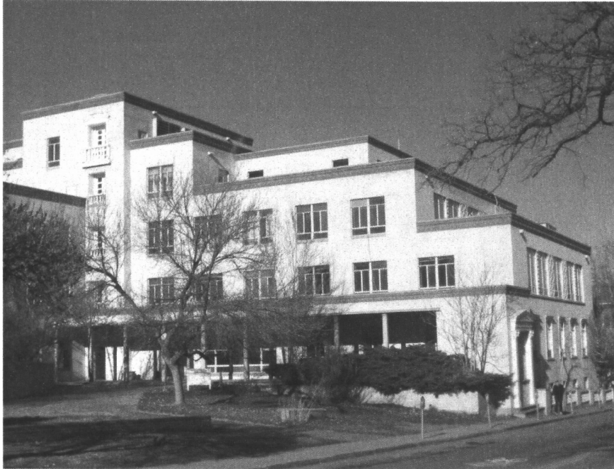
Figure 6: The Northeast corner of the North wing at Palace Avenue. These are the two primary facades of this building. Note the detail of the windows on the North façade, the decorative capitals at the now bricked in portal entry, the natural concrete columns at the portal leading to the main entry that faced the former parking lot/drop-off. Note the absence of the sign (See Figure 22) that used to be on the east wall, the missing cross at the top of the bricked up portal entrance pediment and the missing cruciform on top of the tower element.
