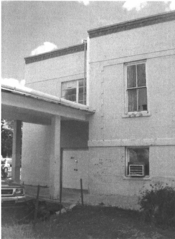
Figure 35: Connection of Meem design and original boiler building with canopy/pipe rack that connects to the hospital structure.
