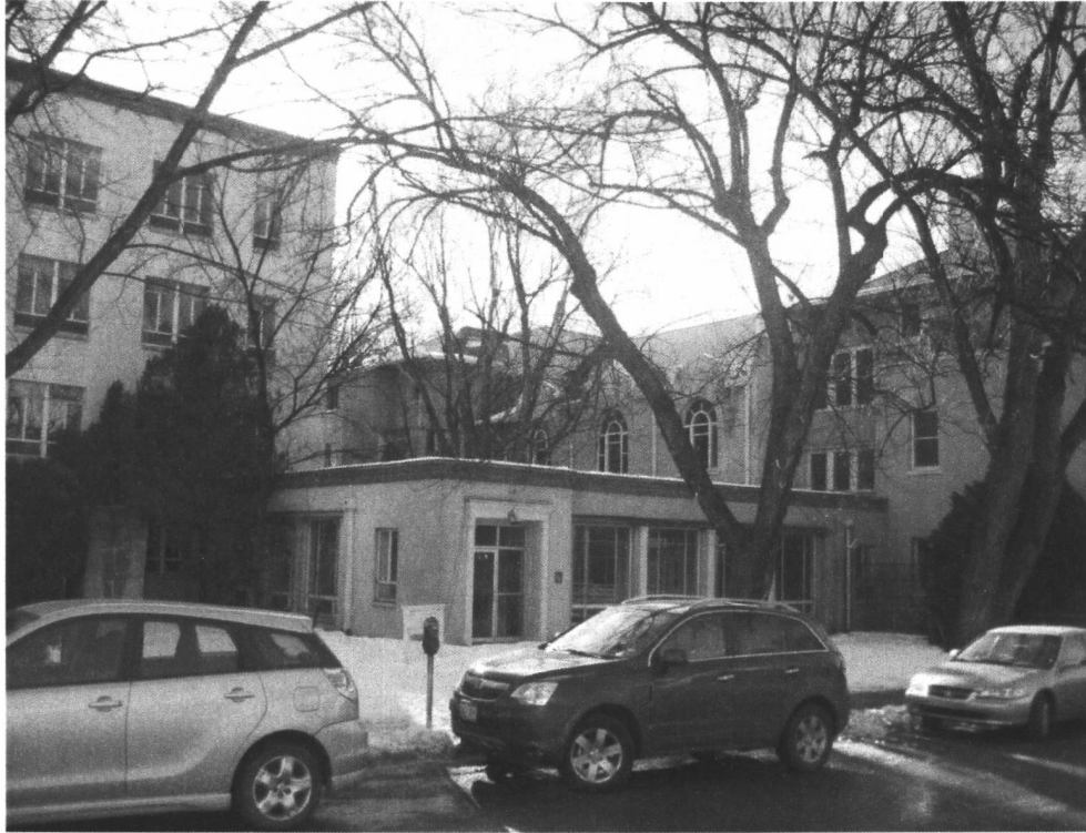
Figure 14: The connection to Marian Hall on Palace Avenue. Is it a breezeway? ...a portal? ...a secondary entrance? ...an enclosed courtyard? This element does not seem to be architecturally clear or function as intended. Note there was a drop off here originally for ambulatory patients that remained until the late 70's. The connection effectively serves to obscure the elevation of Marian Hall (a significant structure) where the dining room and chapel window detailing is located.
