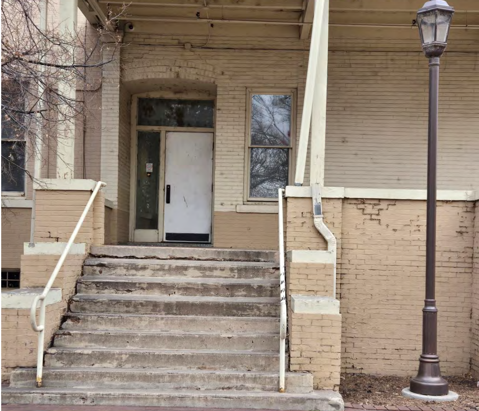
Marian Hall West Elevation Entry Door
