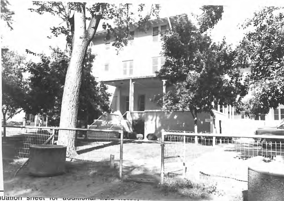
#35 west elevation, N end
