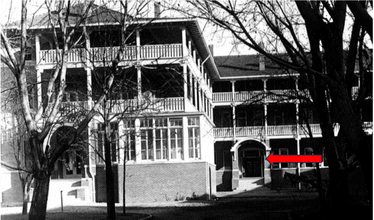
Figure 10: Photo circa 1950 showing the current window as a door
