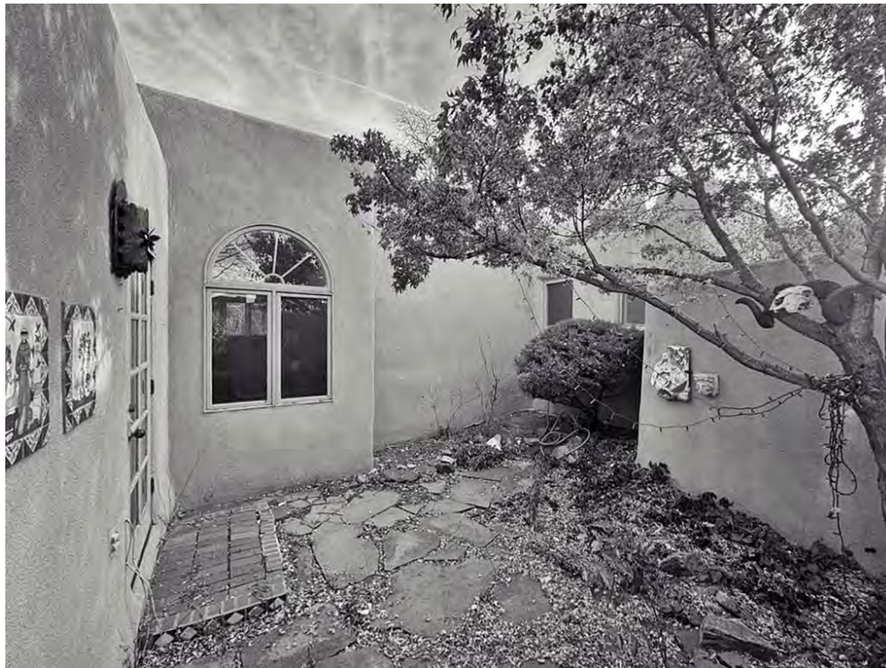
Photo 13: West elevation. Camera facing southeast. Gayla Bechtol, February 3, 2025.
