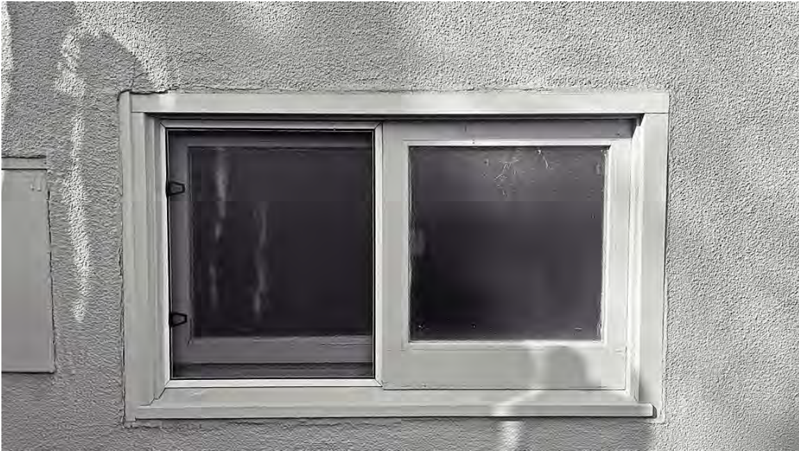
Photo 10: South elevation. Window detail. Camera facing northwest.
