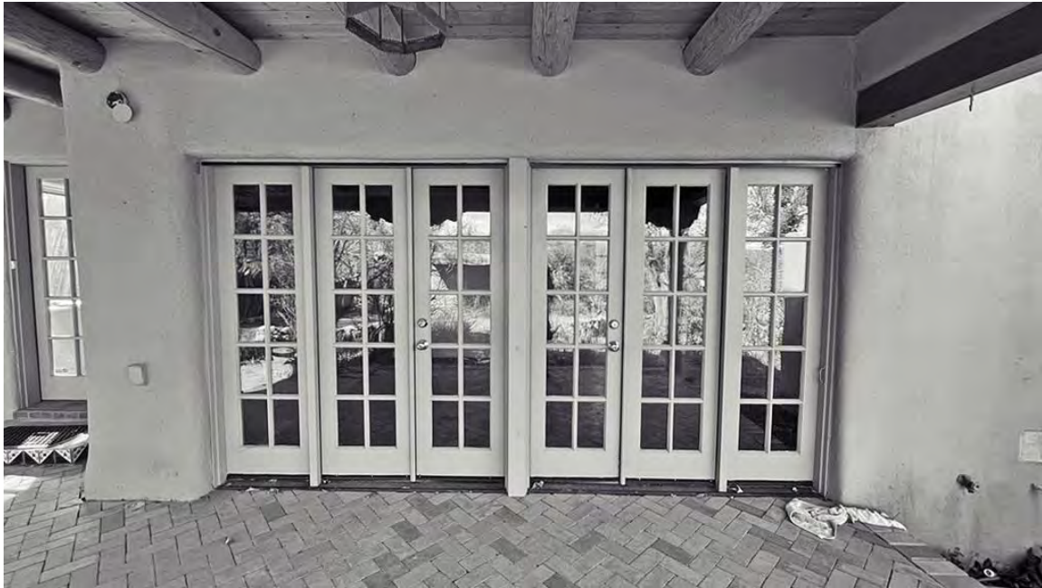
Photo 6: East elevation. Patio doors. Camera facing southwest.
