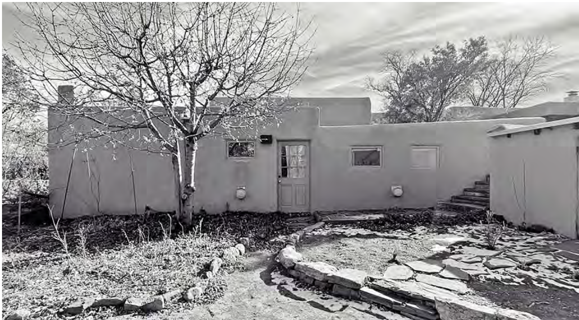
Photo 8: North elevation. Everything in view was constructed after 1992. Camera facing southeast.
