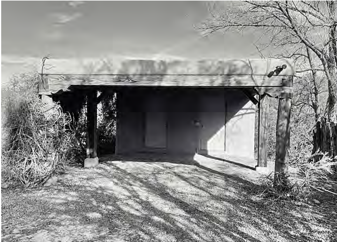
Photo 14: Carport and storage. This structure was built in 2003. Camera facing northeast.
