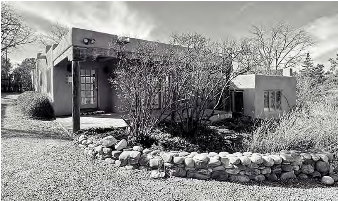
Photo 5: East (front) elevation. Everything in view was constructed after 1992. Camera facing southwest.
