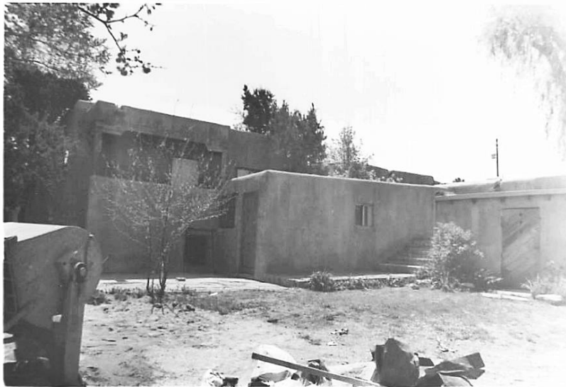
#14 north elevation, east portion
