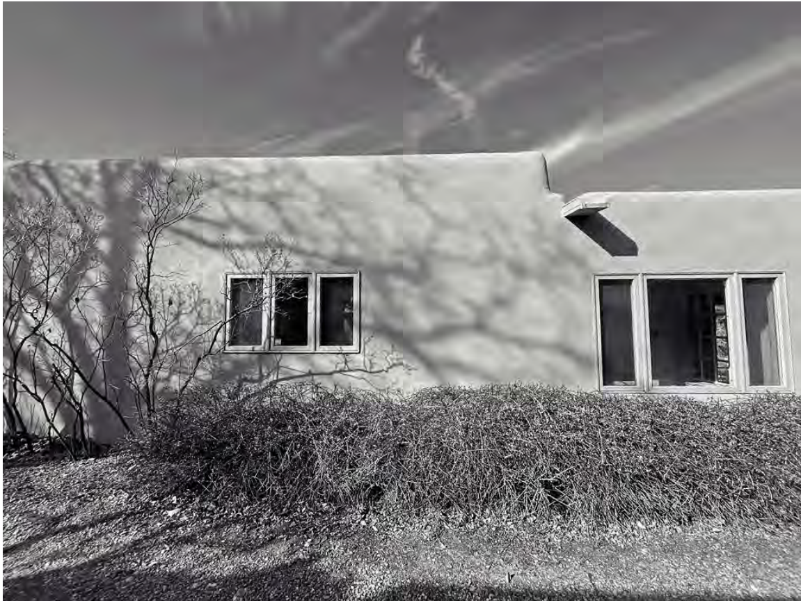
Photo 11: South elevation East section. Camera facing northwest.
