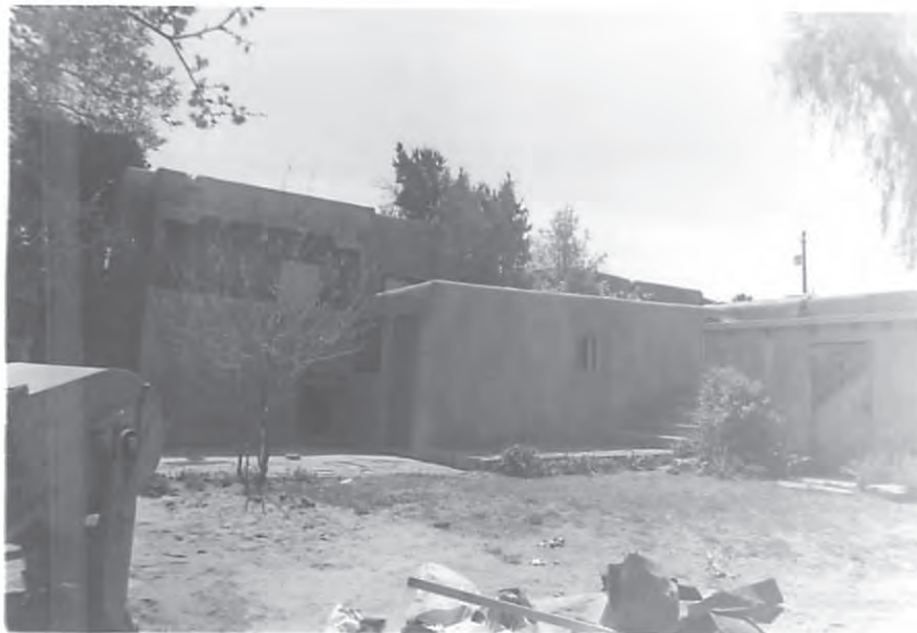
#14 north elevation, east portion
