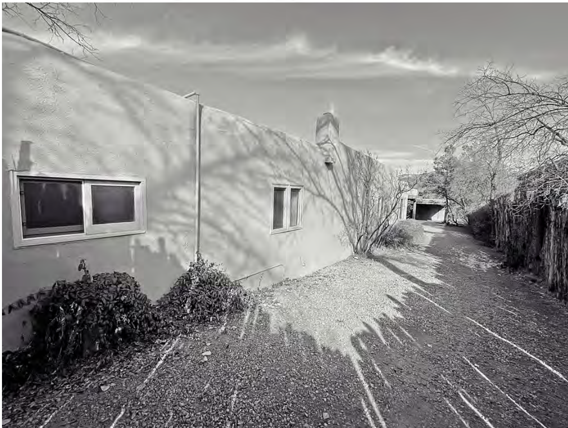
Photo 9: South elevation oblique. Camera facing northeast.
