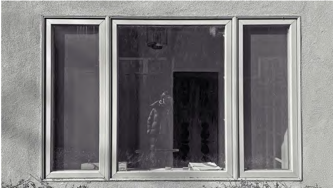
Photo 12: South elevation. Window detail. Camera facing northwest.
