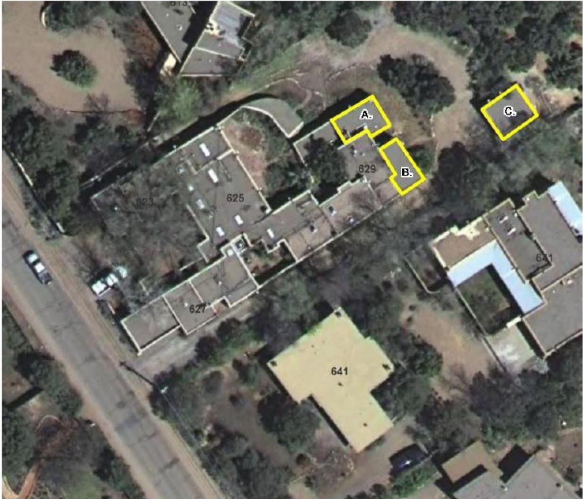
Figure 11: 2005 aerial photograph. Alterations since the 1992 HBI survey: A. bedroom built between 1992 and 2001; B. portal built in 2003; C. carport built in 2003.
