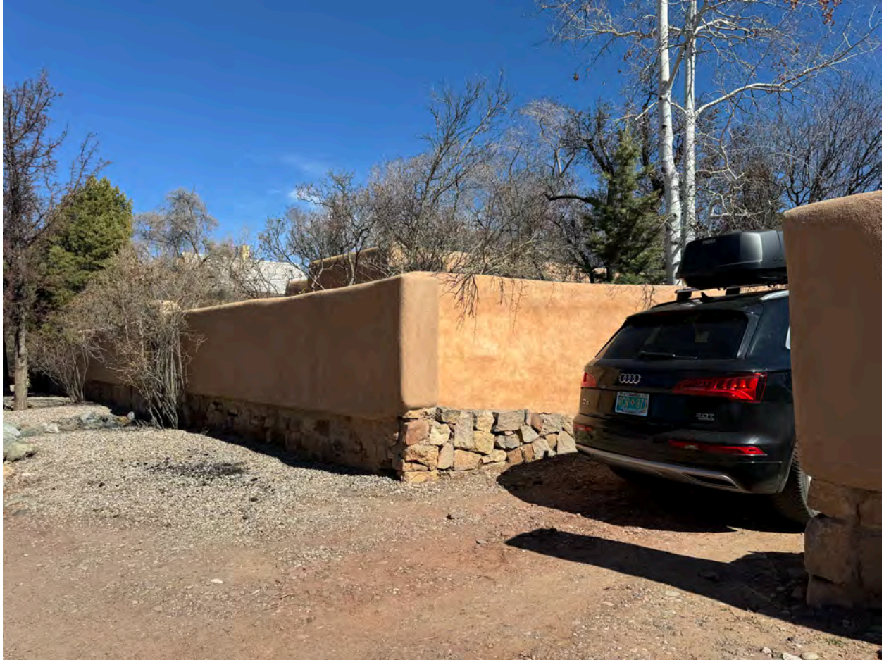
Photo of driveway entrance at wall. Notice different stone and stucco.
