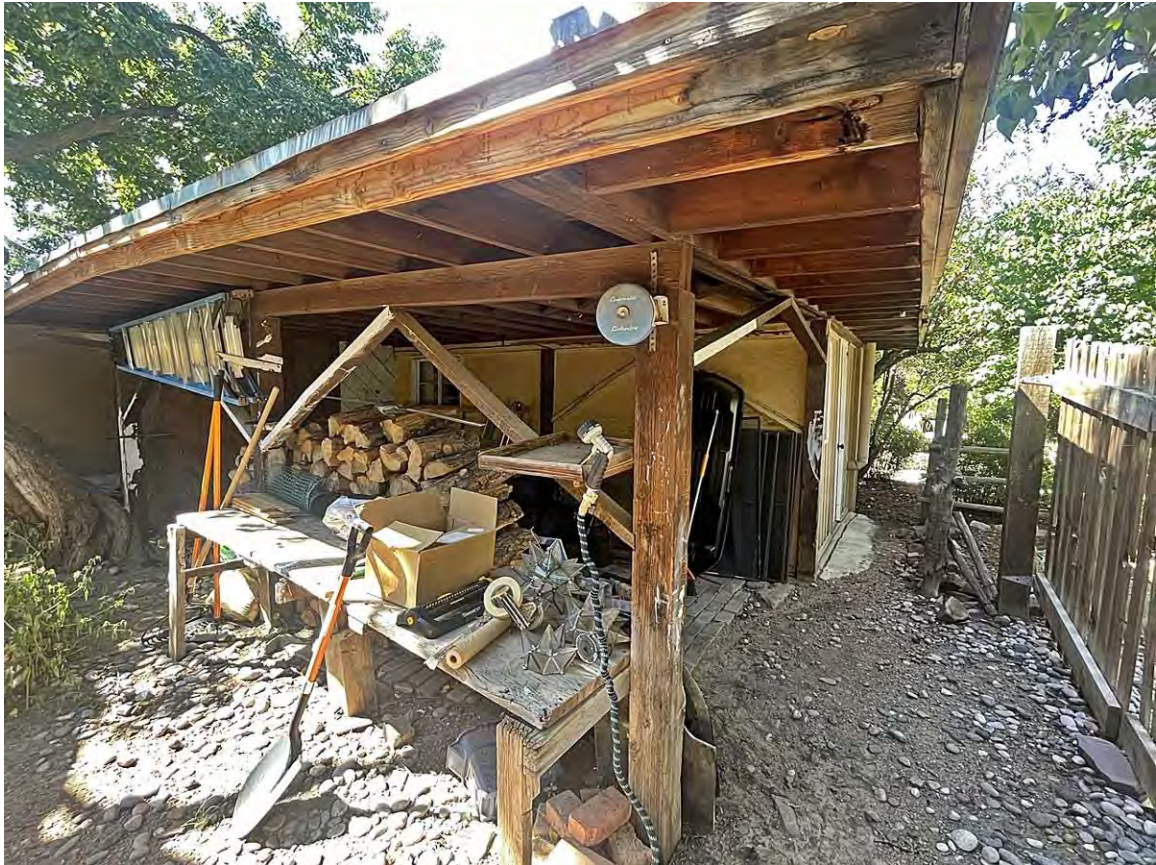
Photo 15: Former carport. Camera facing southeast.
