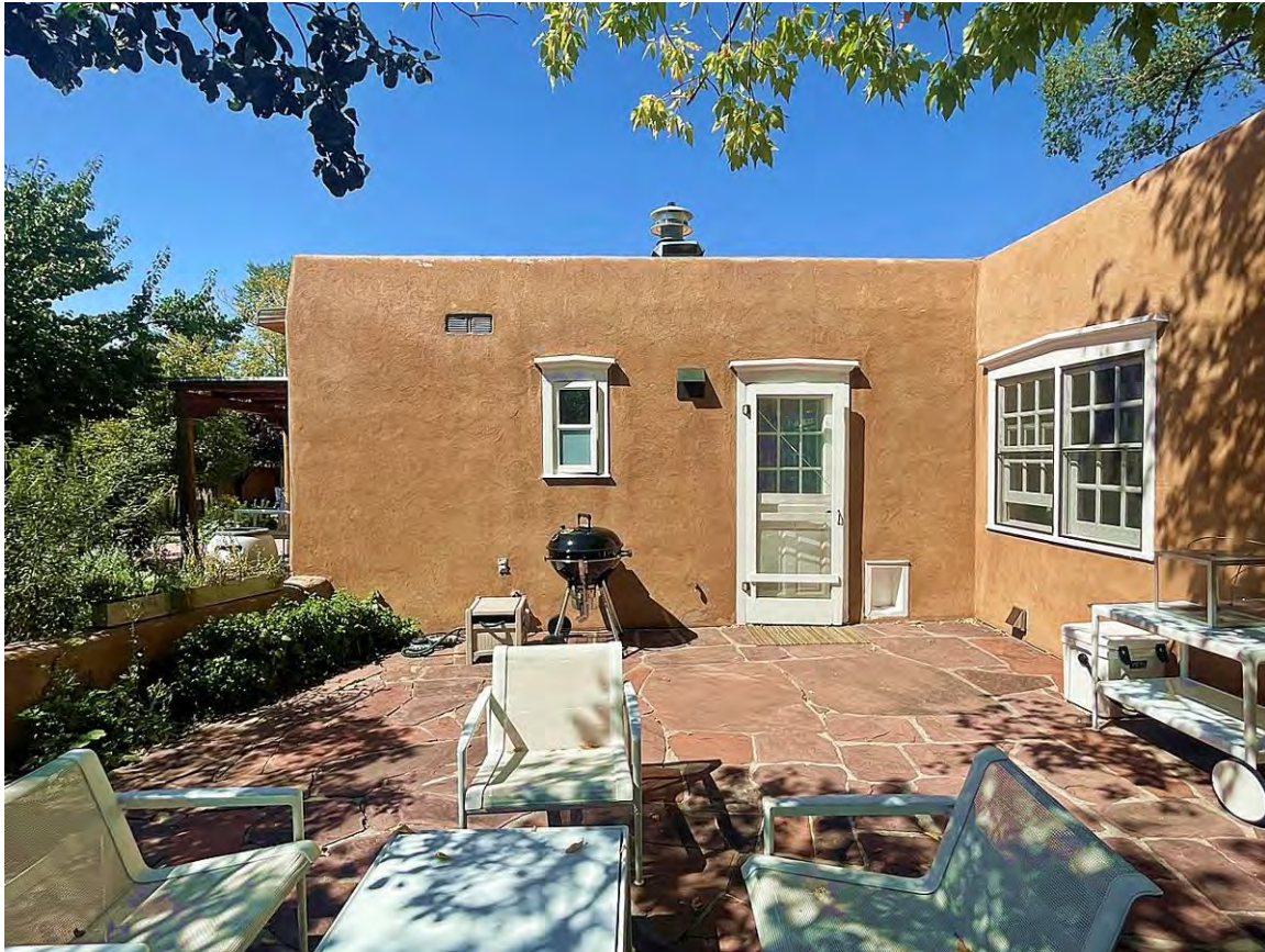
Photo 6: East elevation and presumed enclosed porch. Camera facing west.
