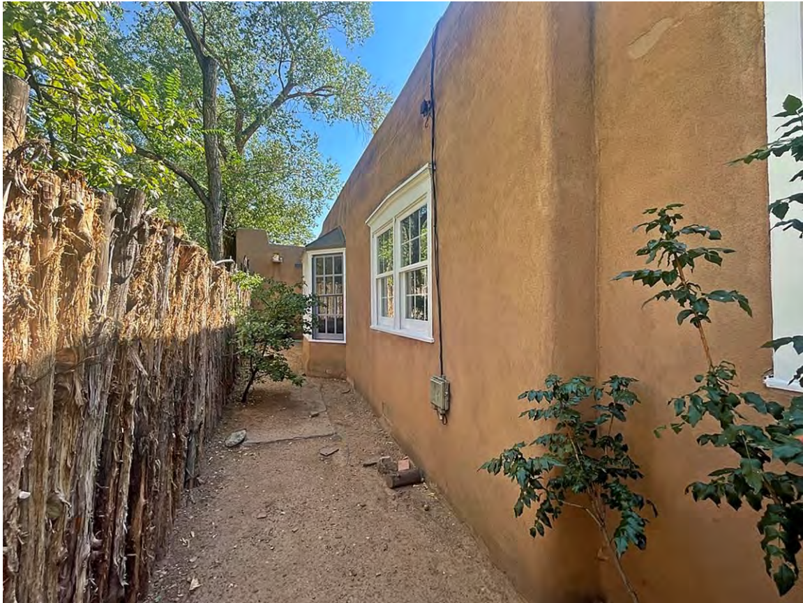
Photo 10: North elevation, bay window in distance. Camera facing southeast.
