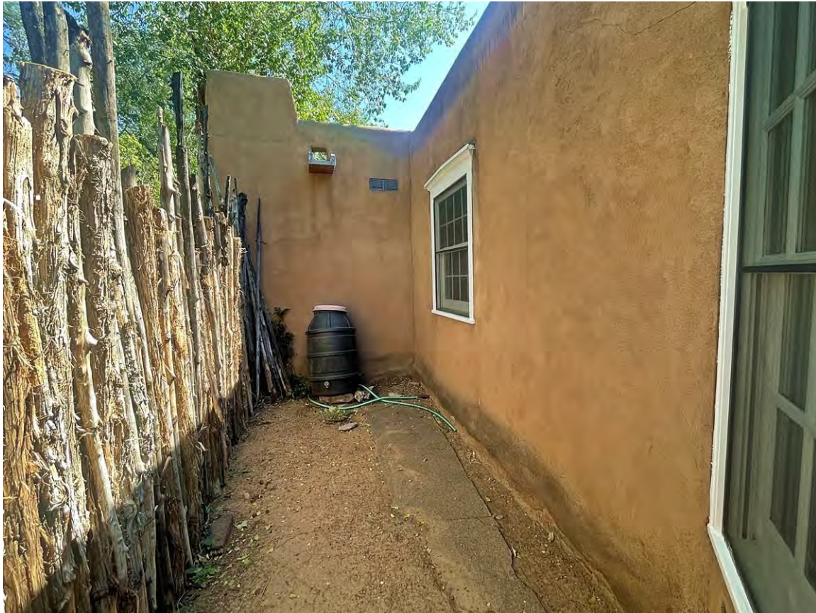
Photo 12: North elevation, east end. Camera facing southeast.
