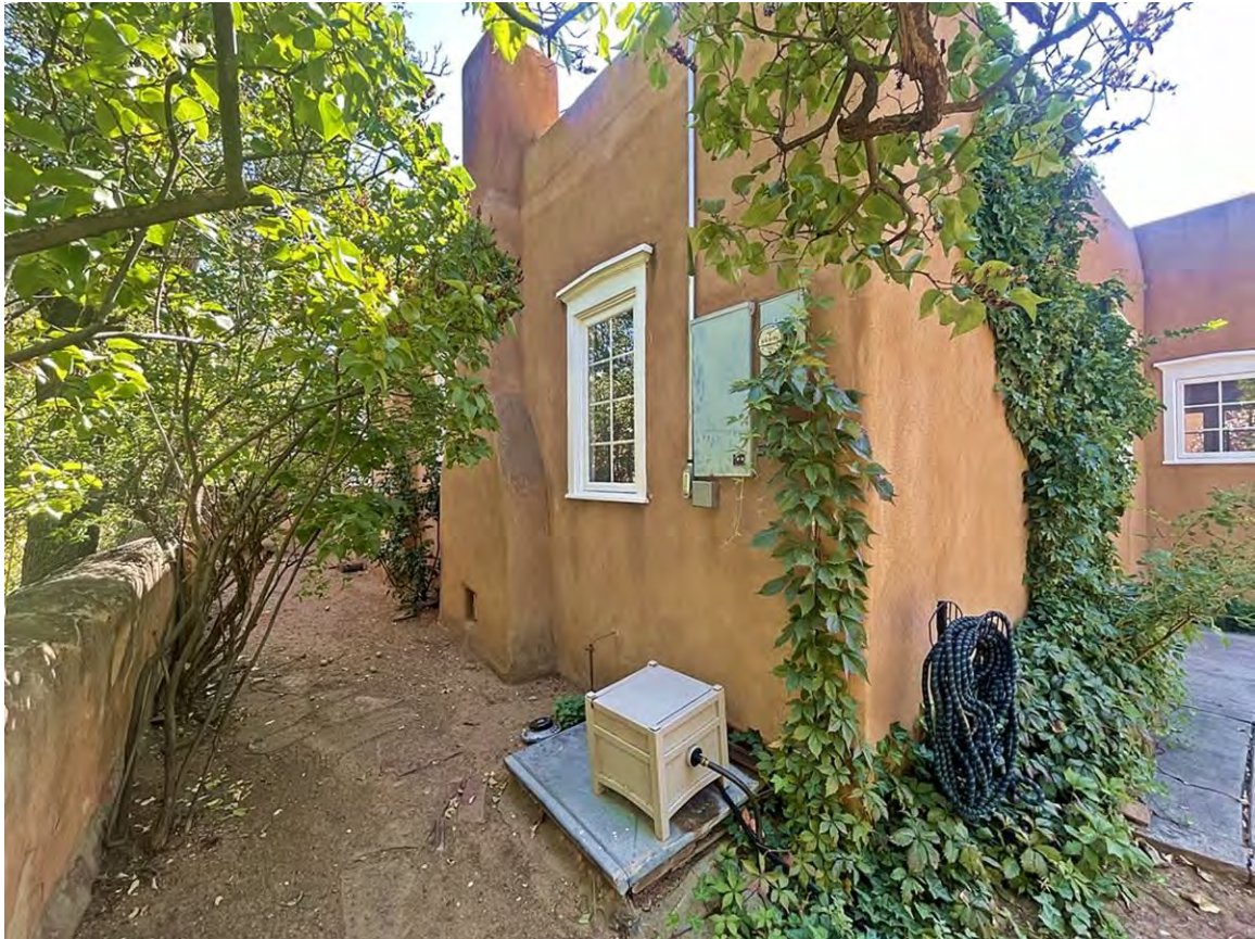
Photo 9: North elevation oblique. Camera facing southeast.
