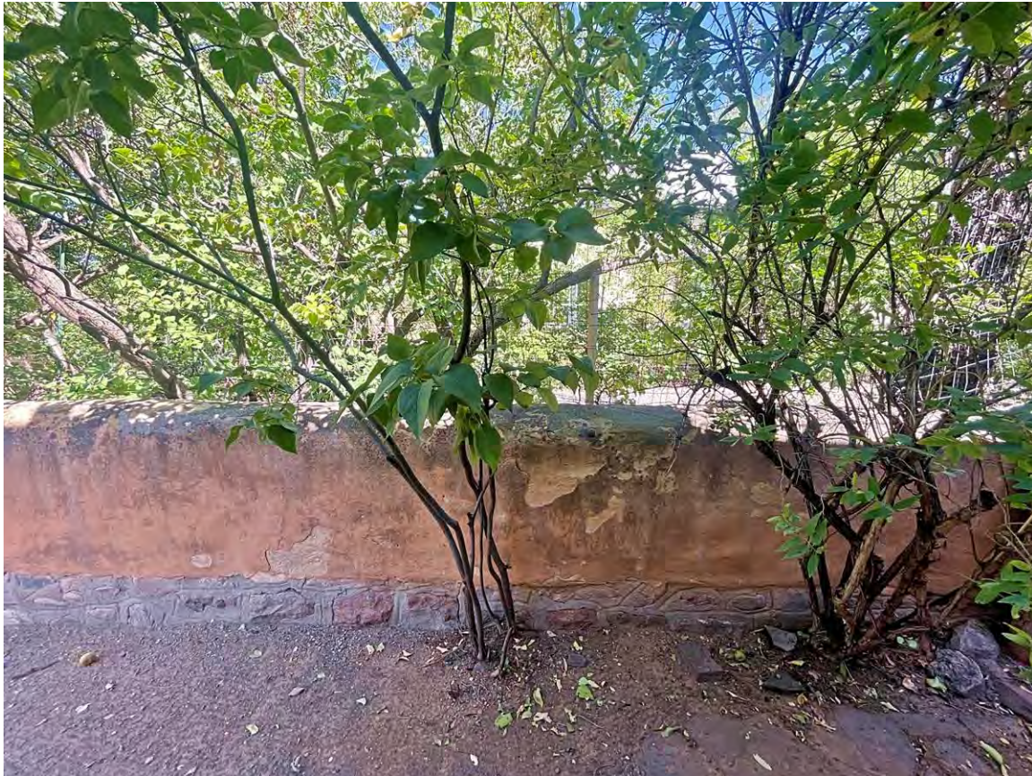
Photo 18: North property wall. Camera facing north.
