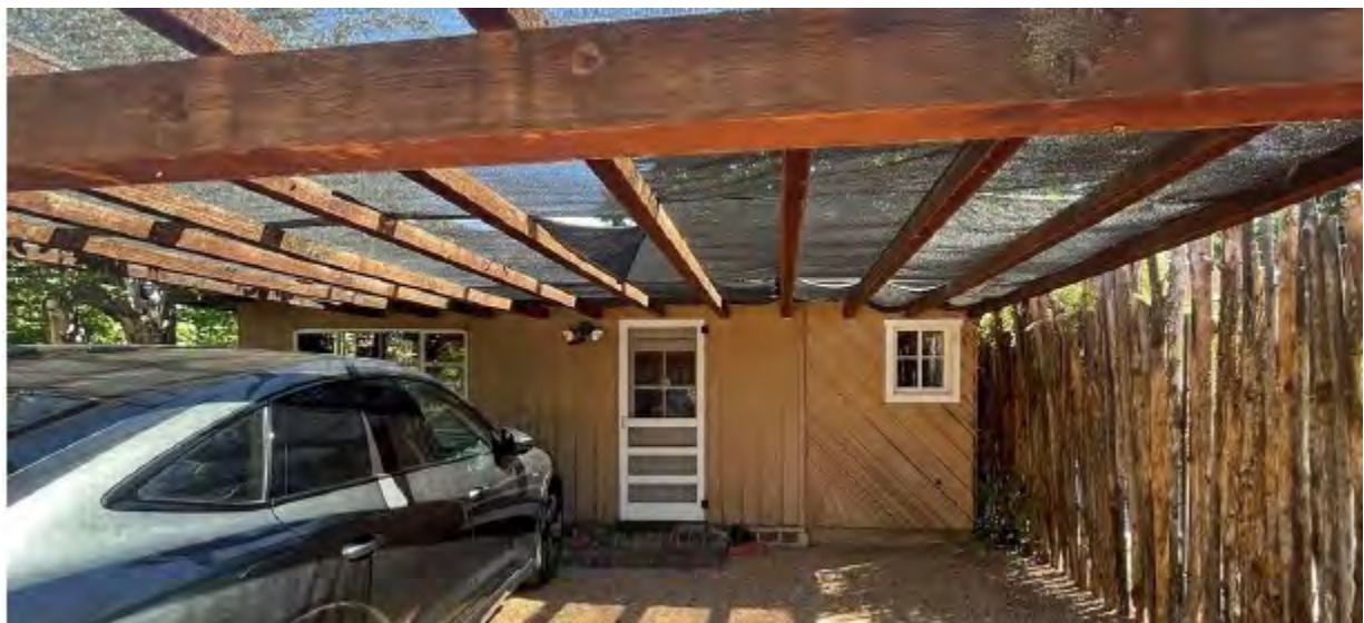
Figure 2: Guesthouse: west elevation under carport
