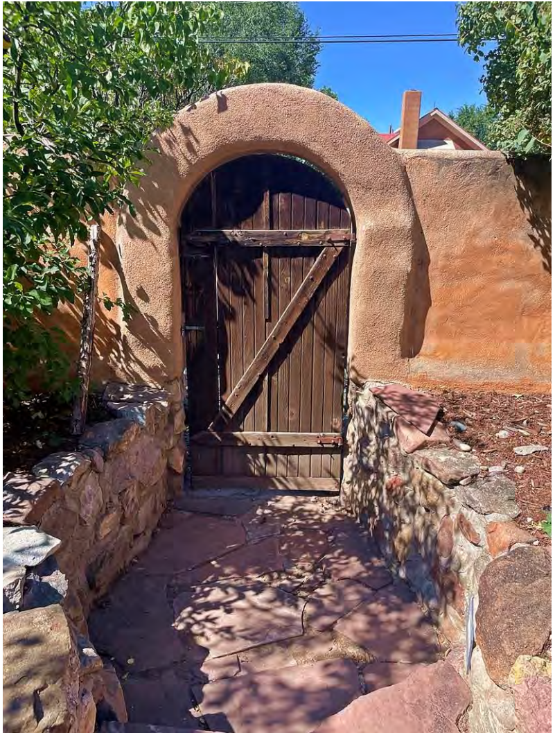
Photo 16: Front wall, entry gate. Camera facing west.
