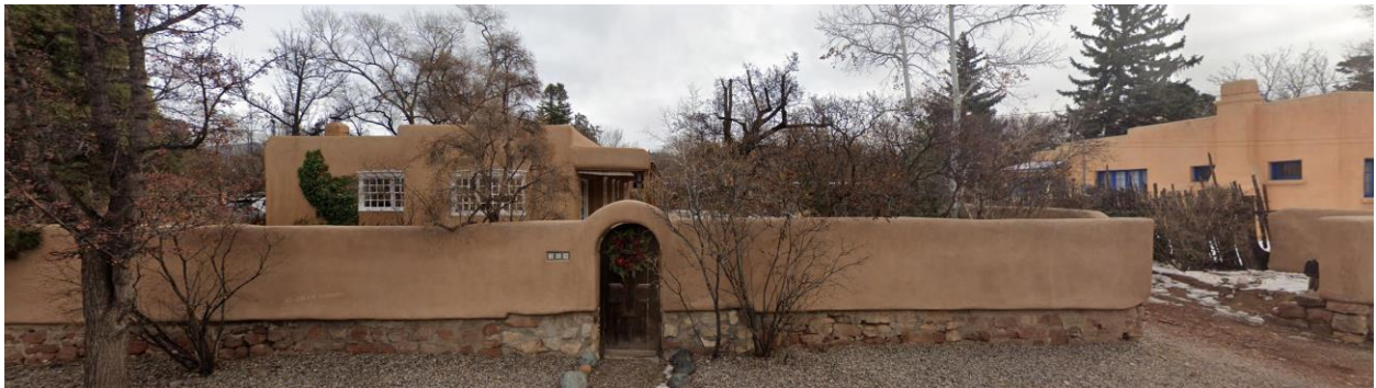
Figure 1: East elevation with front yard wall
