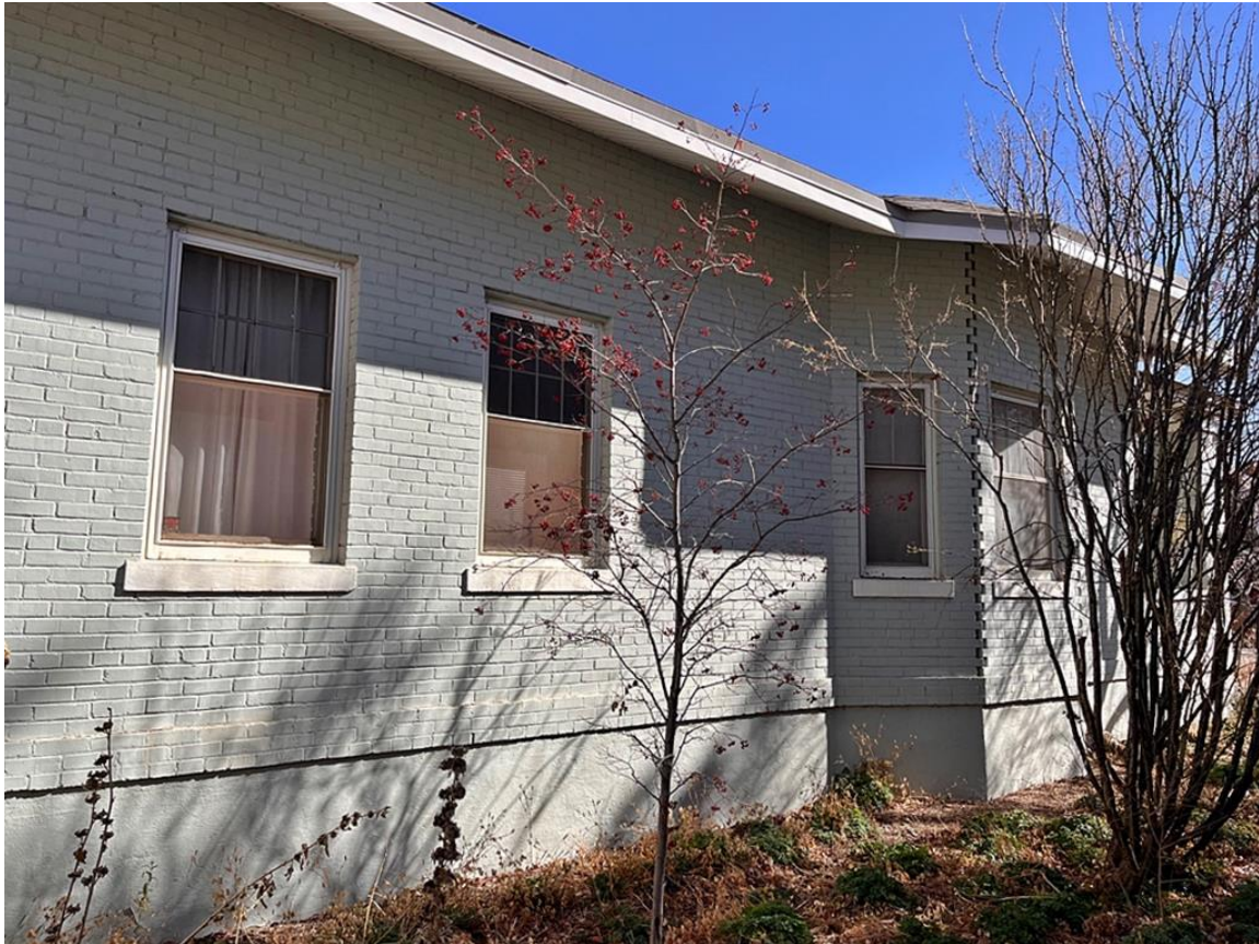
Photo 9: West elevation. Camera facing southeast.
