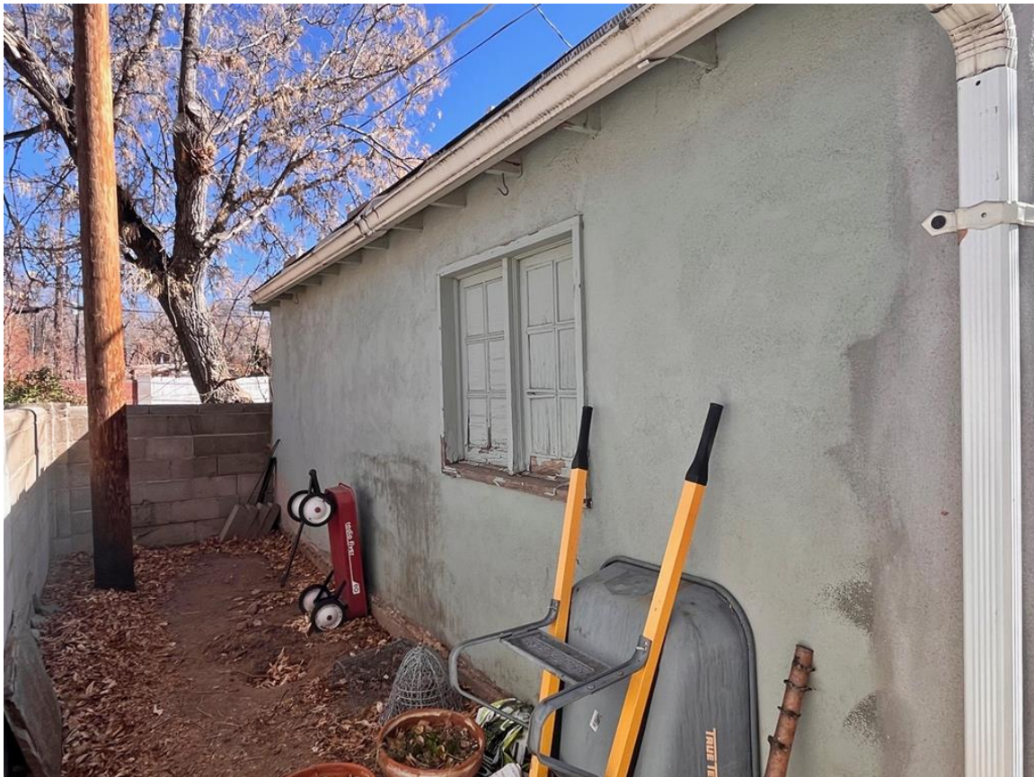
Photo 12: Garage, north elevation. Camera facing southeast.
