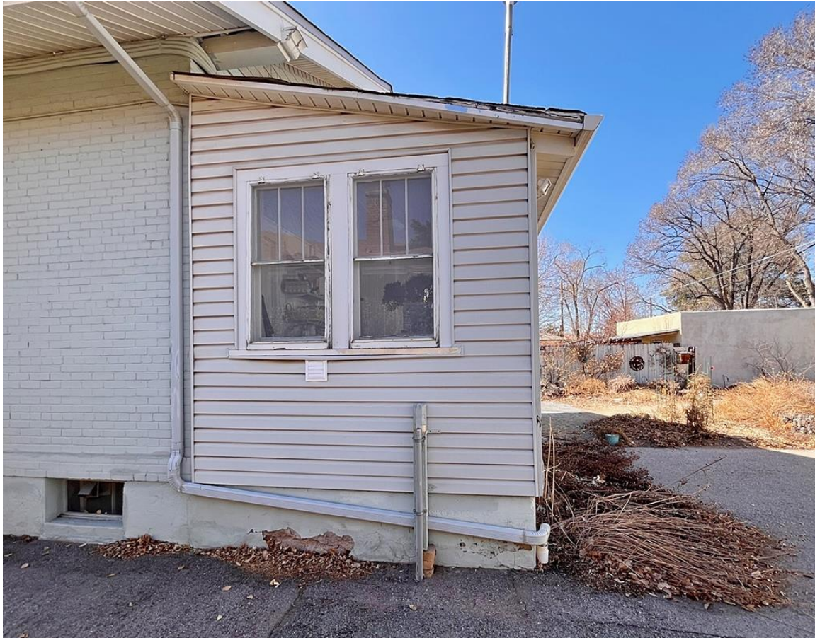
Photo 7: East elevation of mudroom addition. Camera facing west.
