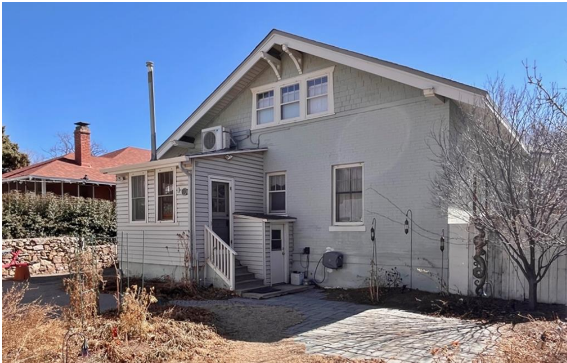
Photo 8: North elevation. Camera facing southeast.
