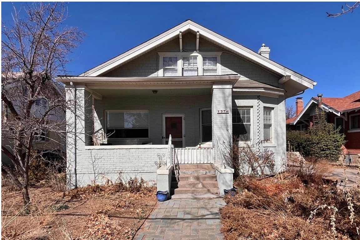
Photo 2: Front (south) façade. Camera facing north.
