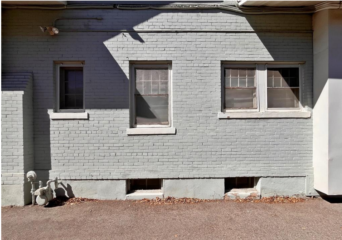
Photo 6: East elevation windows. Camera facing west.
