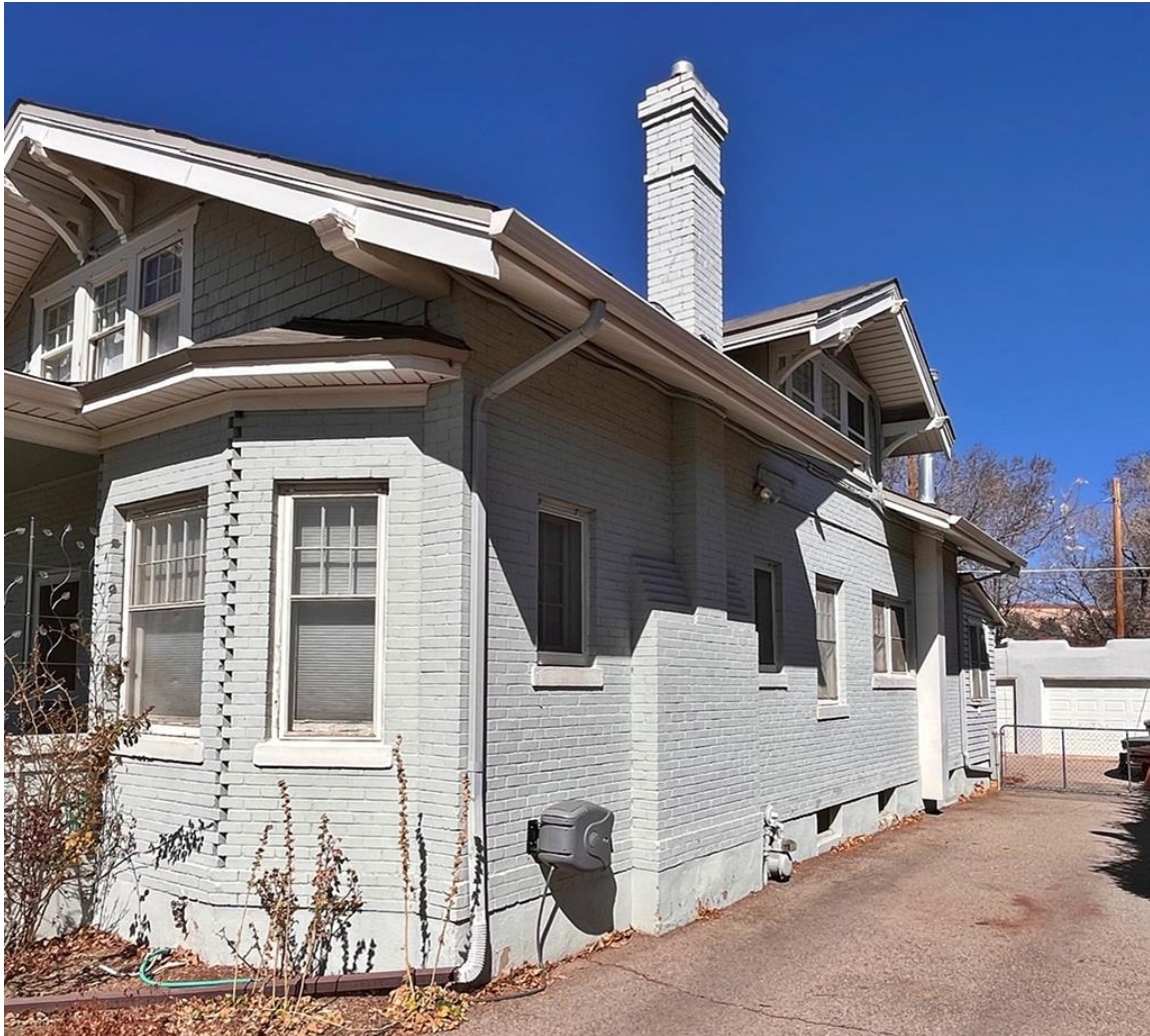
Photo 4: Bay window and east elevation. Camera facing northwest.
