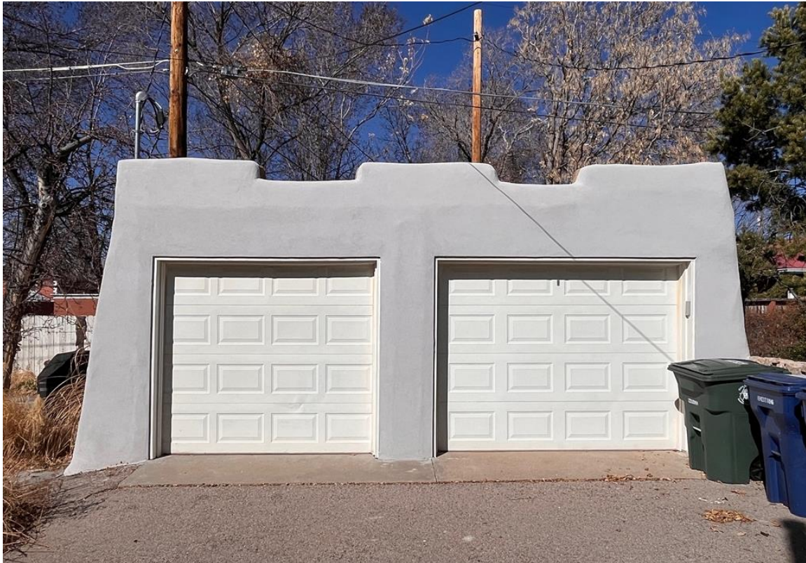
Photo 12: Garage, south elevation. Camera facing north.
