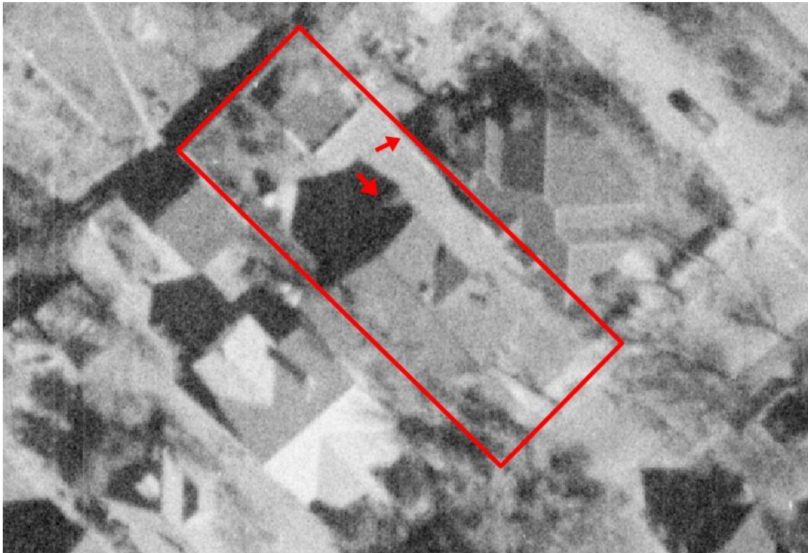
Figure 6: November 10, 1958, aerial photograph. Note structure along east property line and mudroom.
