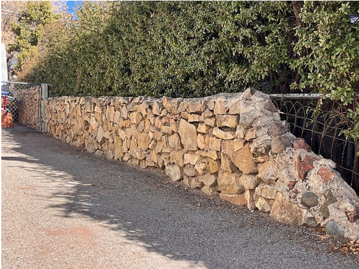
Photo 14: East property wall. Camera facing northeast.
