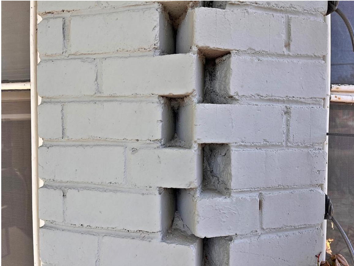
Photo 5: Bricks at the bay window. Camera facing northwest.
