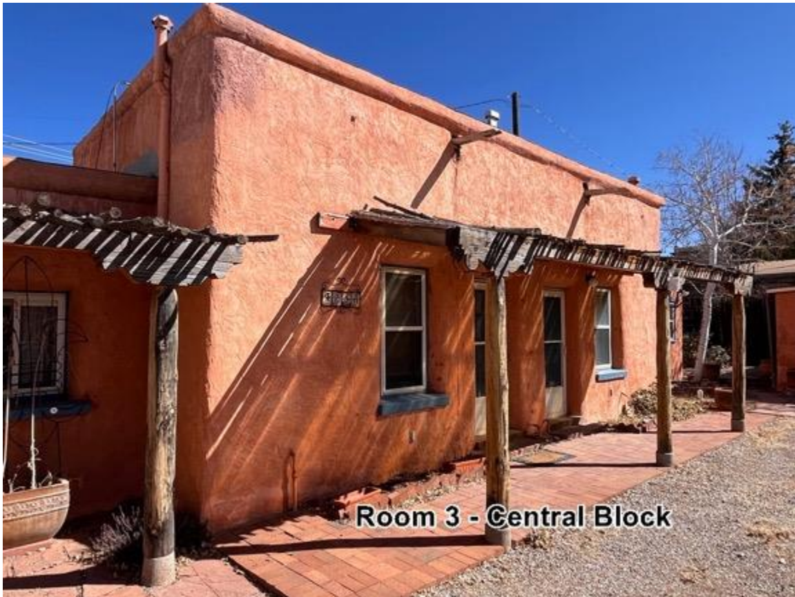
Photo 15: Room 3 (Central Block). Camera facing northeast.
