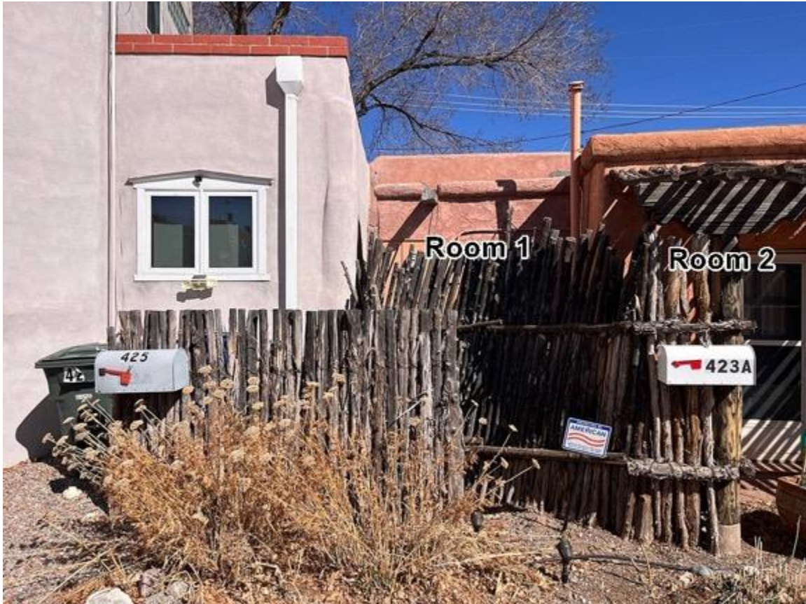
Photo 6: West end of subject building, holding Rooms 1 and 2. White building to the left, replaced the Trinidad Chavez House. Camera facing north.
