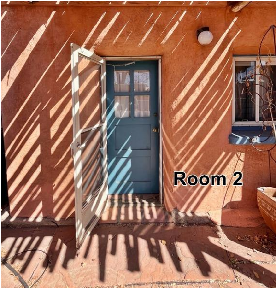
Photo 11: Room 2. Door and window. Camera facing north.
