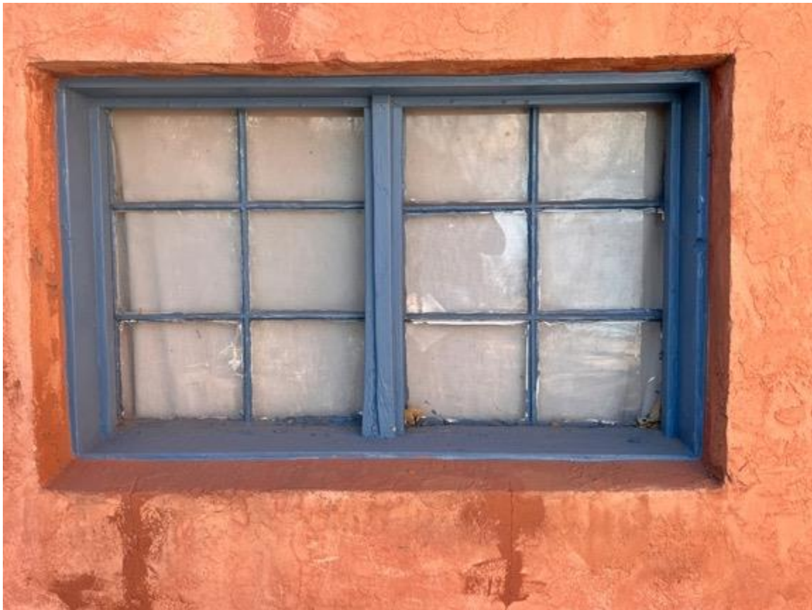
Photo 33: Garage. North elevation. Window. Camera facing south.
