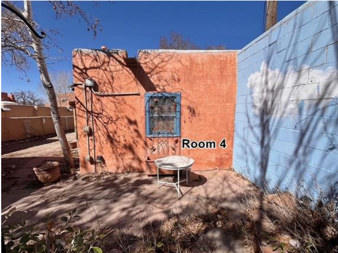
Photo 26: Room 4. East elevation. Camera facing west.
