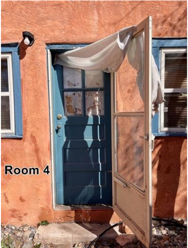
Photo 25: Room 4. Door. Camera facing north.
