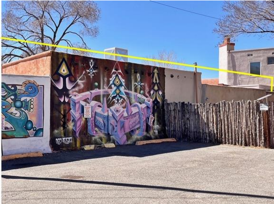
Photo 28: Subject building. North elevation at North Guadalupe Street parking lot. Camera facing southwest.
