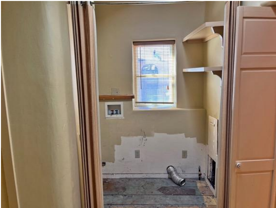
Photo 27: Room 4. Interior, frame bathroom enclosure. Camera facing south.
