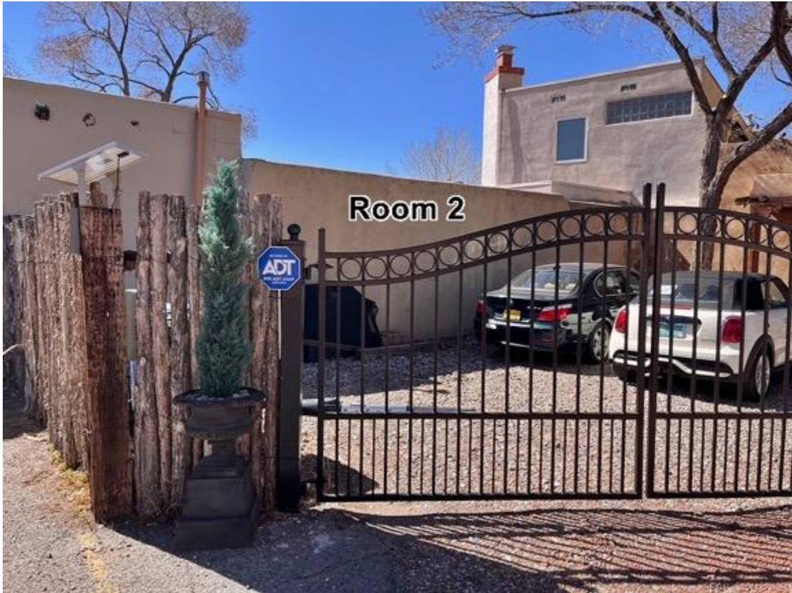
Photo 30: Room 2. North elevation. Camera facing southwest.
