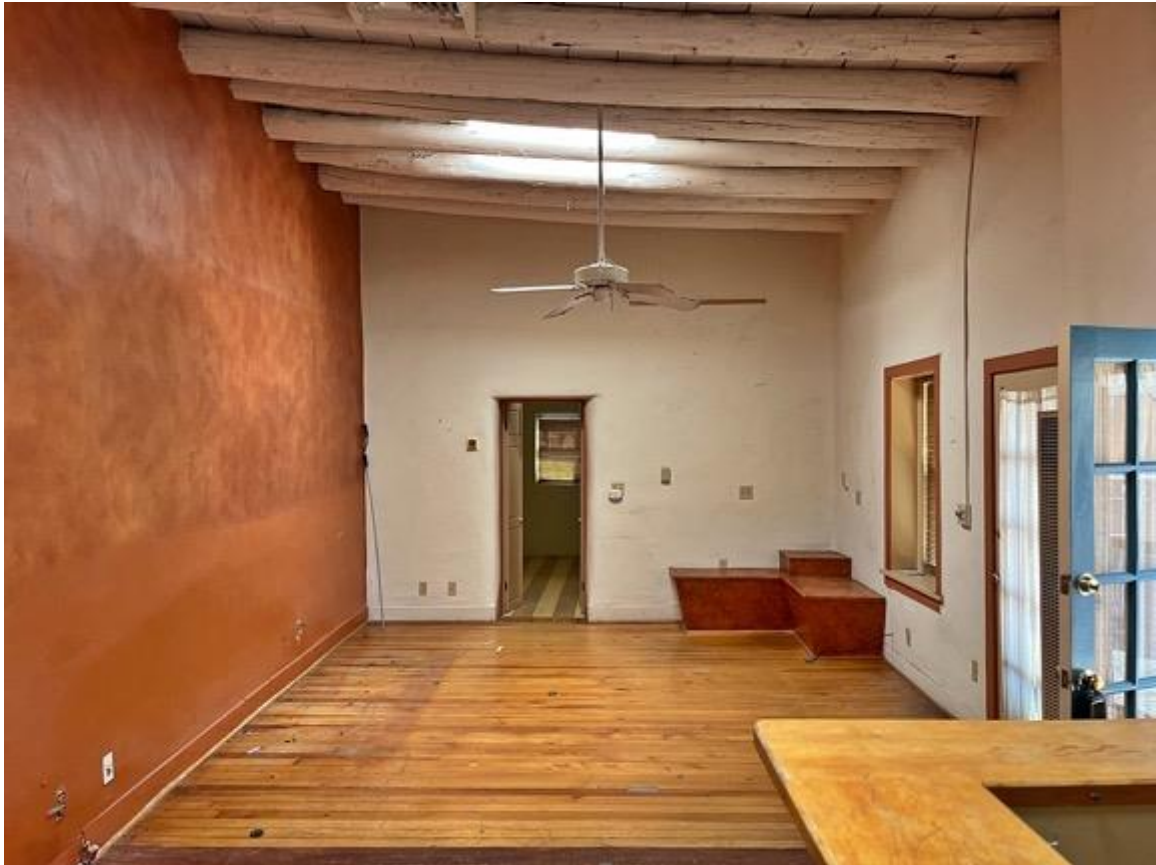
Photo 19: Room 3. Interior. Camera facing east.
