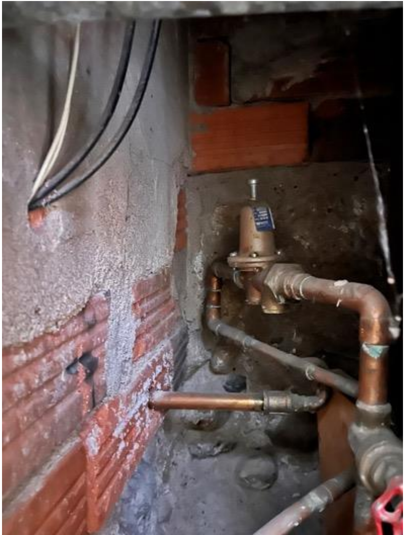
Photo 8: Room 1. Interior showing tile construction behind the plumbing access door.
