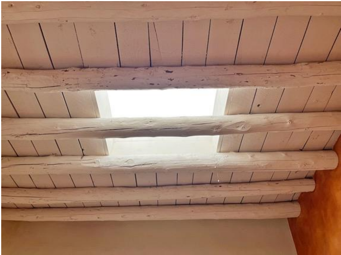
Photo 22: Room 3. Interior ceiling.
