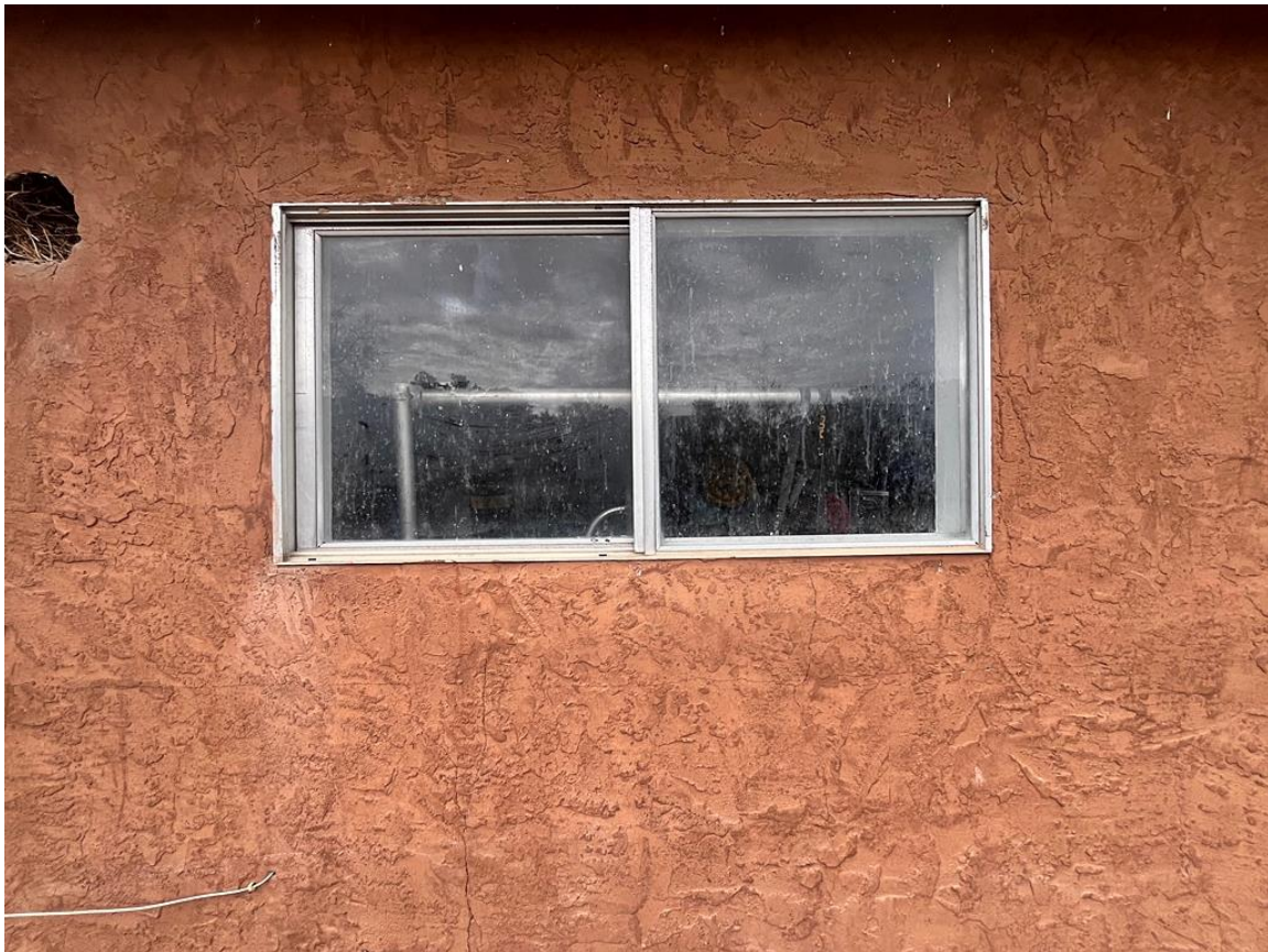
Photo 9: Aluminum sliding window on east elevation. Camera facing northwest.
