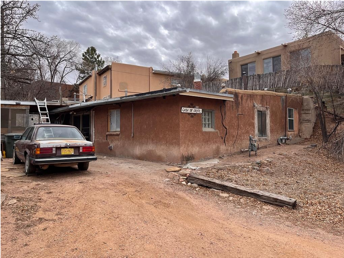
Photo 16: 537 ½ Rodriguez Street, the former José and Rosalina Ortiz House. Camera facing southeast.
