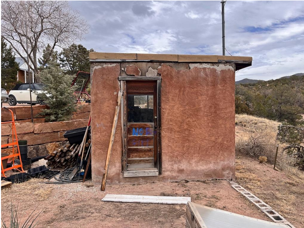
Photo 5: West elevation. Camera facing northeast.
