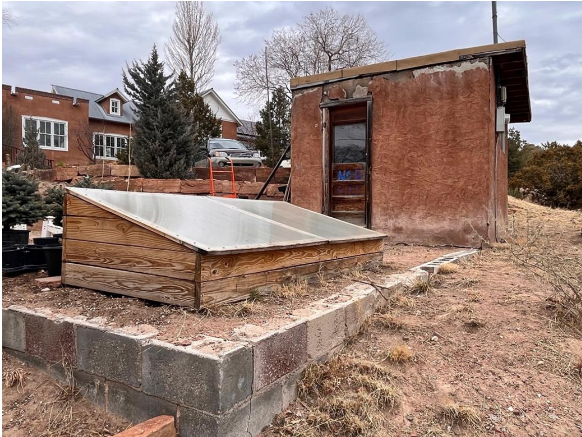
Photo 14: Low foundation wall. Camera facing northeast.
