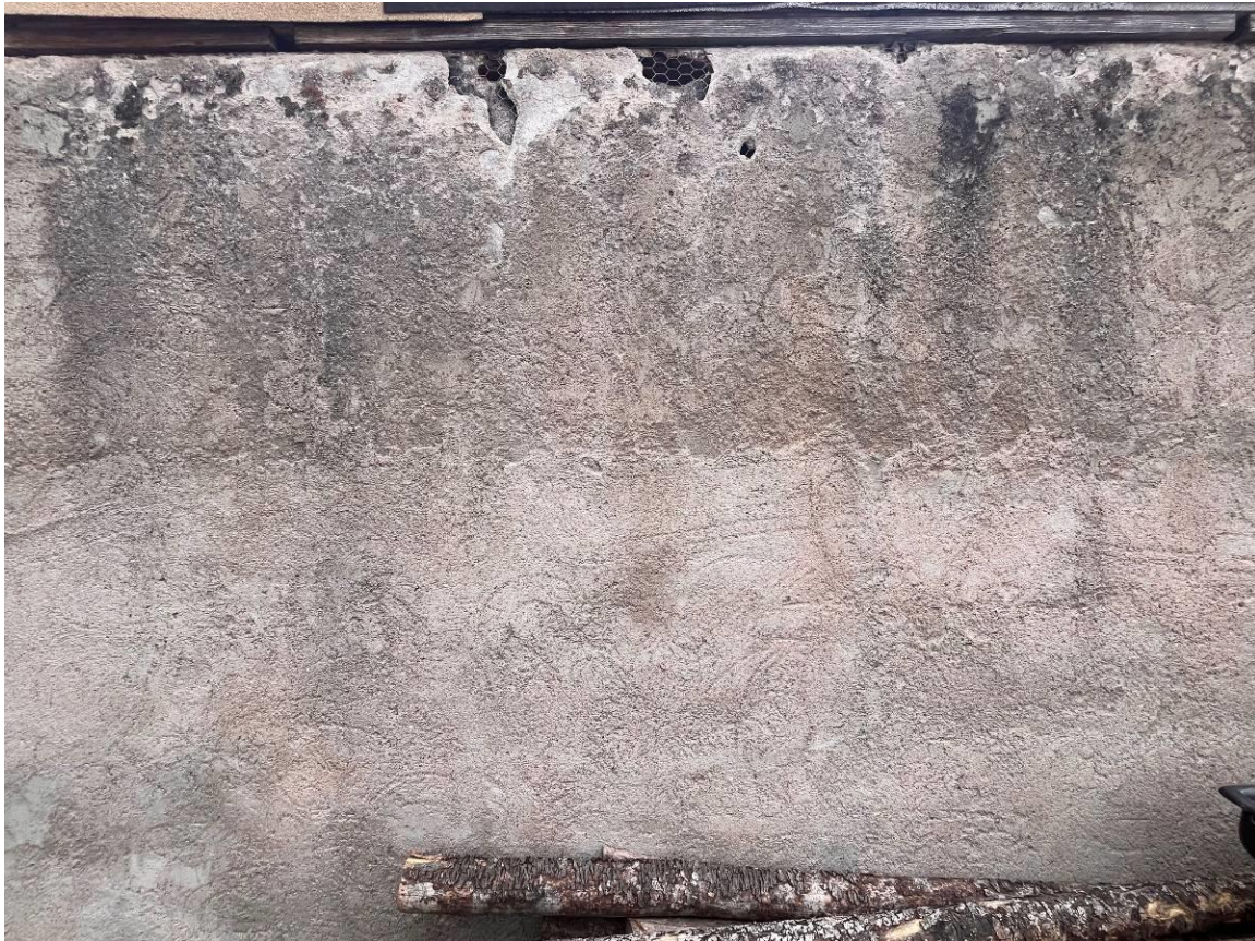
Photo 11: North elevation. Camera facing southeast.
