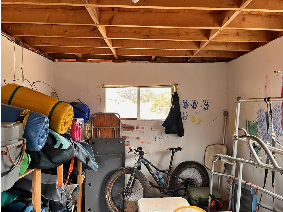
Photo 12: Interior of shed. Camera facing northeast.
