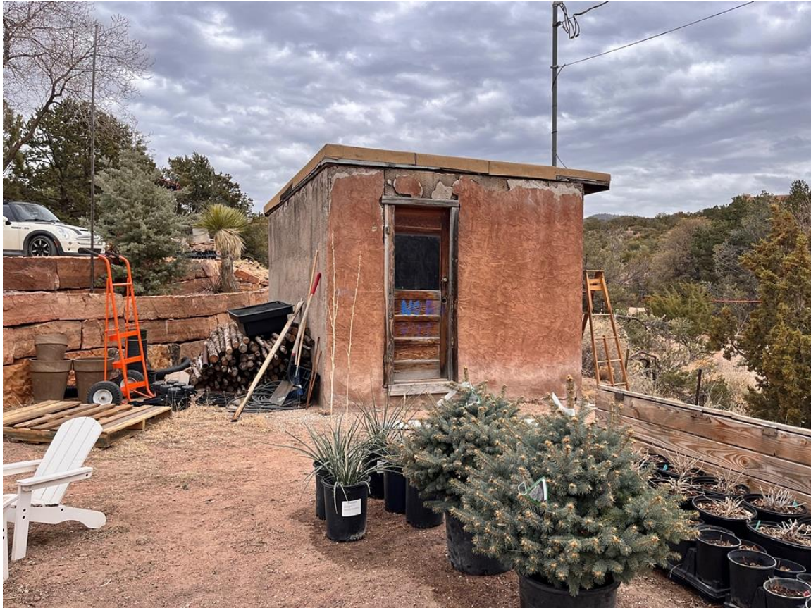
Photo 4: West elevation and immediate setting. Camera facing northeast.
