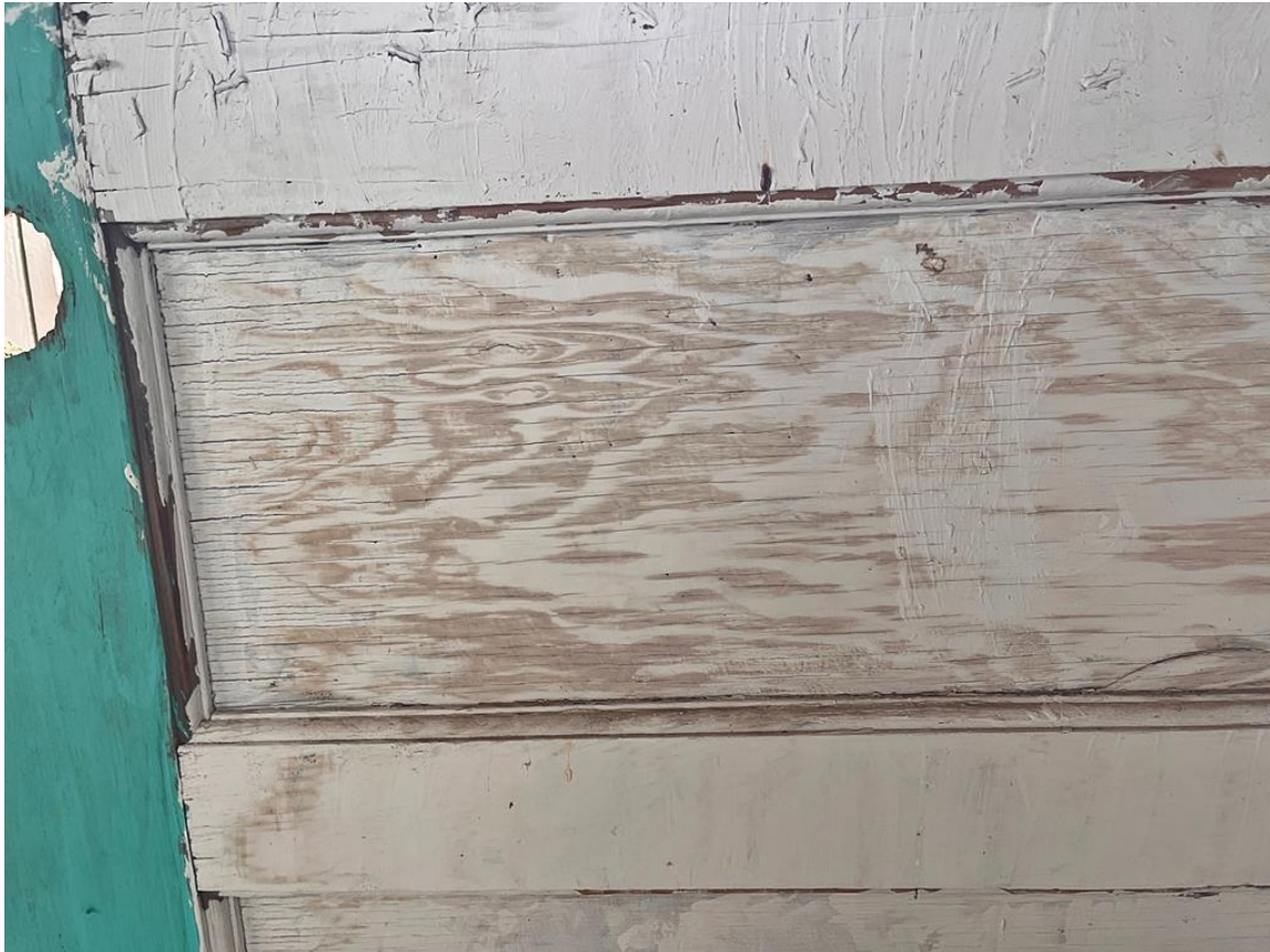
Photo 7: Interior of west door.
