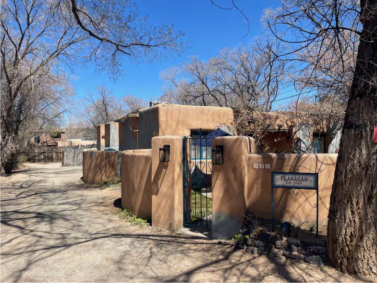
925 Residence and Casita Southwest Elevation from Street
