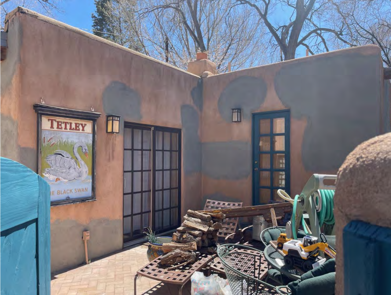
925 Residence Northwest Elevation at Entry
