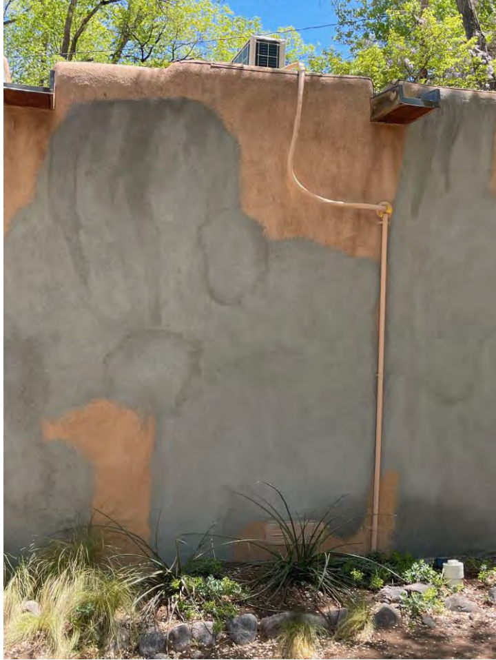
925 Residence West Elevation Roof HVAC Line
