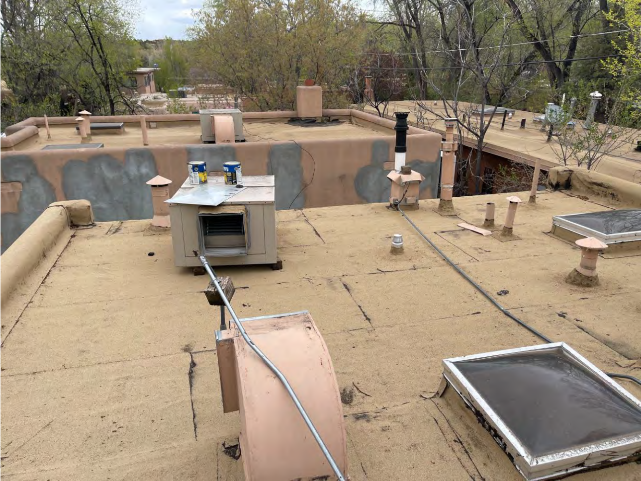
925 Residence and Casita Roof
