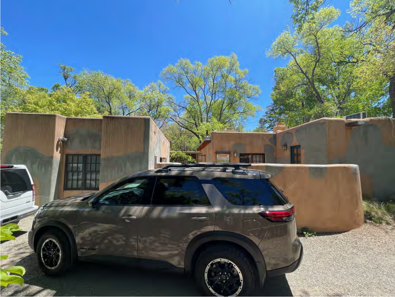
925 Residence and Casita West Elevation
