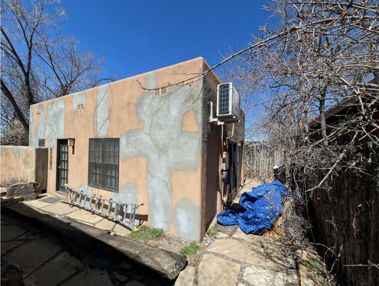
925 Casita Southeast Elevation at Courtyard
