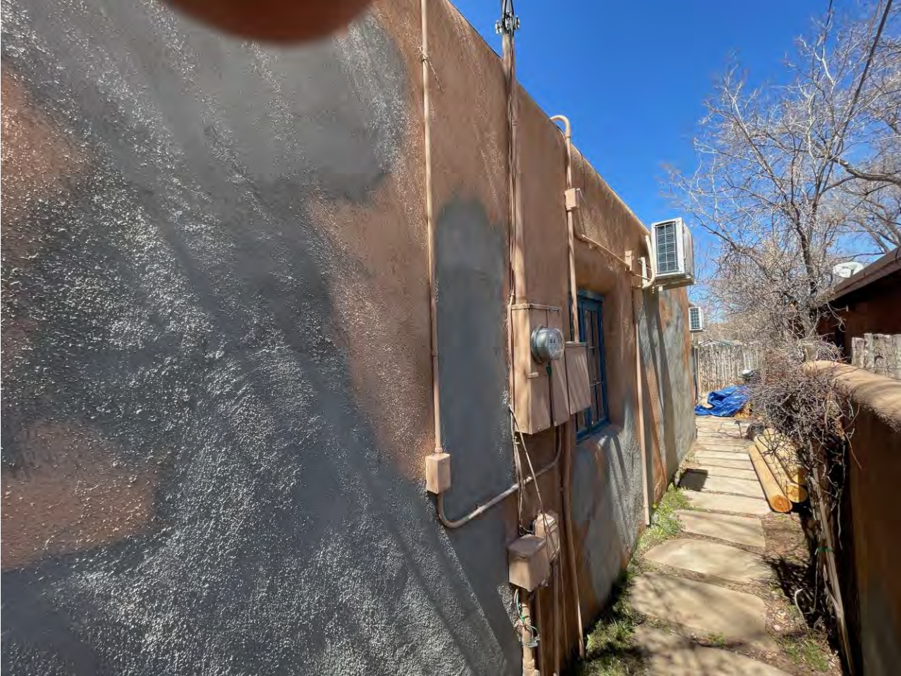
925 Residence and Casita East Elevation with HVAC Units
