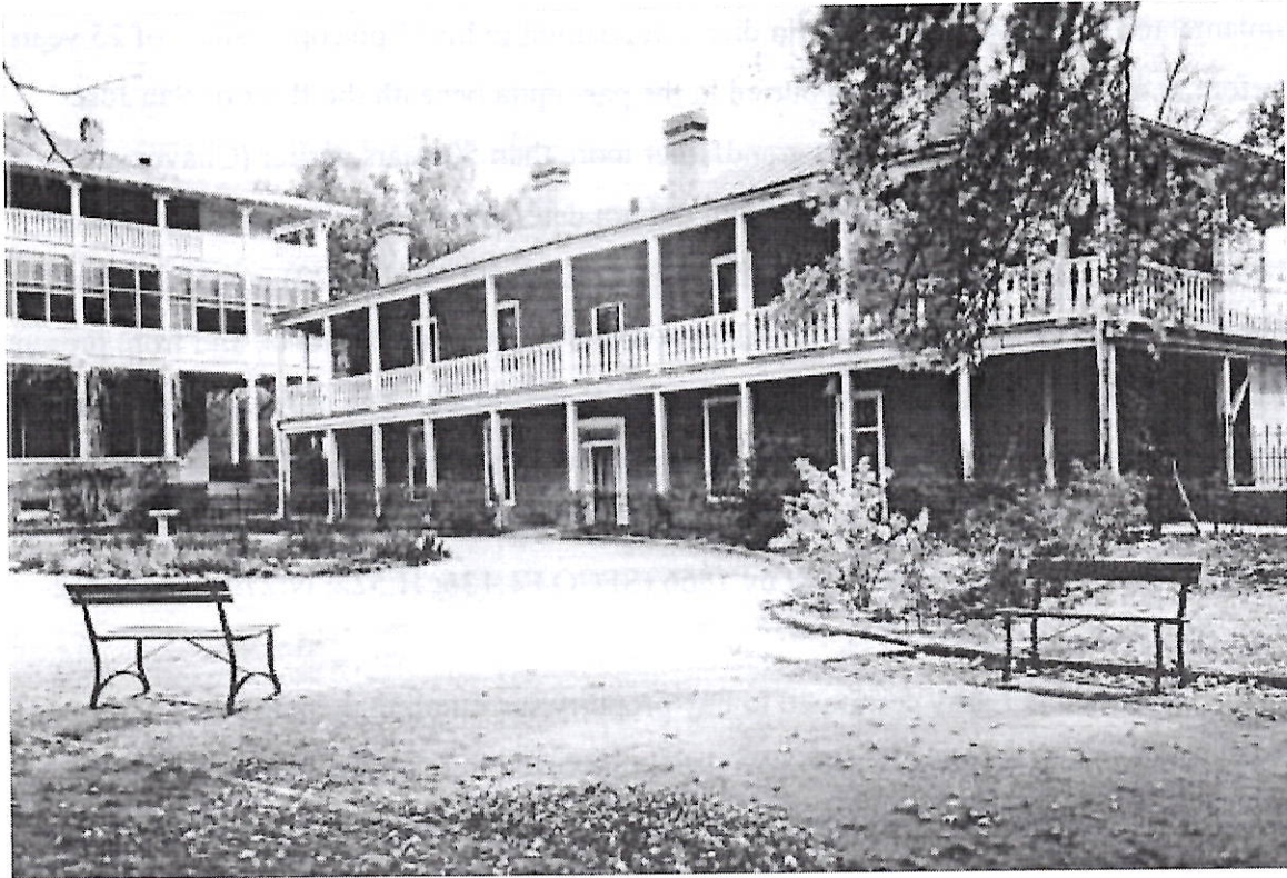
Fig. 6. The Old Seminary. Constructed in 1853 by Carlos Brun as a single story building for use as a rectory and boys school for Bishop Lamy (see Fig. 4). The second story with porches was added by the Sisters of Charity after 1865 when they used the building as a hospital. Sleeping porches on Marian Hall can be seen in the left. The Old Seminary was demolished in 1954. Photograph from Kimball and Smith 1977.
