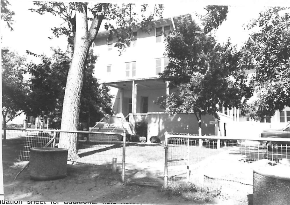
#35 west elevation, N end
