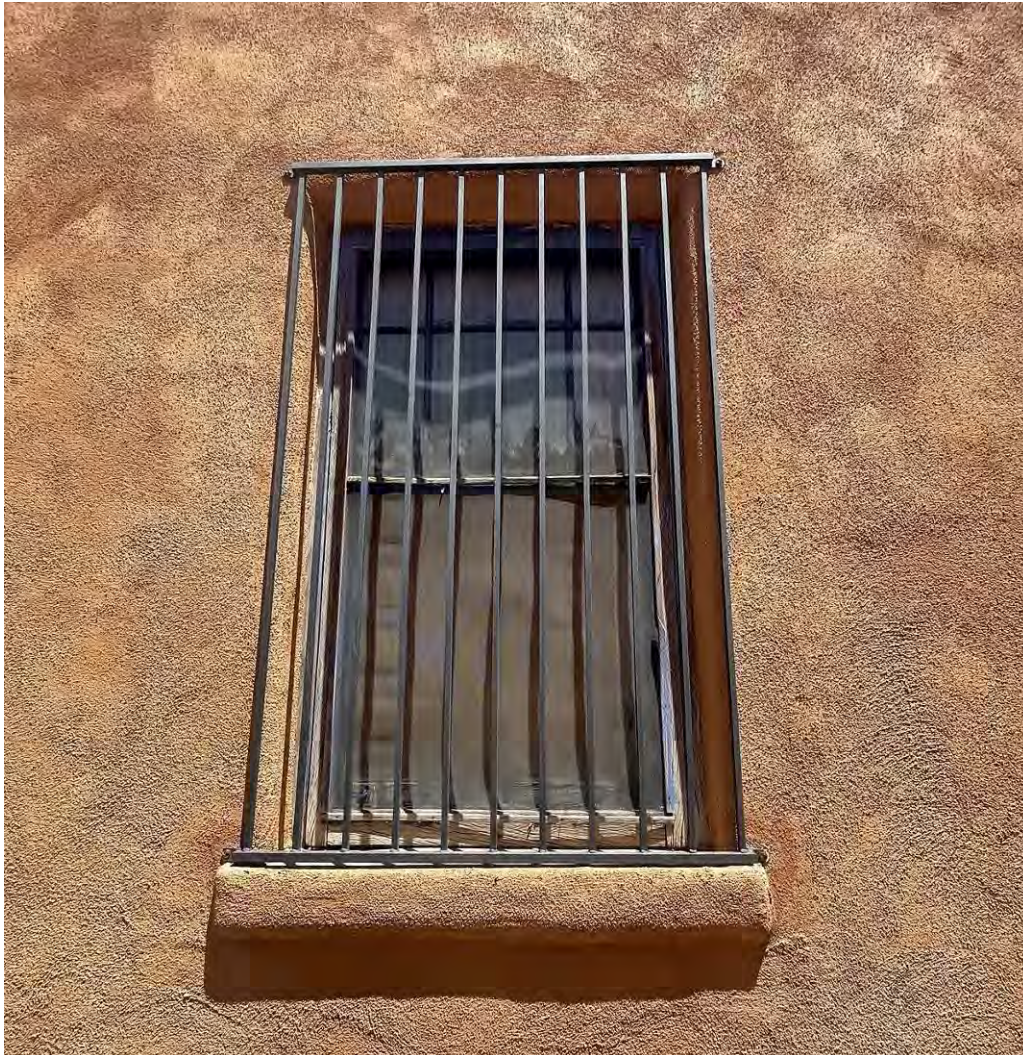
Photo 9: South elevation. Original 8/1 window. Camera facing up.
