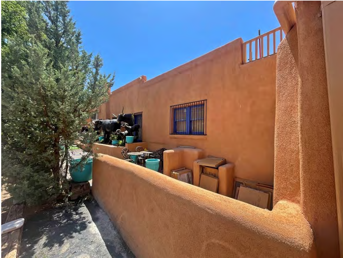
Photo 6: North elevation oblique. Addition with railing at right. Camera facing northeast.
