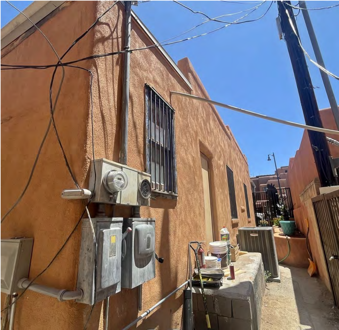
Photo 8: South elevation oblique. Enclosed porch or non-historic addition at left. Camera facing northeast.
