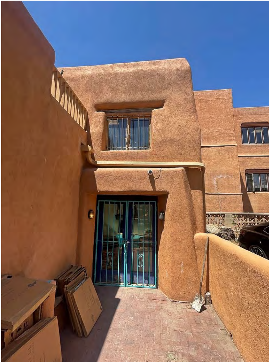
Photo 10: Back building, east elevation, north end. Camera facing west.
