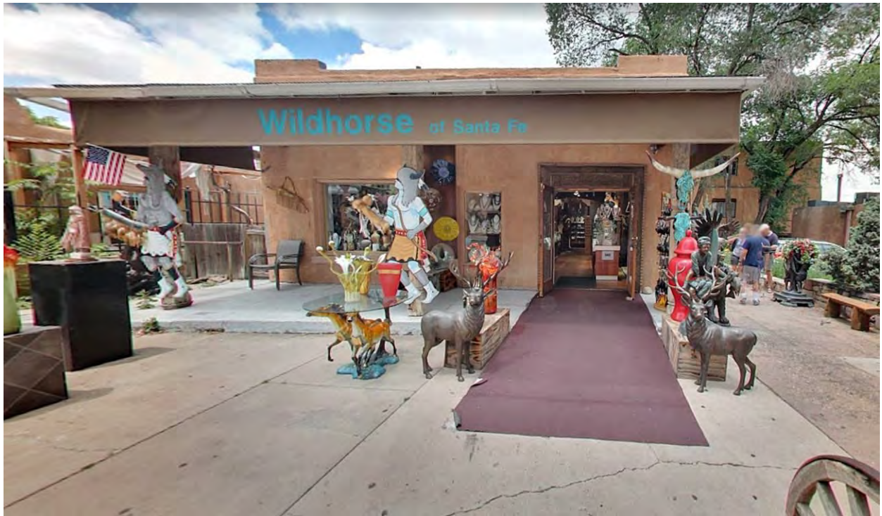
Figure 2: Google Street View image of east façade. Note smaller double wood doors and smaller two wood windows.
