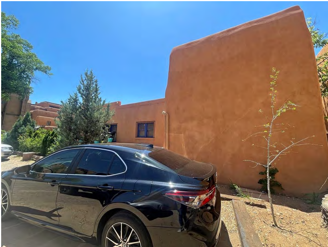
Photo 11: Back building, north elevation. Camera facing southeast.
