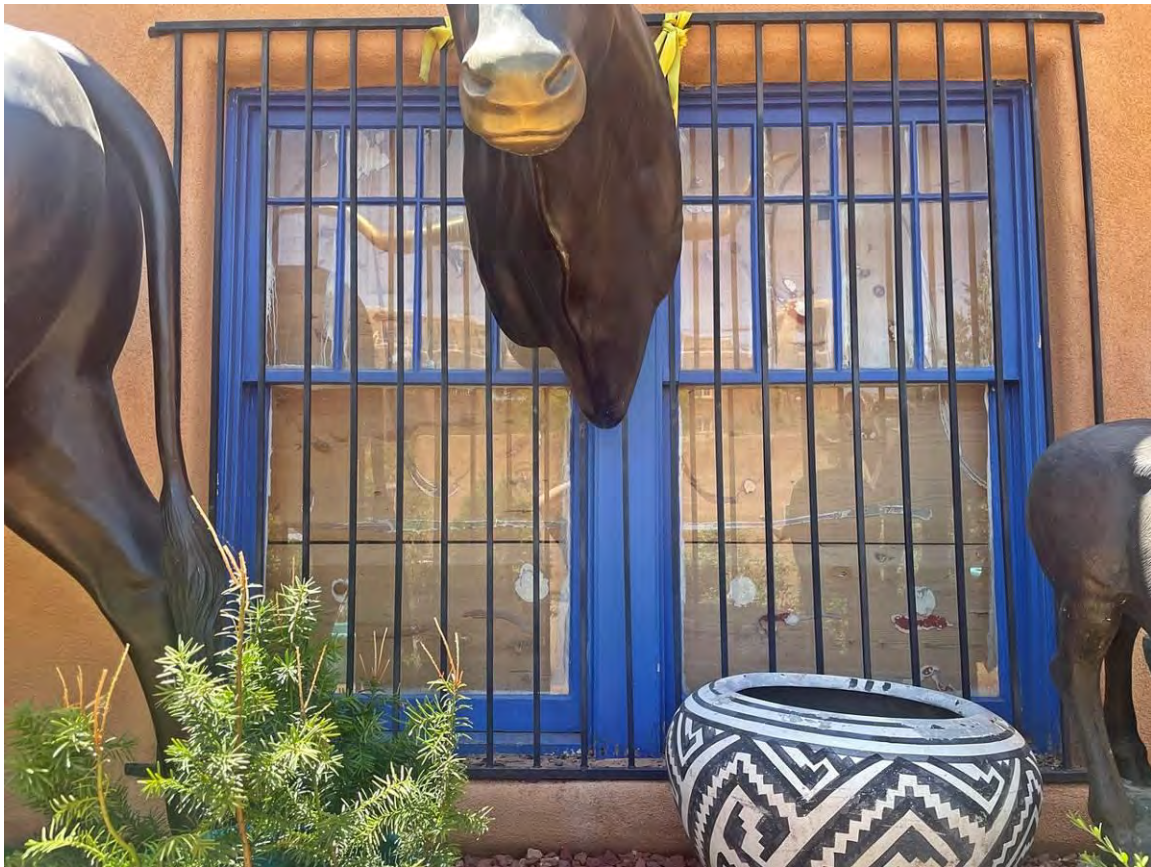
Photo 5: North elevation. Window # 3. Camera facing south.
