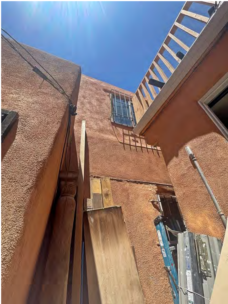
Photo 13: Back building, central east elevation. Camera facing up.
