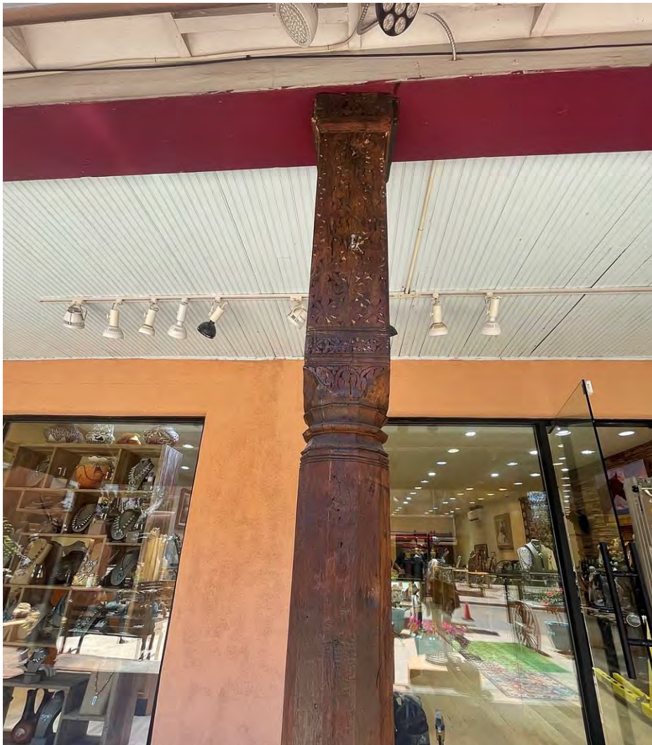
Photo 2: East façade, new porch support. Camera facing up.
