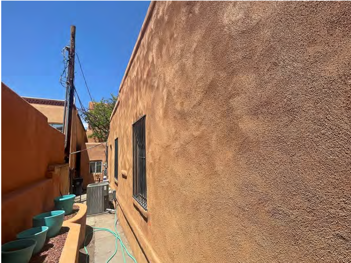
Photo 7: South elevation oblique, east end. Camera facing northwest.
