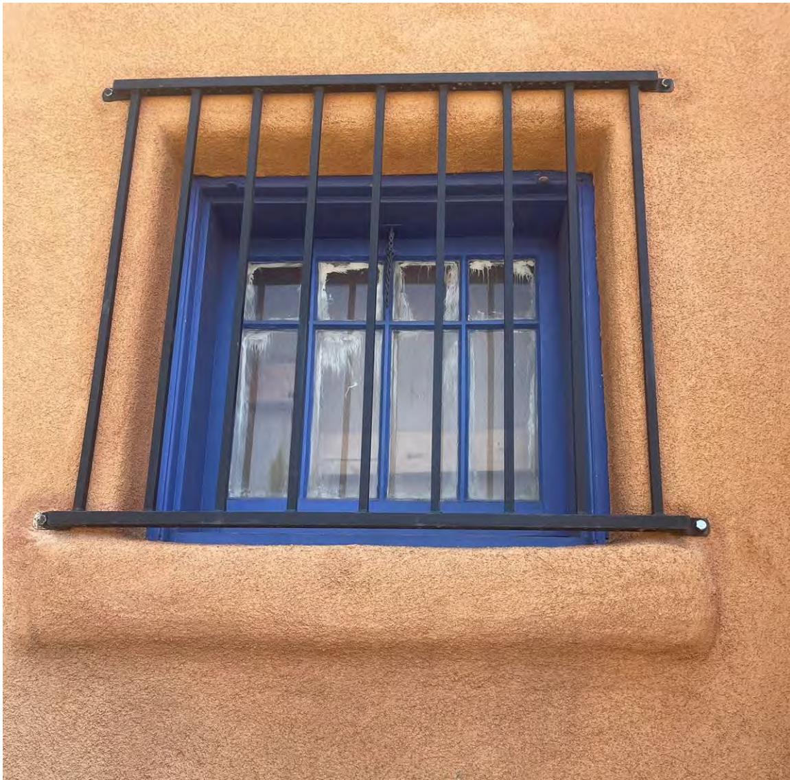
Photo 4: North elevation. Window #1. Camera facing up.
