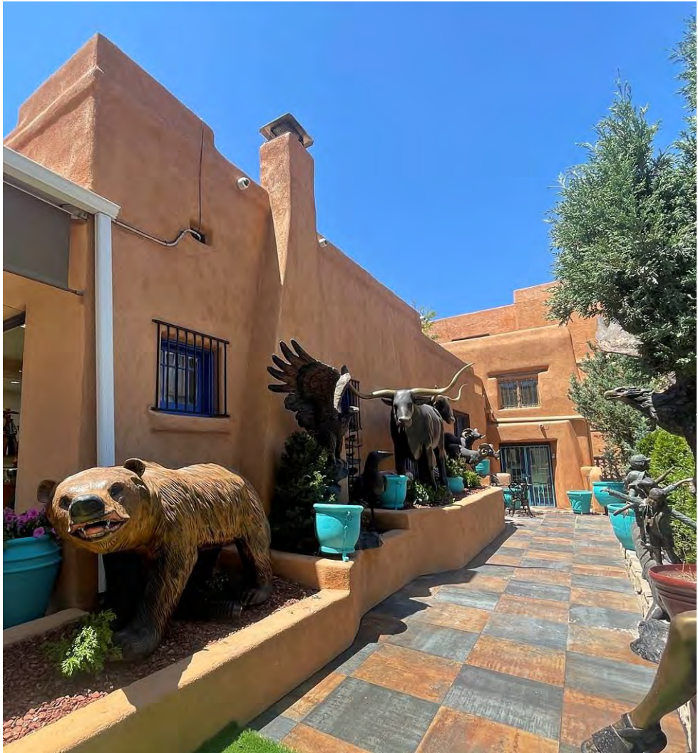
Photo 3: North elevation oblique. Camera facing southwest. Attached back building at right.
