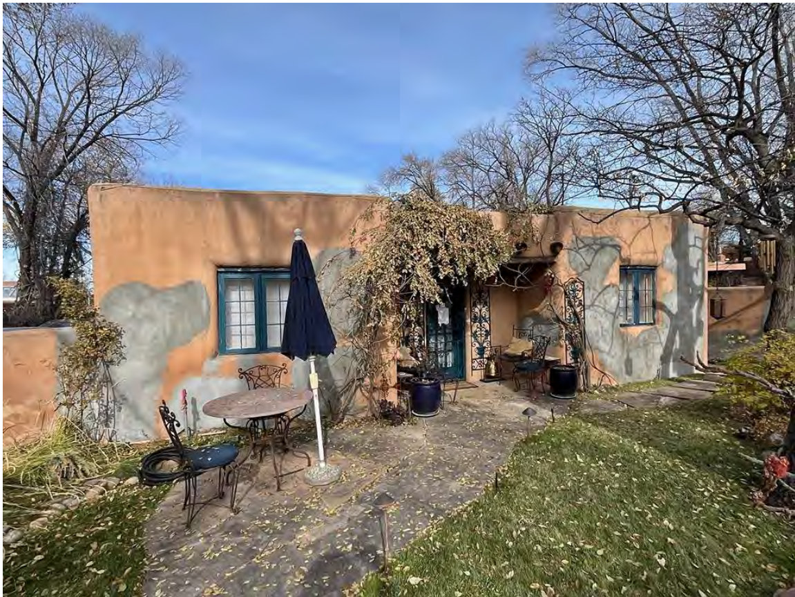
Photo 2: South (front) elevation. Camera facing northeast.
