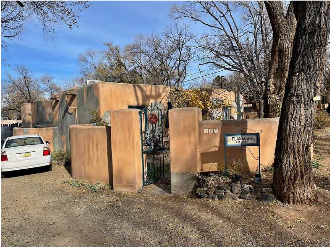
Photo 13: Entry gate and curved wall. Camera facing northeast. Note gate and wall were erected in c.2002.
