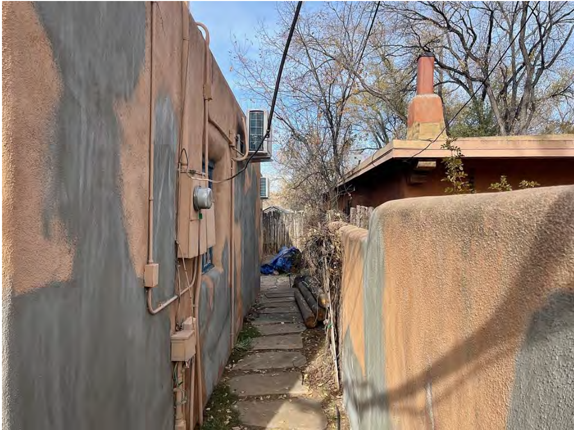
Photo 6: East elevation oblique. Camera facing north.
