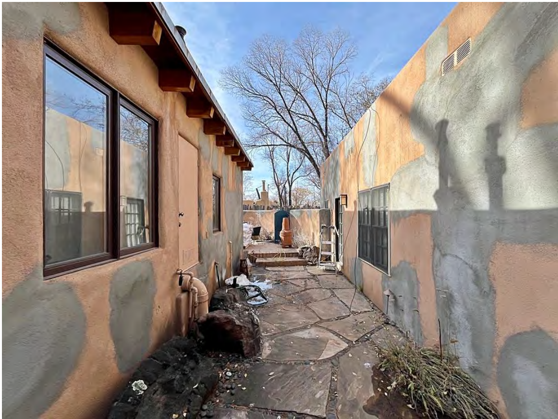
Photo 9: North elevation oblique. 2003 guesthouse at right. Camera facing west.
