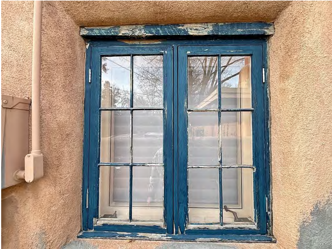
Photo 7: East elevation. Window. Note geared crank-out hardware. Camera facing west.
