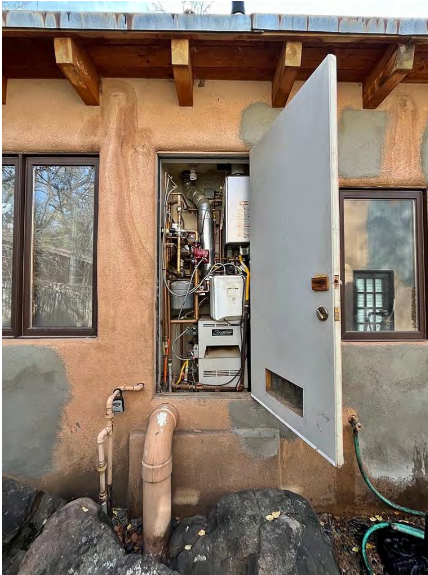
Photo 10: North elevation. Mechanical room entry. Camera facing south.
