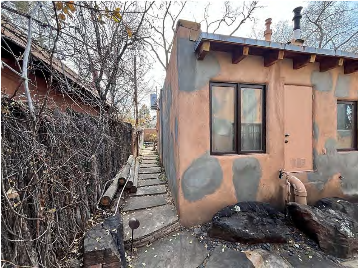
Photo 8: North elevation. Northeast corner. Camera facing southwest.
