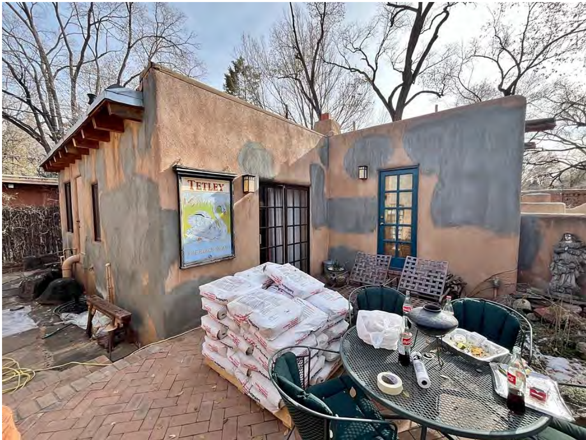
Photo 11: Northwest (patio) elevation. Camera facing southeast.
