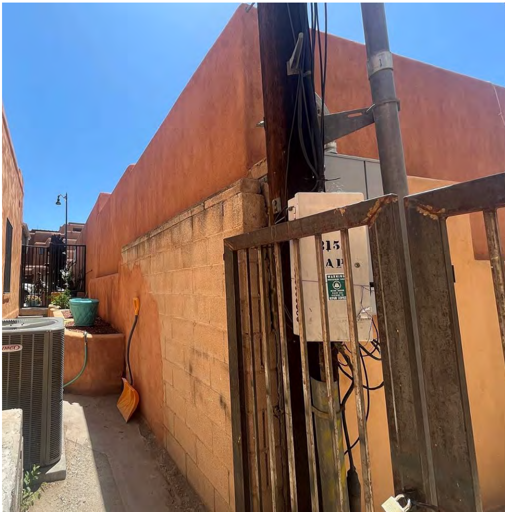
Photo 2: North elevation. Camera facing southeast.
