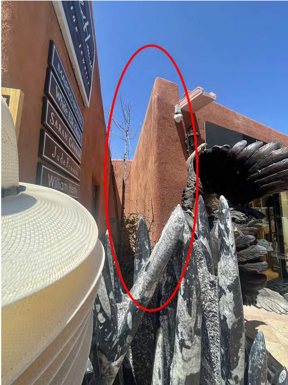
Photo 3: South elevation. Camera facing northwest.
