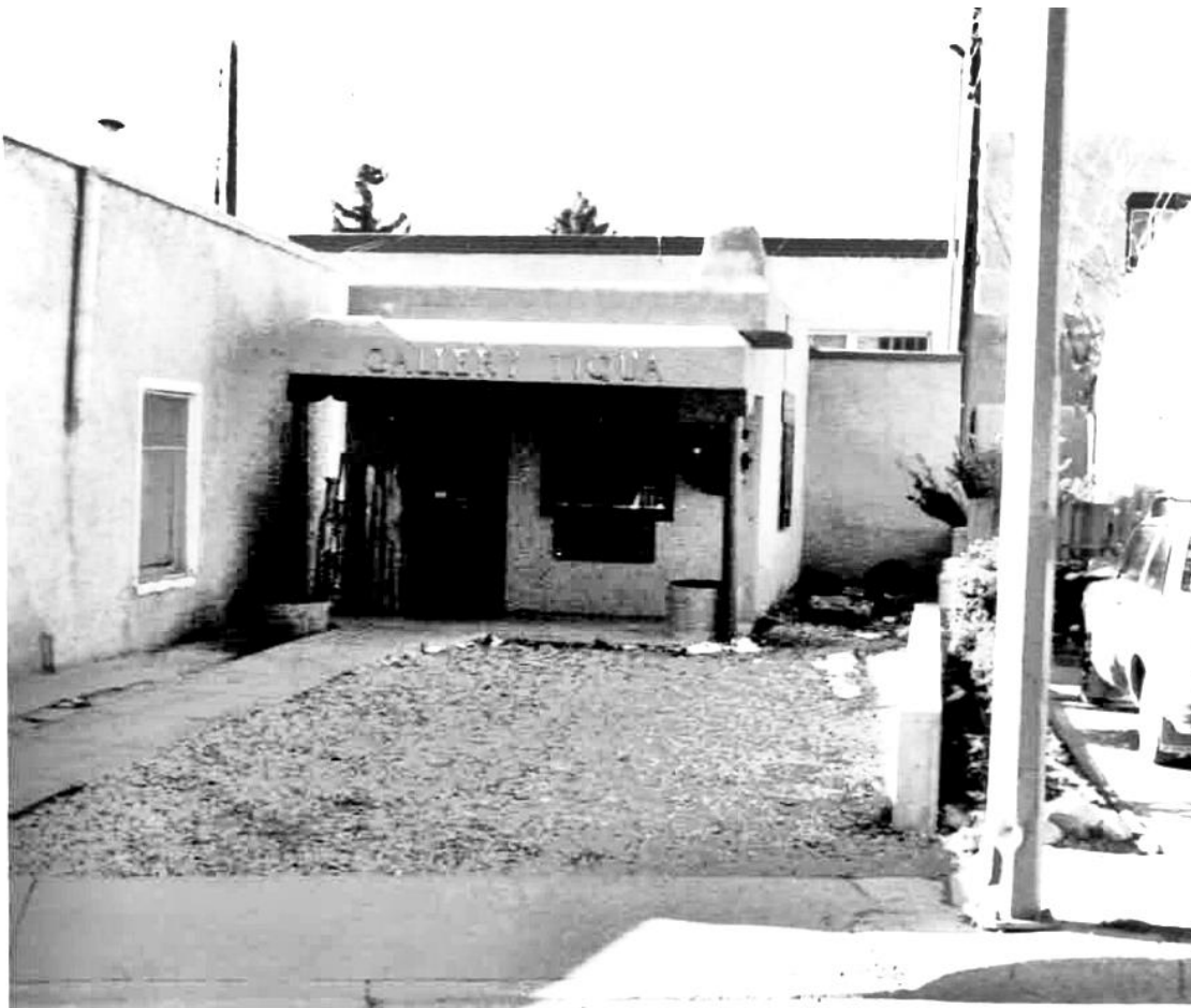
Figure 1: December 20, 1984, HBI survey photo. Harry Weiss. Courtesy NMCRIS.
