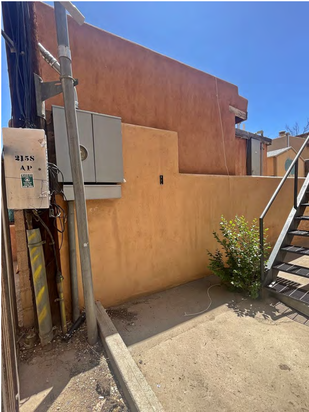
Photo 4: West elevation. Camera facing southeast.
