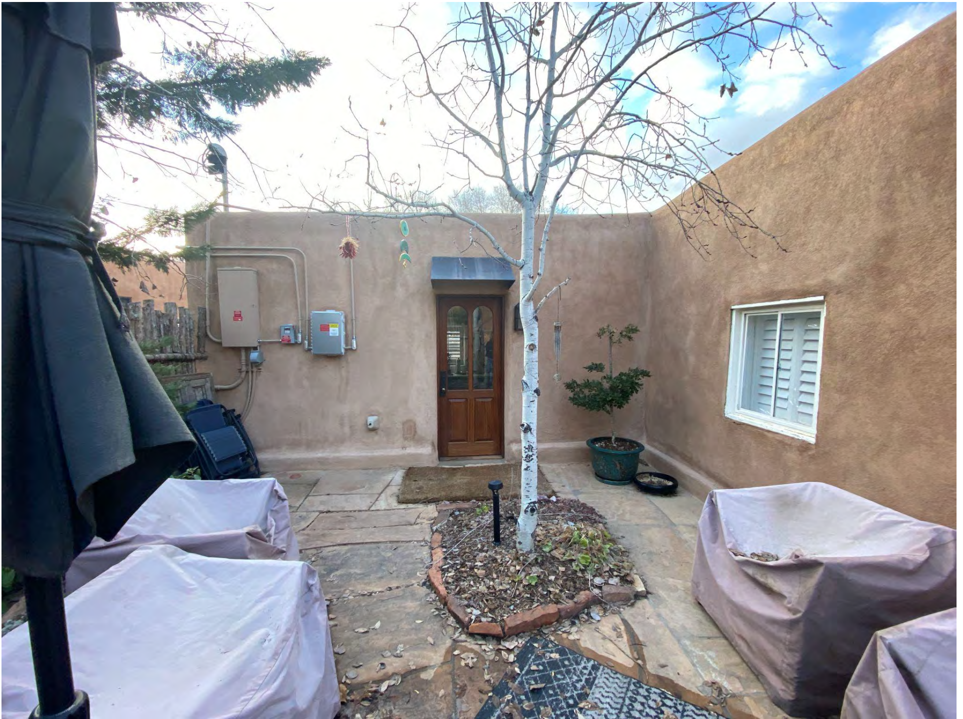
512 Abeyta Street Santa Fe, NM 87505- East Elevation
