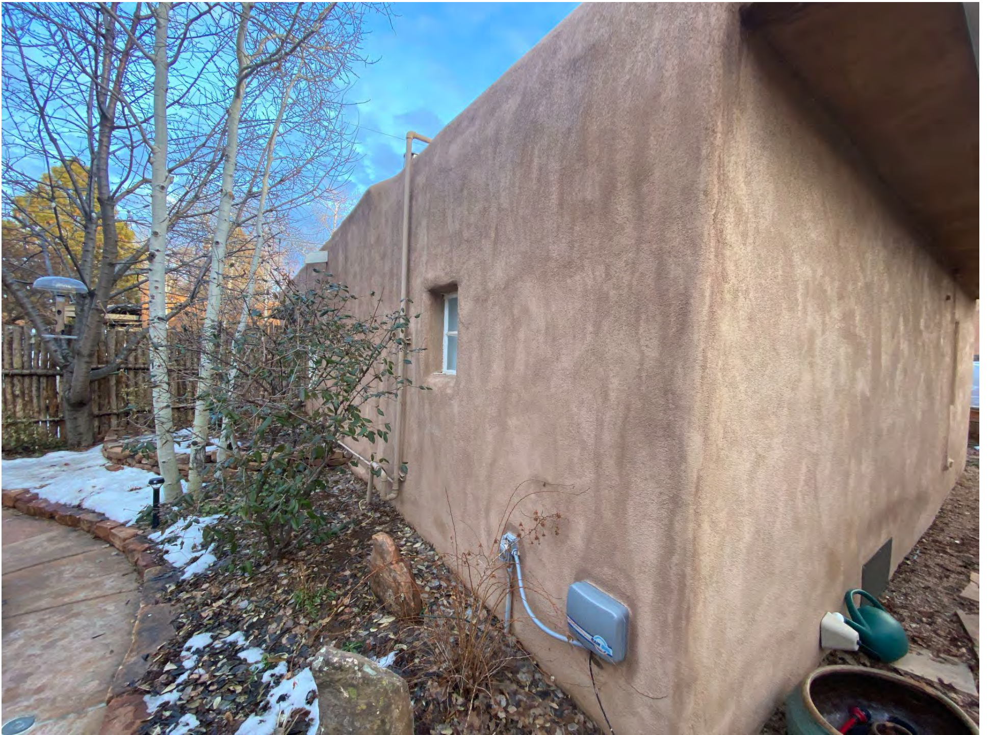
512 Abeyta Street Santa Fe, NM 87505- South Elevation
