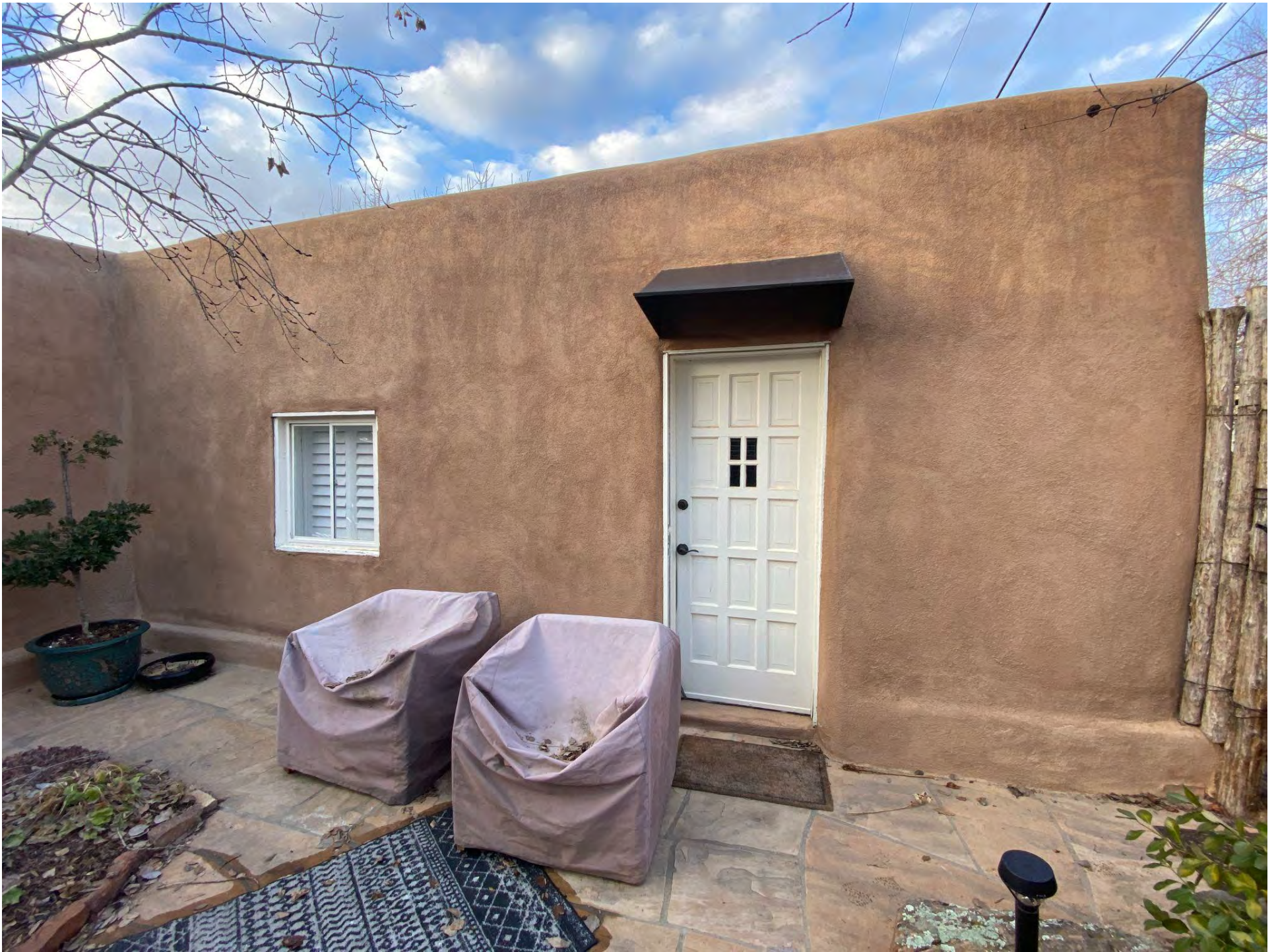
512 Abeyta Street Santa Fe, NM 87505- South Elevation
