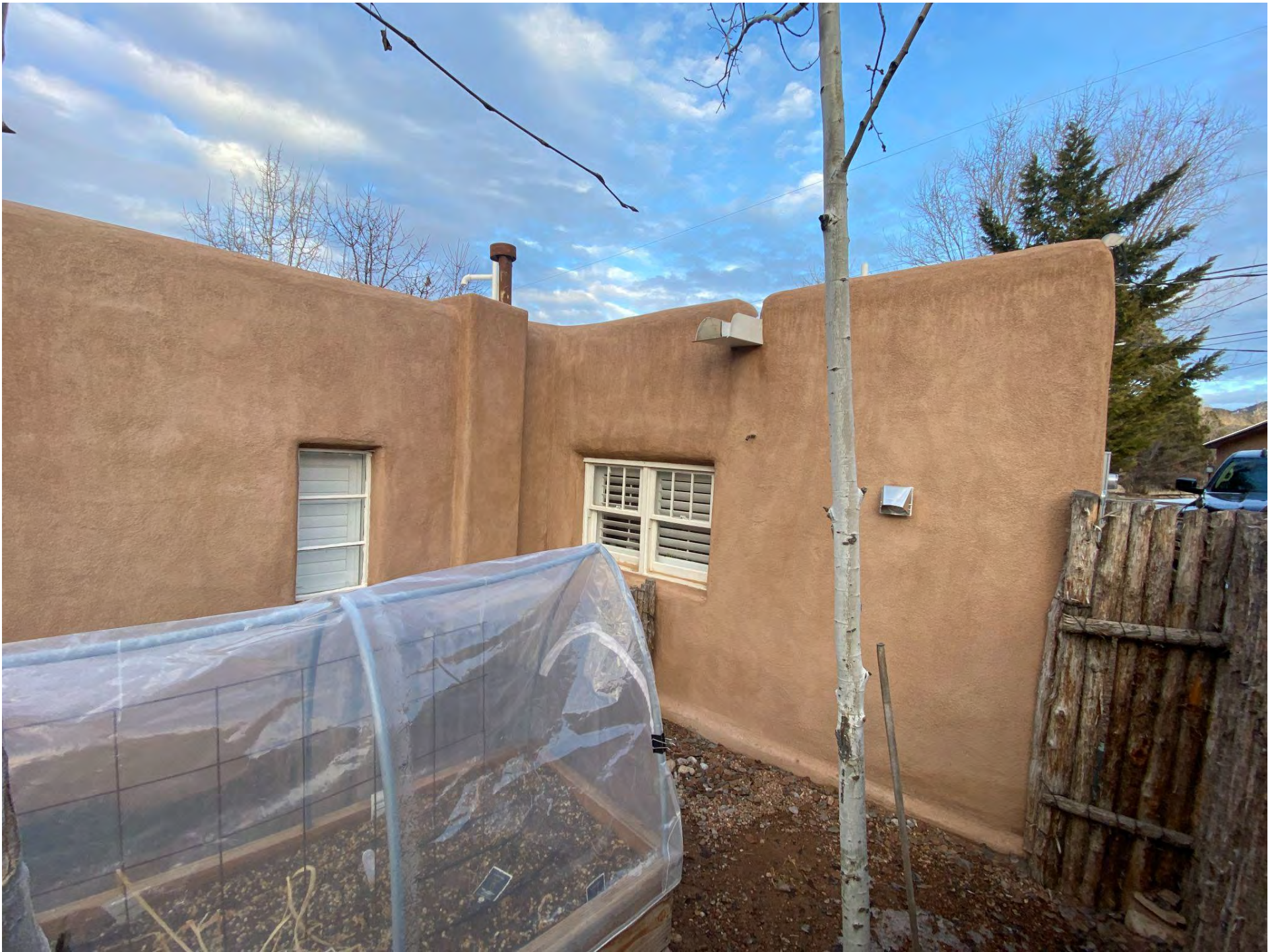
512 Abeyta Street Santa Fe, NM 87505- South West Elevation
