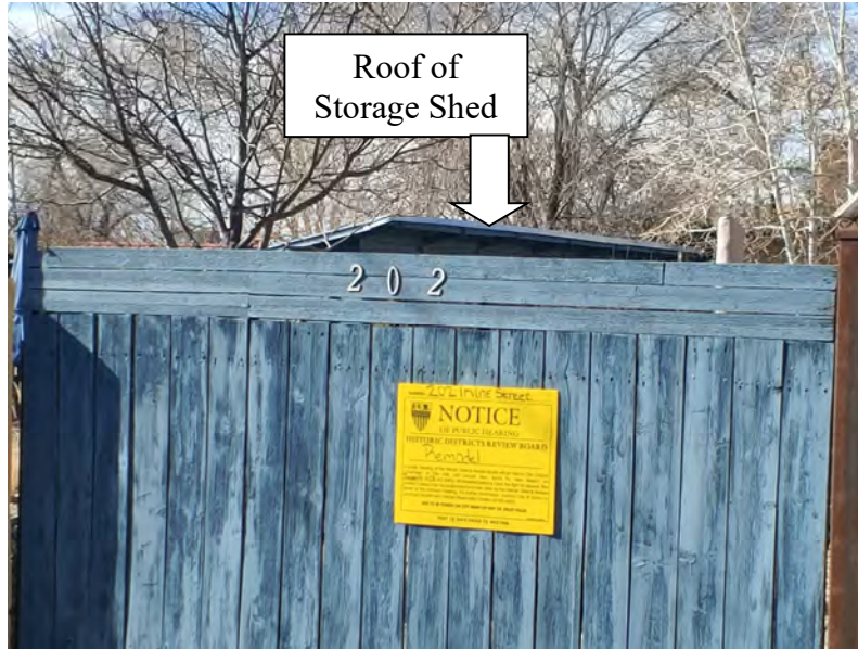
View of Storage Shed from Irvine Street (View looking West)
