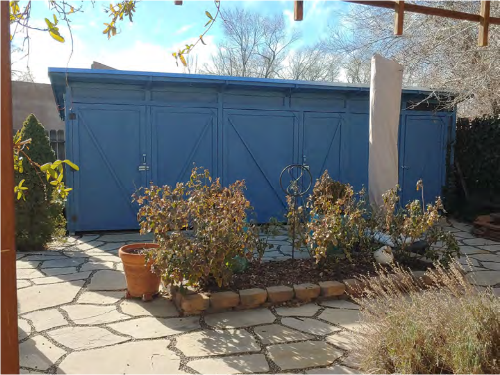
North Elevation (View looking South)
